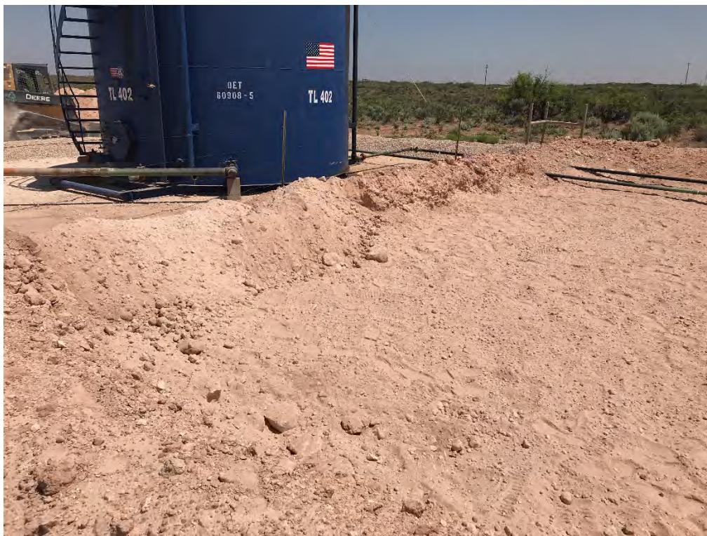
Backfilled Excavation (Looking Southeast)
