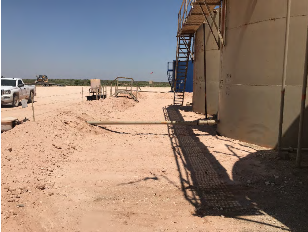
Backfilled Excavation (Looking East)
