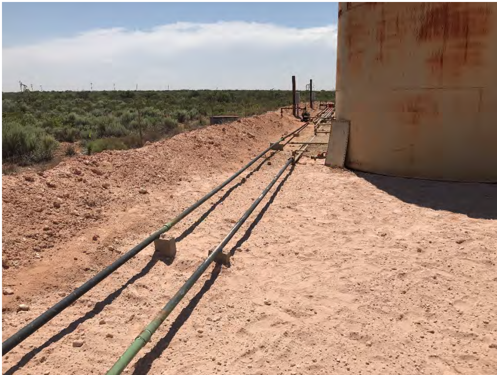
Backfilled Excavation (Looking West-Southwest)
