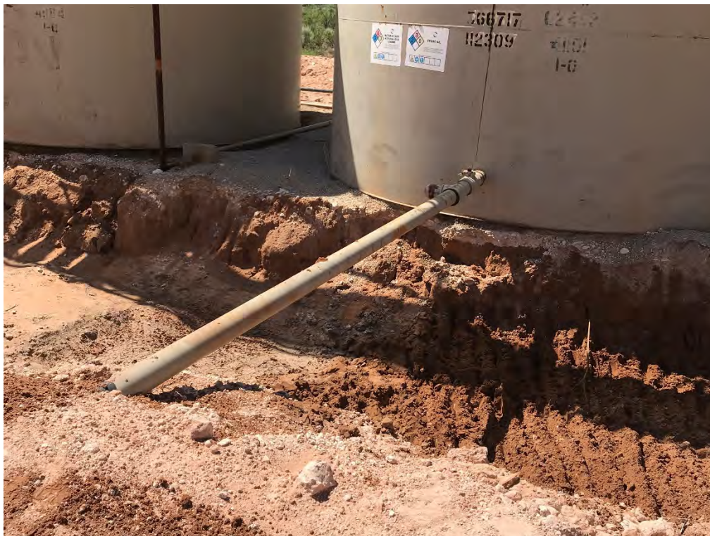
Excavation (Looking South-Southeast)
