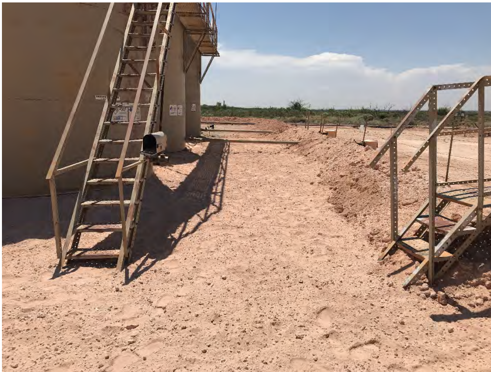
Backfilled Excavation (Looking West)
