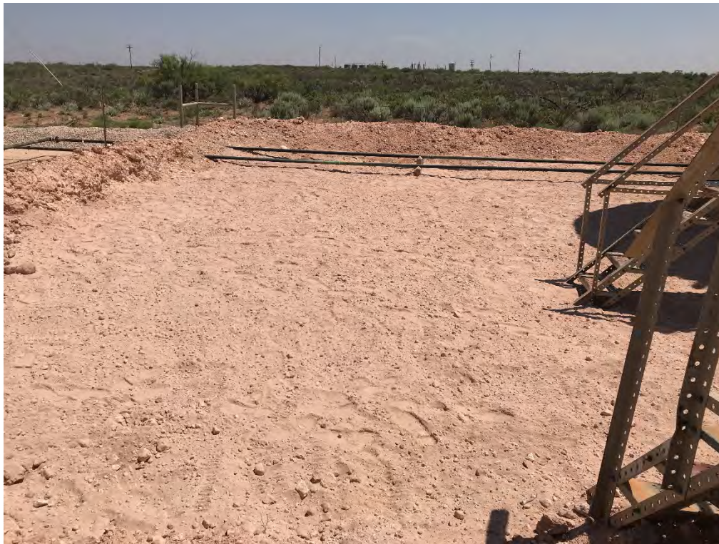
Backfilled Excavation (Looking South)
