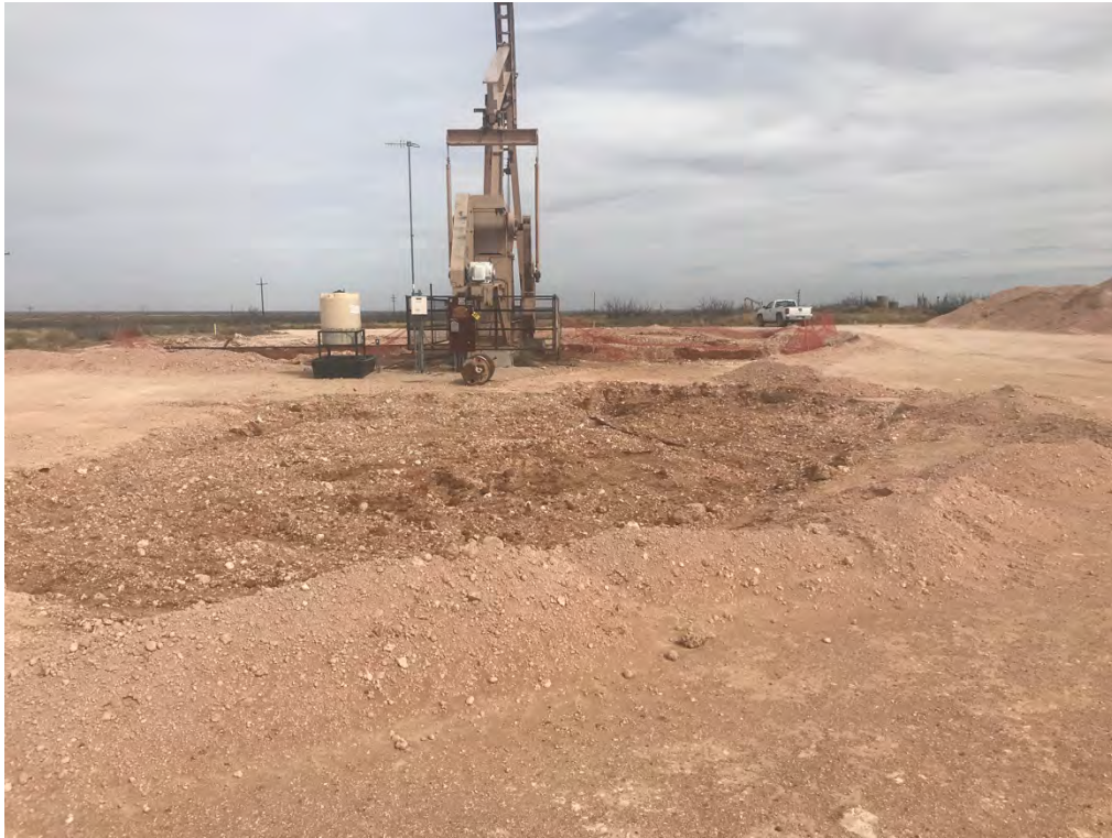
Covington A Federal 0002 – Excavation (Looking East)
