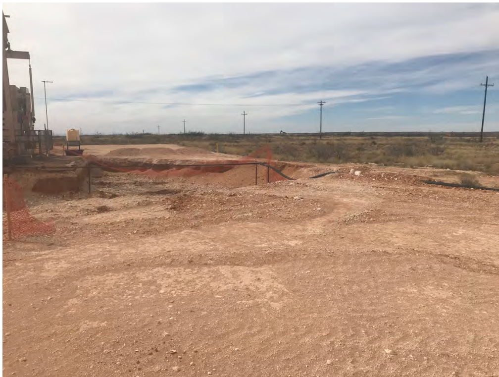
Covington A Federal 0002 – Excavation (Looking West)
