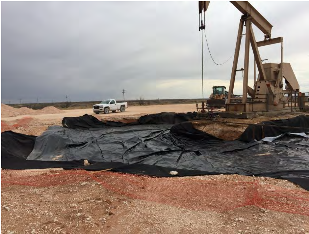
Covington A Federal 0002 – Felt & Liner Installation (Looking Southwest)
