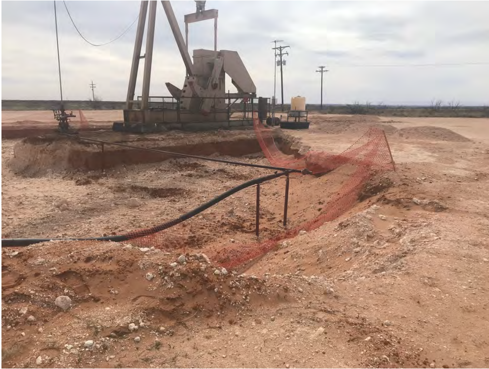
Covington A Federal 0002 – Excavation (Looking Southwest)
