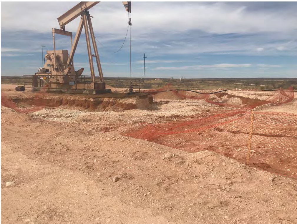
Covington A Federal 0002 – Excavation (Looking Northwest)
