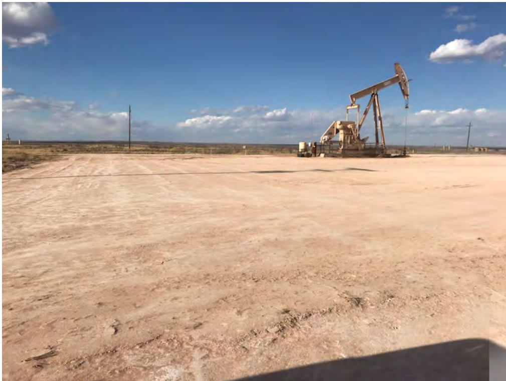
Covington A Federal 0002 – Backfilled Excavation (Looking North-Northeast)
