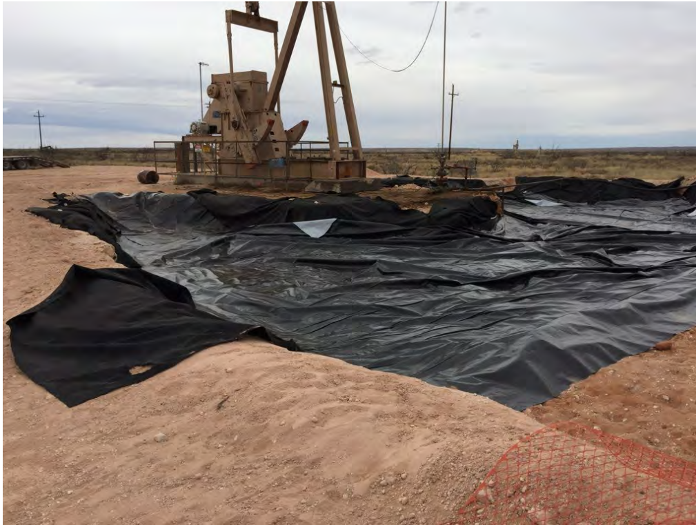
Covington A Federal 0002 – Felt & Liner Installation (Looking Northwest)
