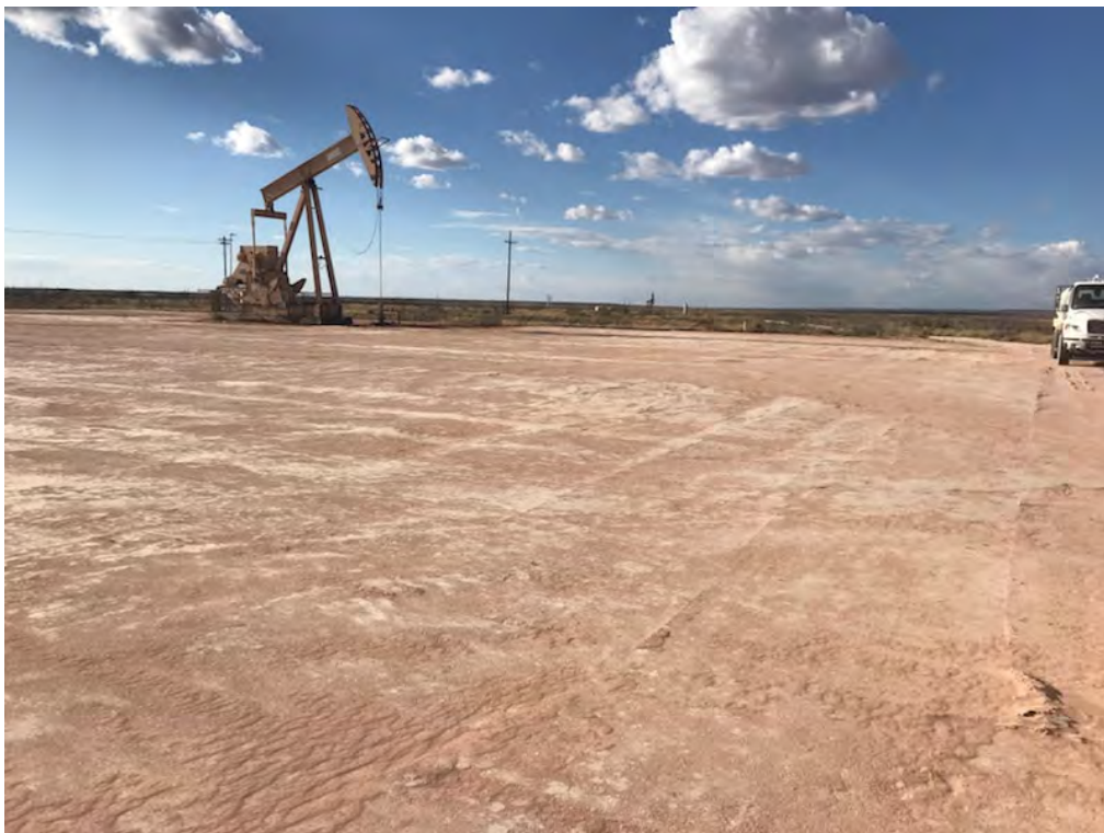
Covington A Federal 0002 – Backfilled Excavation (Looking North-Northwest)
