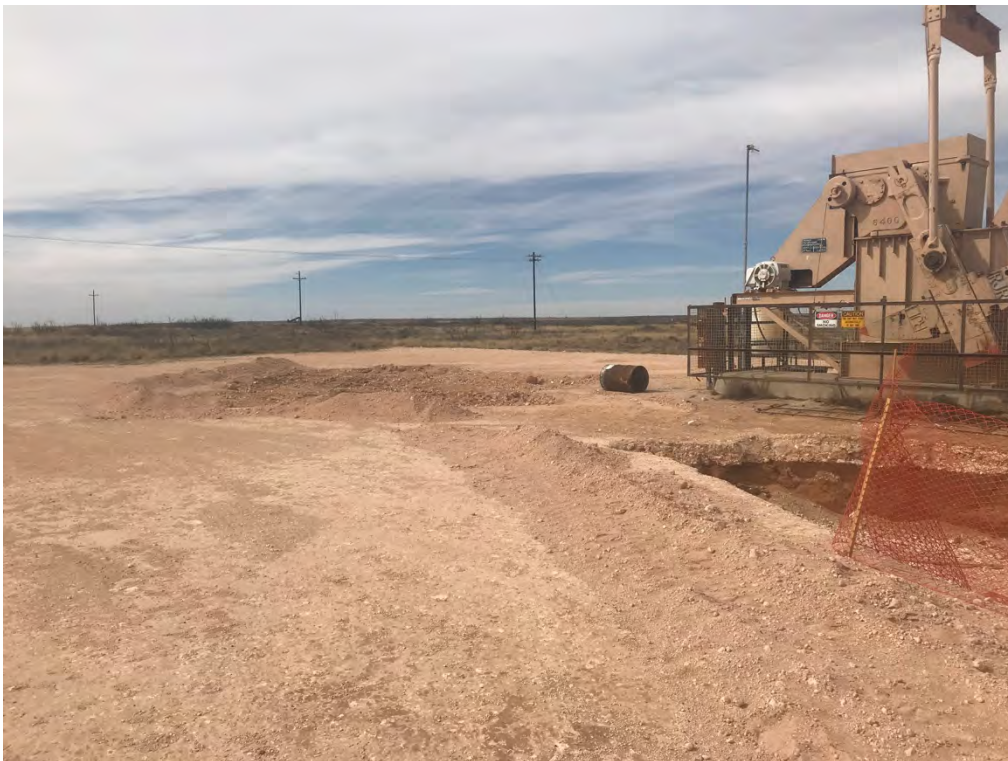
Covington A Federal 0002 – Excavation (Looking North-Northwest)
