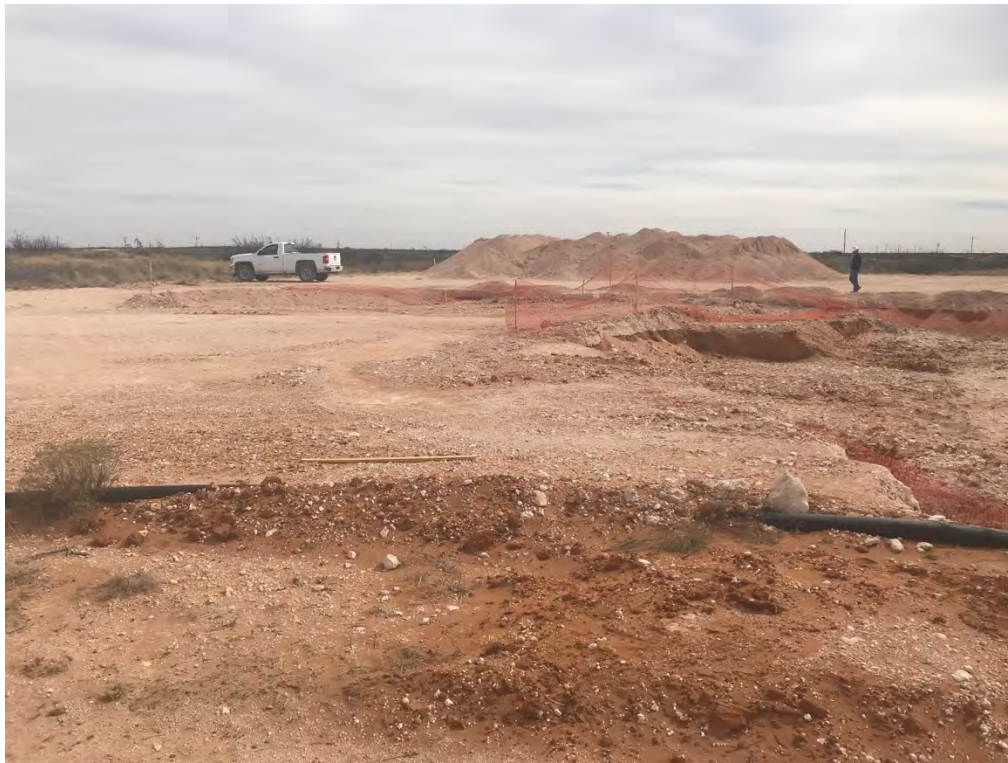
Covington A Federal 0002 – Excavation (Looking Southeast)
