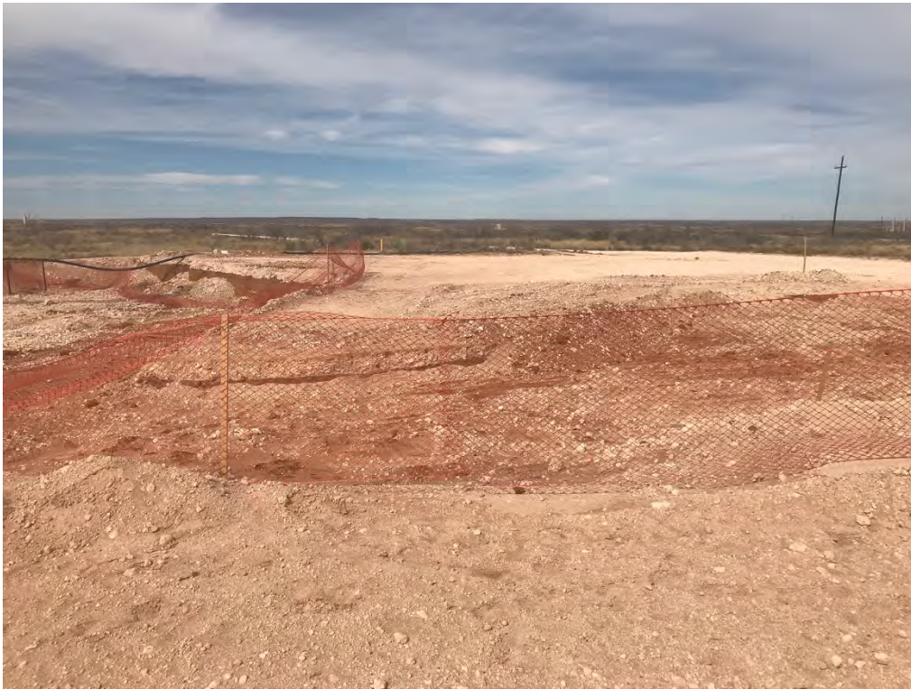
Covington A Federal 0002 – Excavation (Looking North)
