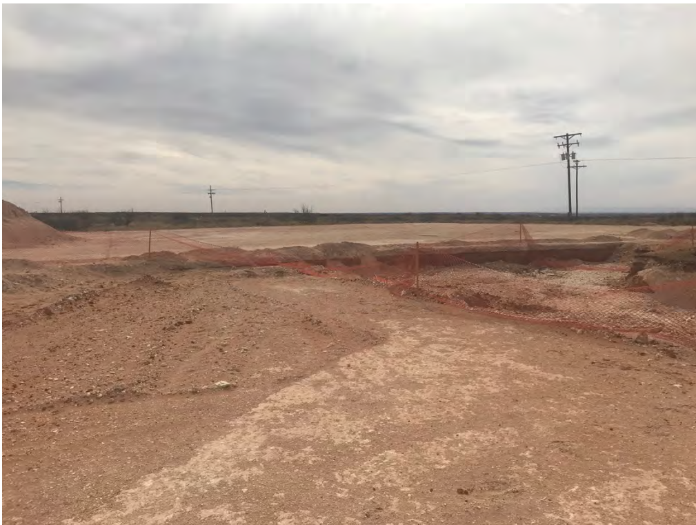
Covington A Federal 0002 – Excavation (Looking South-Southwest)
