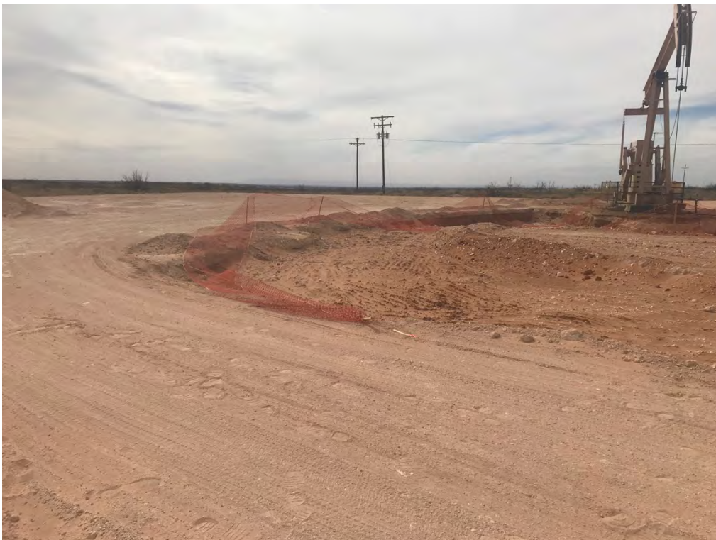
Covington A Federal 0002 – Excavation (Looking West)
