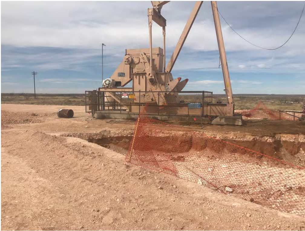
Covington A Federal 0002 – Excavation (Looking North)
