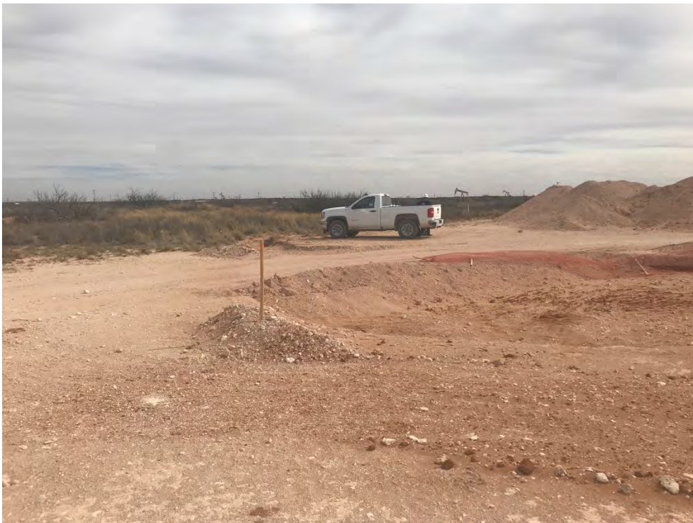
Covington A Federal 0002 – Excavation (Looking Southeast)
