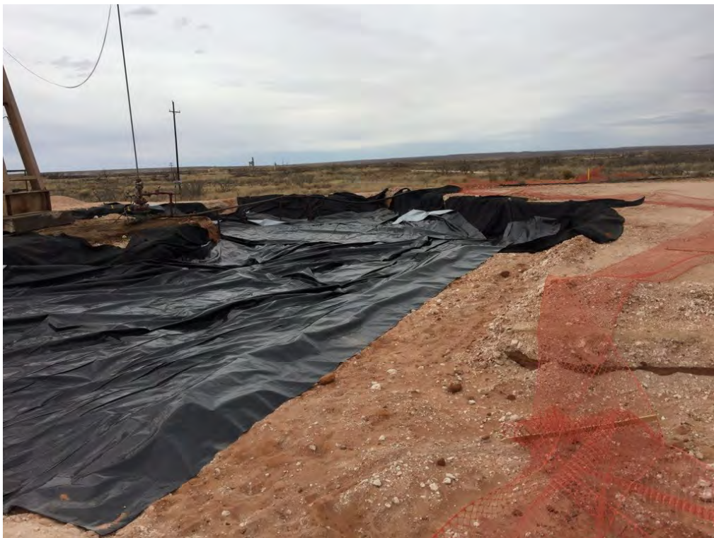
Covington A Federal 0002 – Felt & Liner Installation (Looking North-Northwest)
