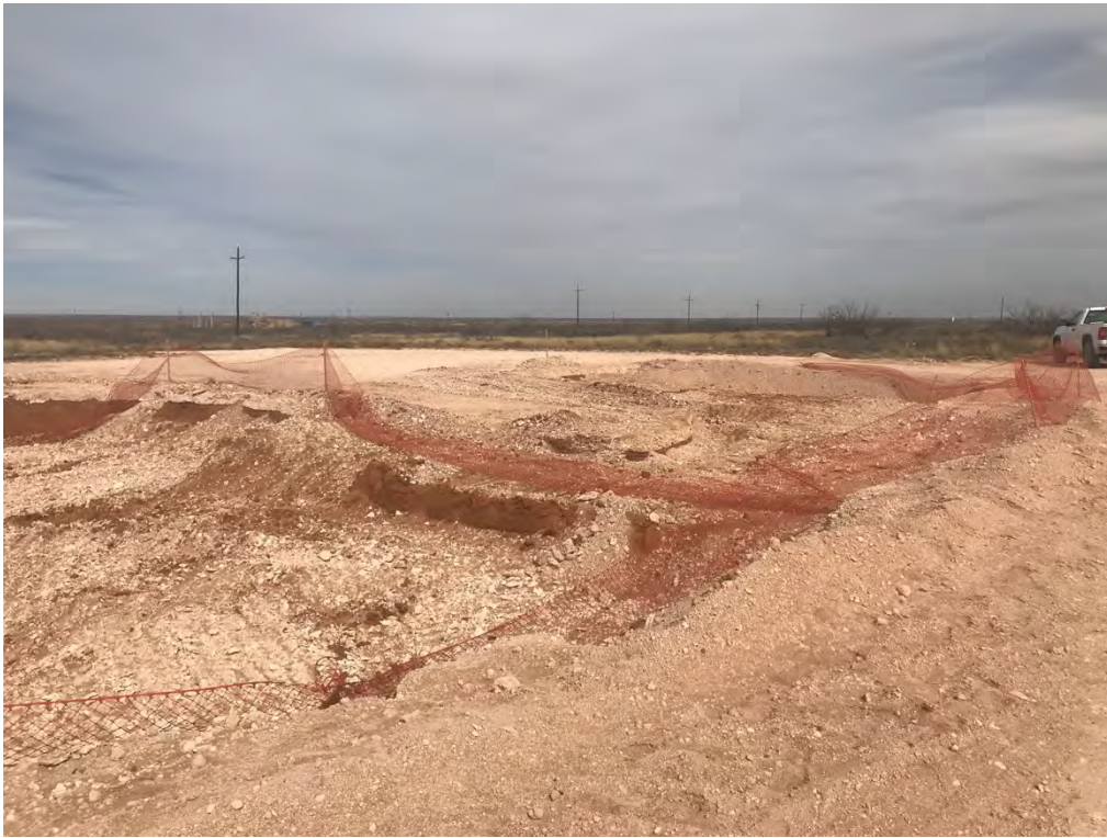
Covington A Federal 0002 – Excavation (Looking Northeast)
