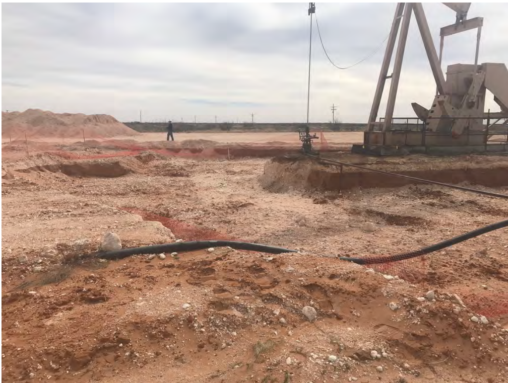
Covington A Federal 0002 – Excavation (Looking South-Southwest)
