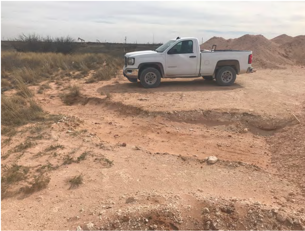
Covington A Federal 0002 – Excavation (Looking South)
