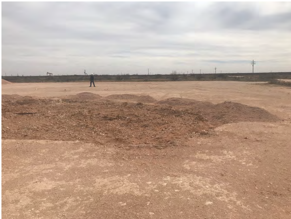
Covington A Federal 0002 – Excavation (Looking South)
