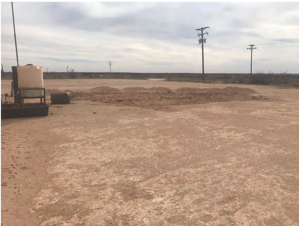
Covington A Federal 0002 – Excavation (Looking South-Southwest)
