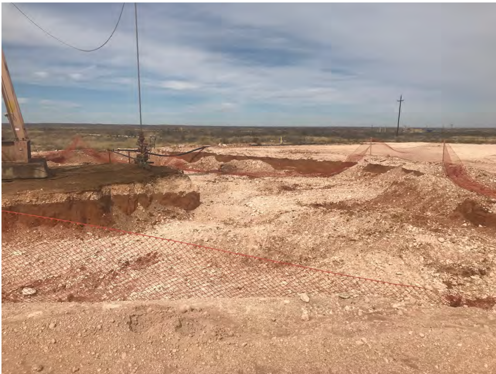
Covington A Federal 0002 – Excavation (Looking North-Northeast)
