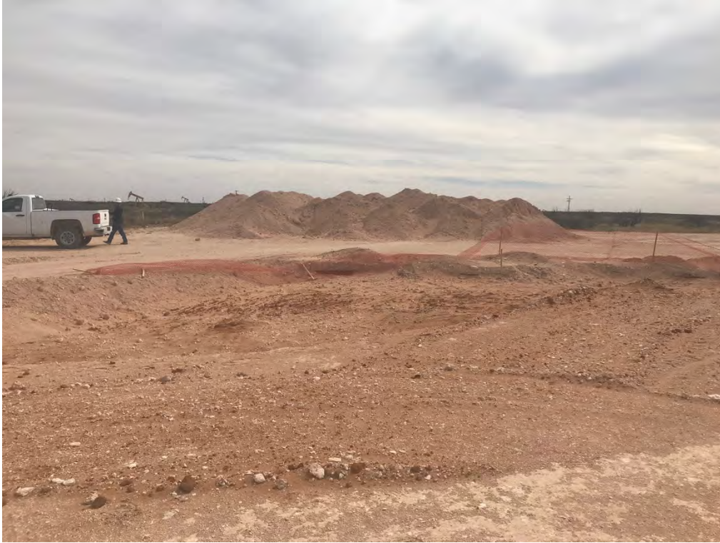
Covington A Federal 0002 – Excavation (Looking Southwest)
