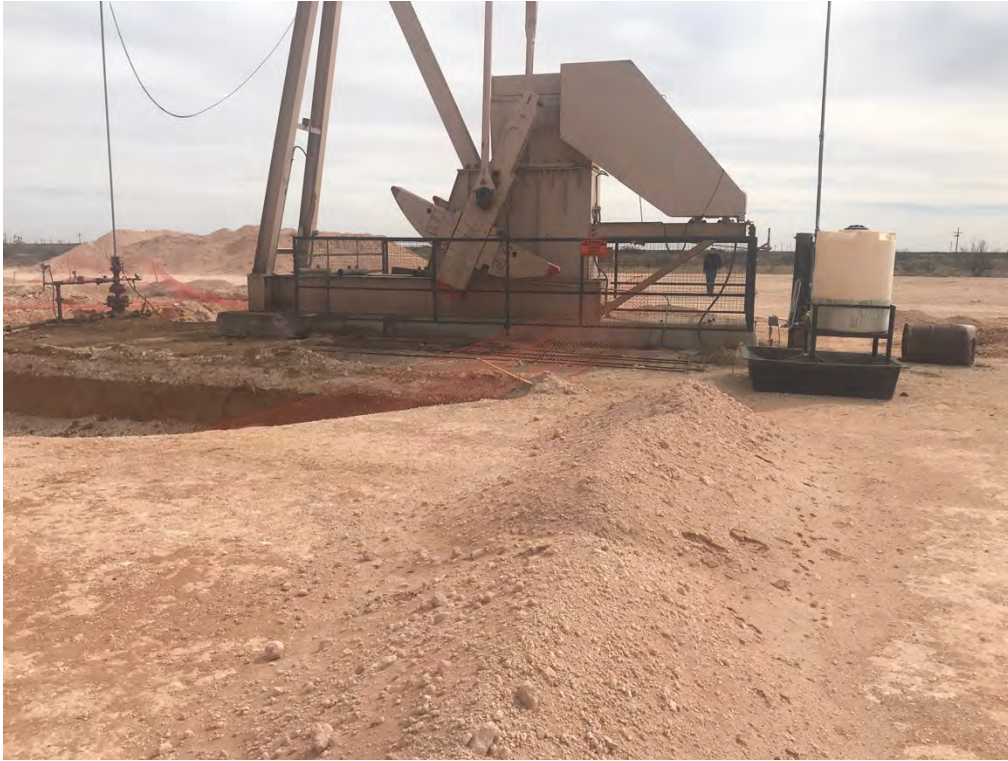
Covington A Federal 0002 – Excavation (Looking South-Southeast)
