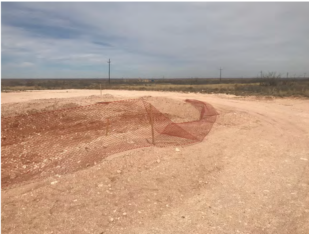
Covington A Federal 0002 – Excavation (Looking East-Northeast)
