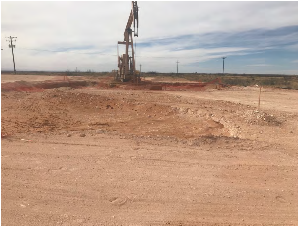
Covington A Federal 0002 – Excavation (Looking West-Northwest)
