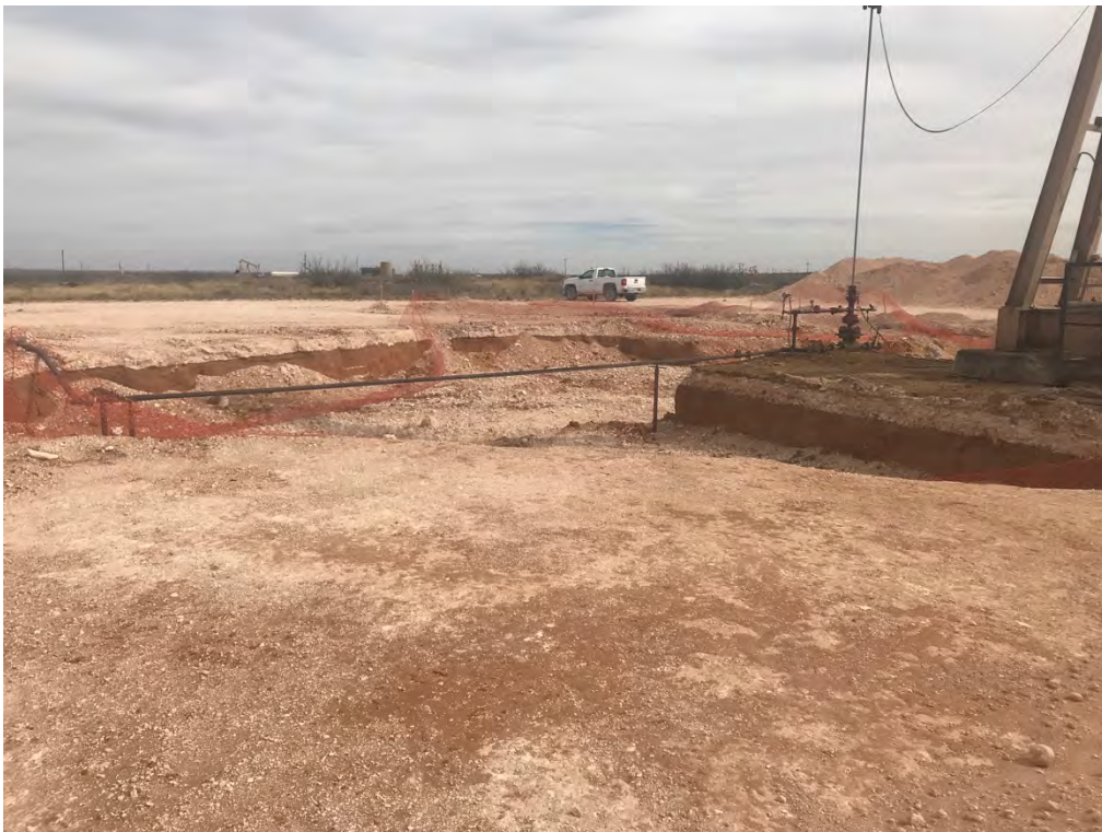
Covington A Federal 0002 – Excavation (Looking Southeast)
