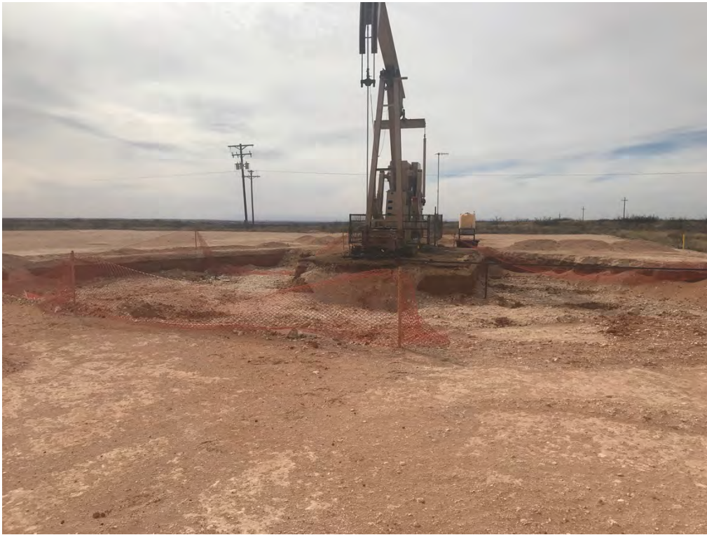
Covington A Federal 0002 – Excavation (Looking West)
