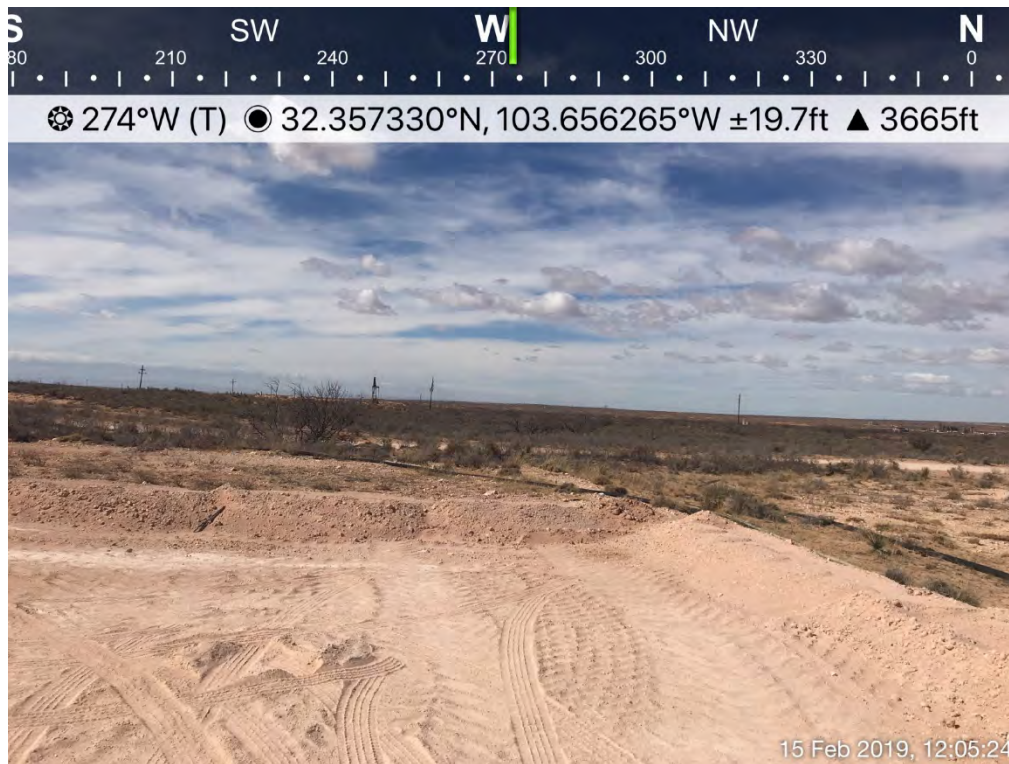
Backfilled Excavation (Looking West)
