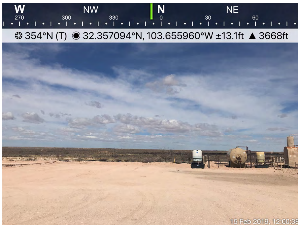
Backfilled Excavation (Looking North)
