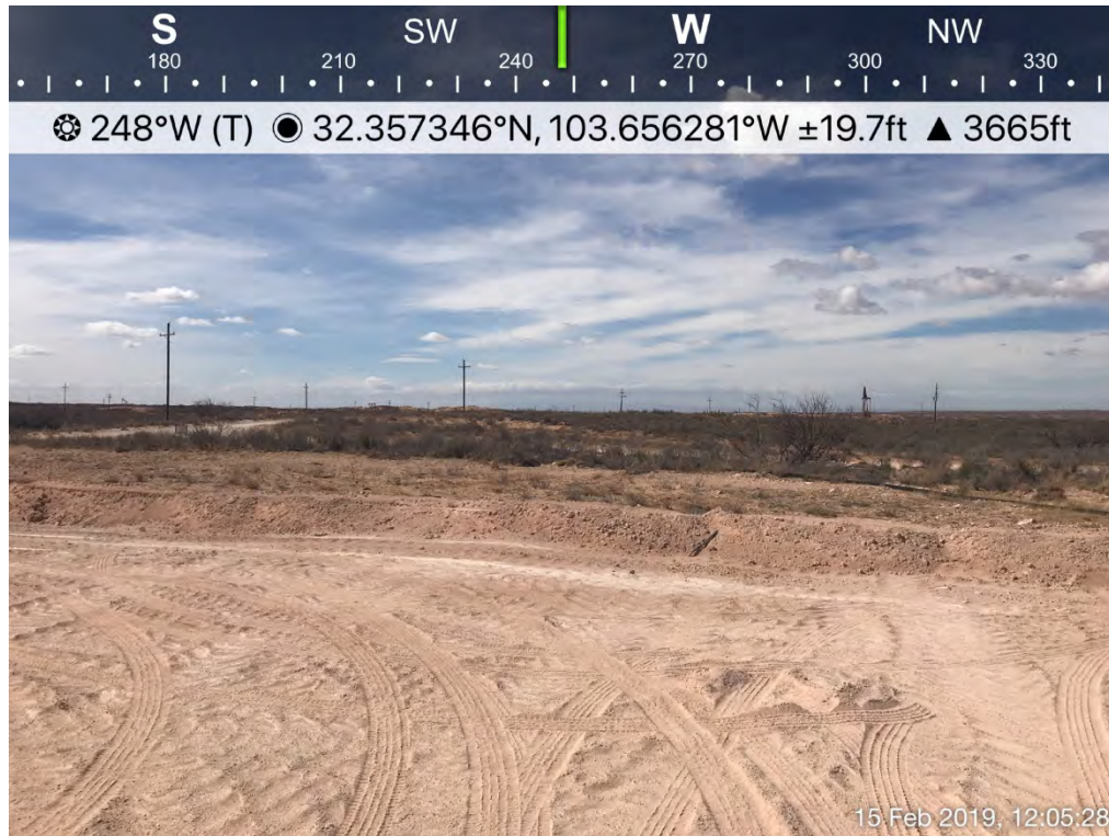
Backfilled Excavation (Looking West-Southwest)
