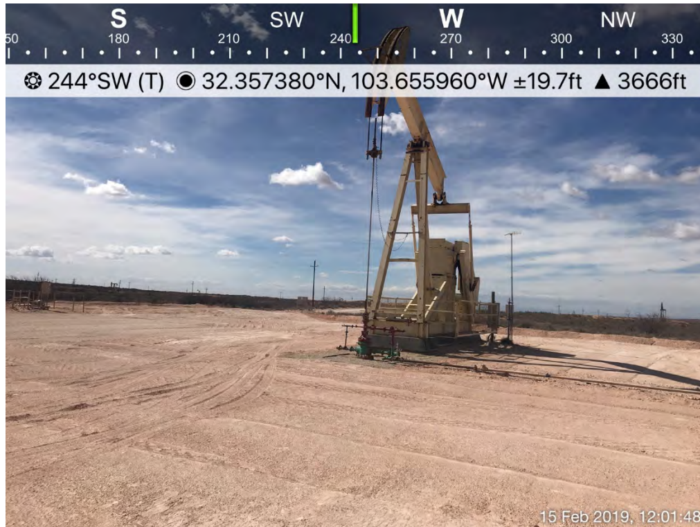
Backfilled Excavation (Looking West-Southwest)
