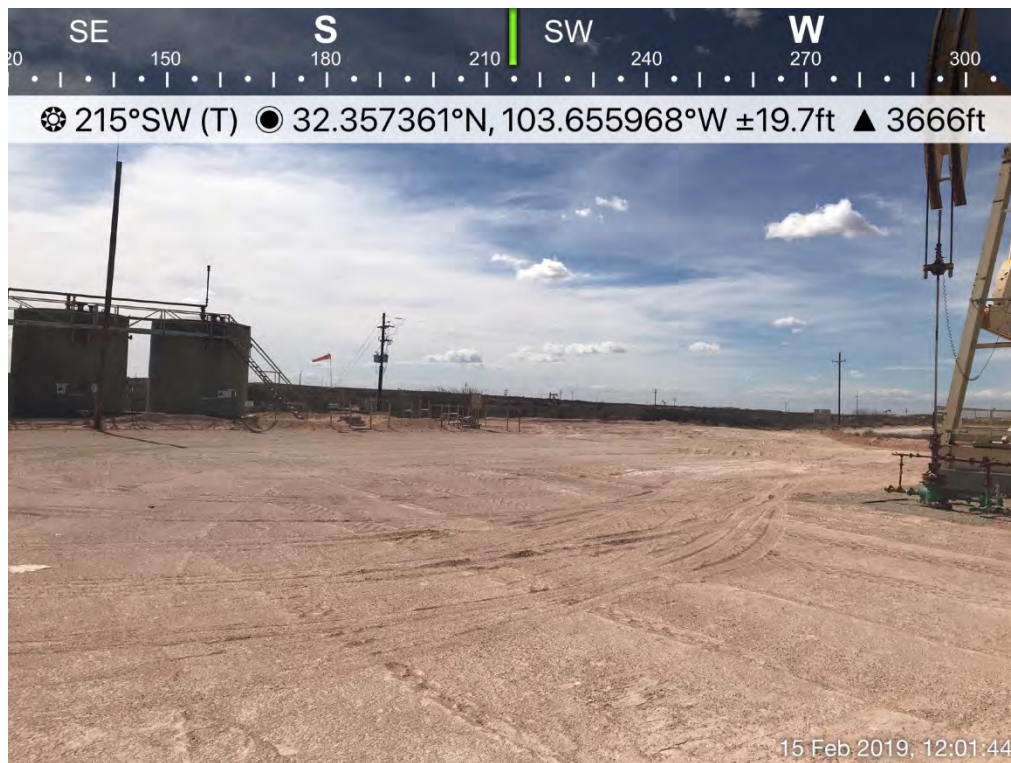
Backfilled Excavation (Looking Southwest)
