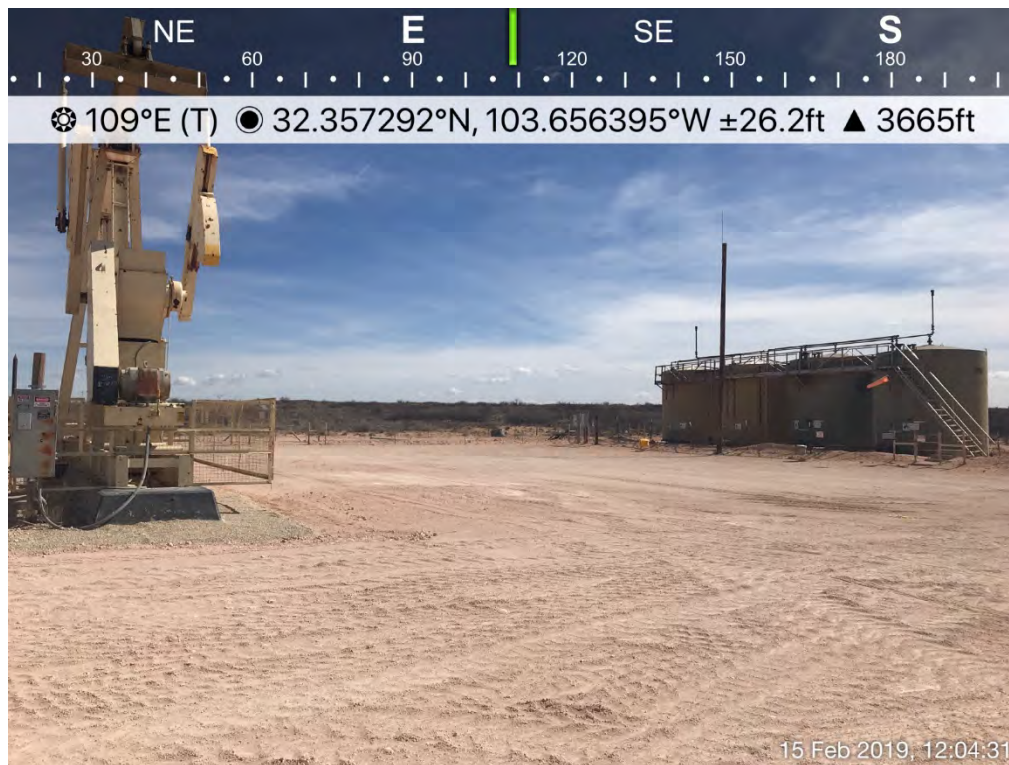
Backfilled Excavation (Looking East-Southeast)
