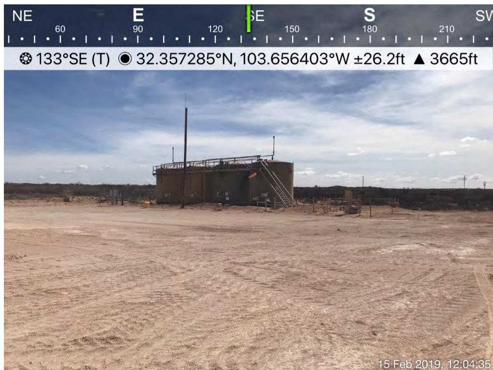
Backfilled Excavation (Looking Southeast)
