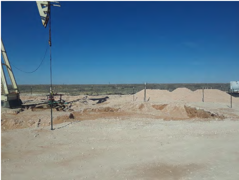
Excavation (Looking Northwest)
