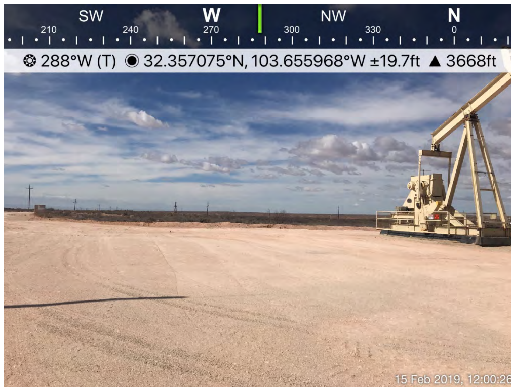
Backfilled Excavation (Looking West-Northwest)
