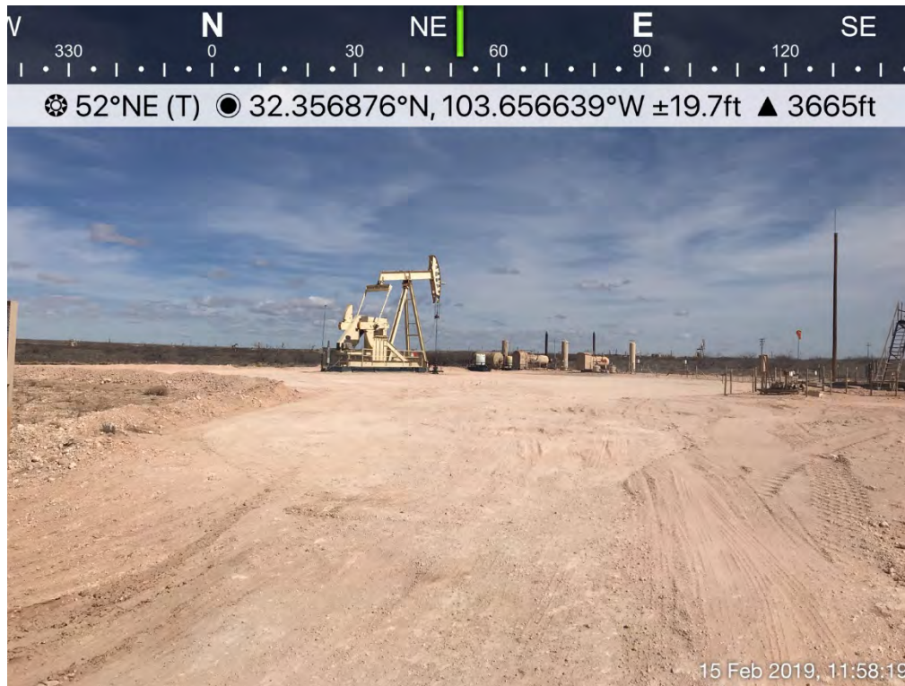
Backfilled Excavation (Looking Northeast)
