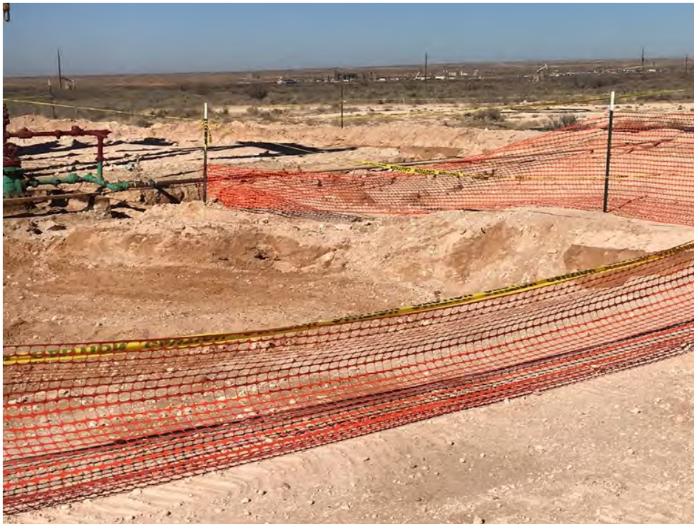
Backfilled Excavation (Looking Northwest)
