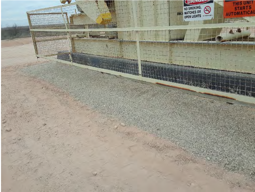
Backfilled Excavation (Looking West-Northwest)
