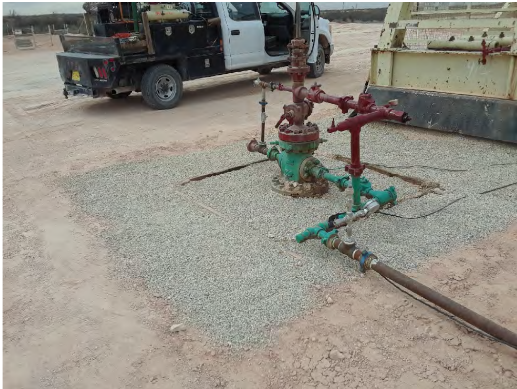
Backfilled Excavation (Looking South-Southwest)
