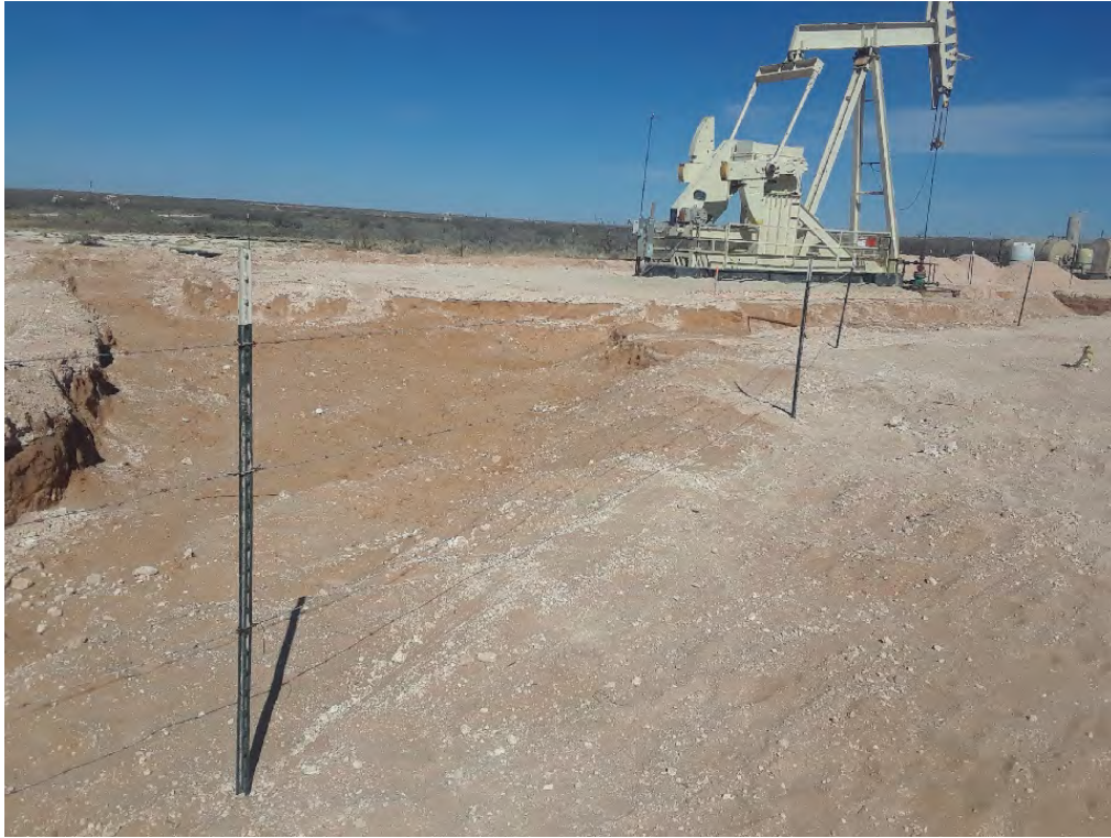
Excavation (Looking North-Northeast)
