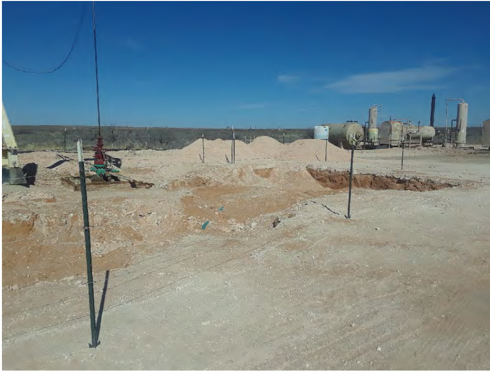
Excavation (Looking Northeast)
