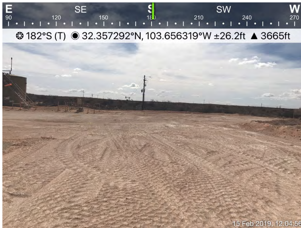
Backfilled Excavation (Looking South)
