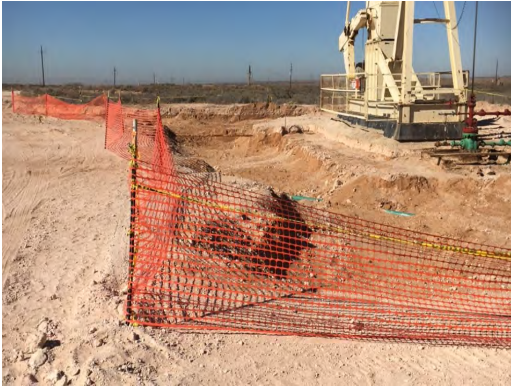
Excavation (Looking West-Northwest)
