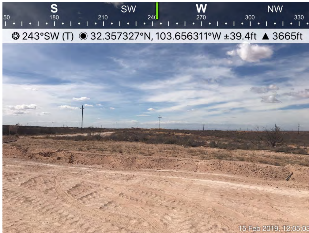
Backfilled Excavation (Looking West-Southwest)
