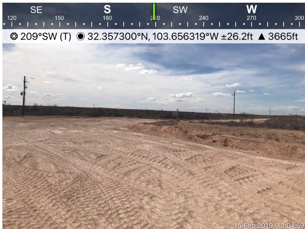
Backfilled Excavation (Looking South-Southwest)
