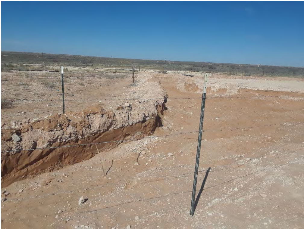
Excavation (Looking North)
