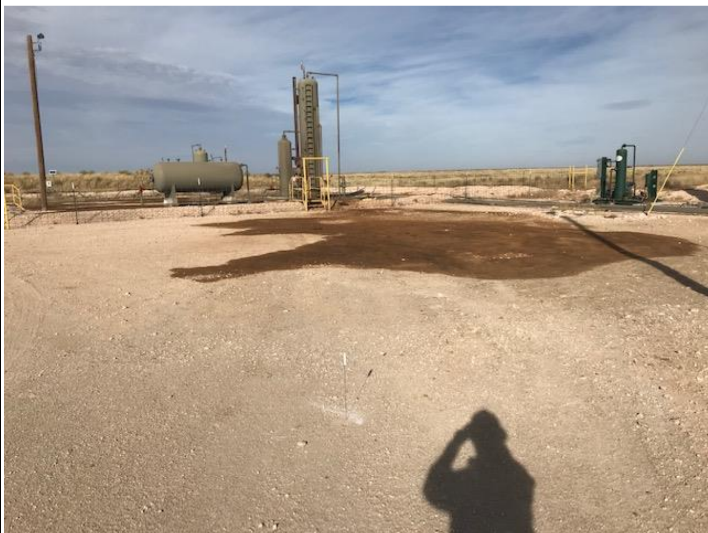
View of release extent on the caliche well pad, facing northeast.
