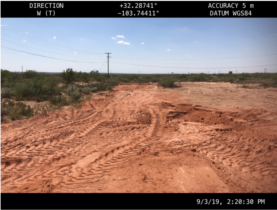
Back Filled Excavation
