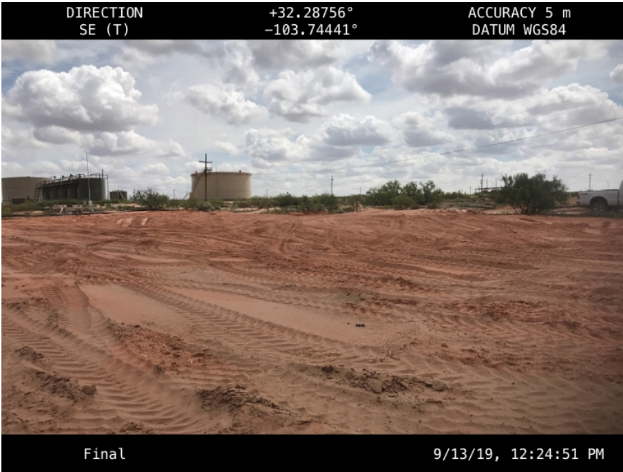
Back Filled Excavation
