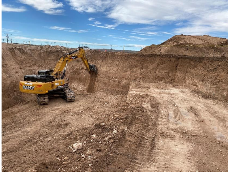
Photograph 13: View of the excavation facing northeast.
