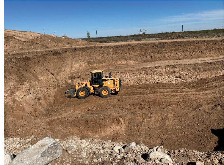
Photograph 14: View of the excavation facing east.
