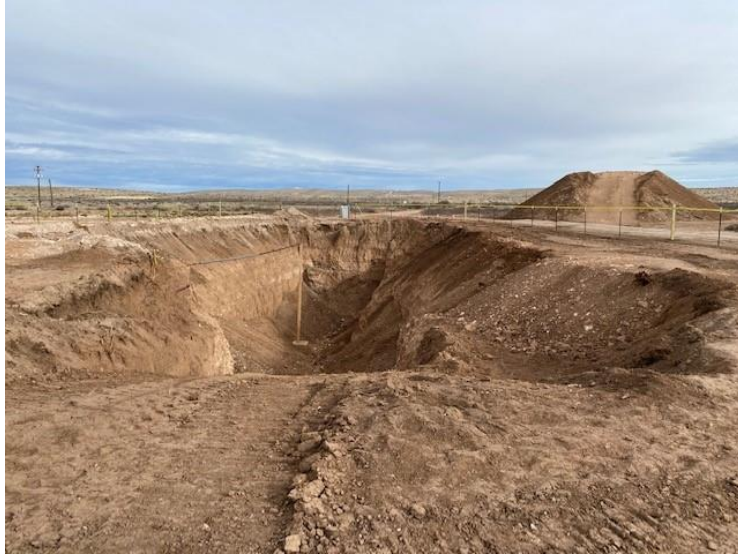
Photograph 5: View of the excavation facing north.
