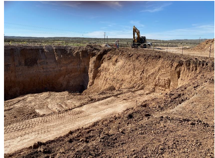
Photograph 16: View of the excavation facing northwest.
