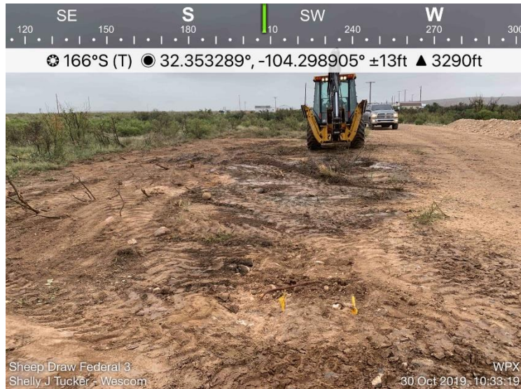
Photograph 1: View of the Site facing south. Photo by courtesy of Wescom.
