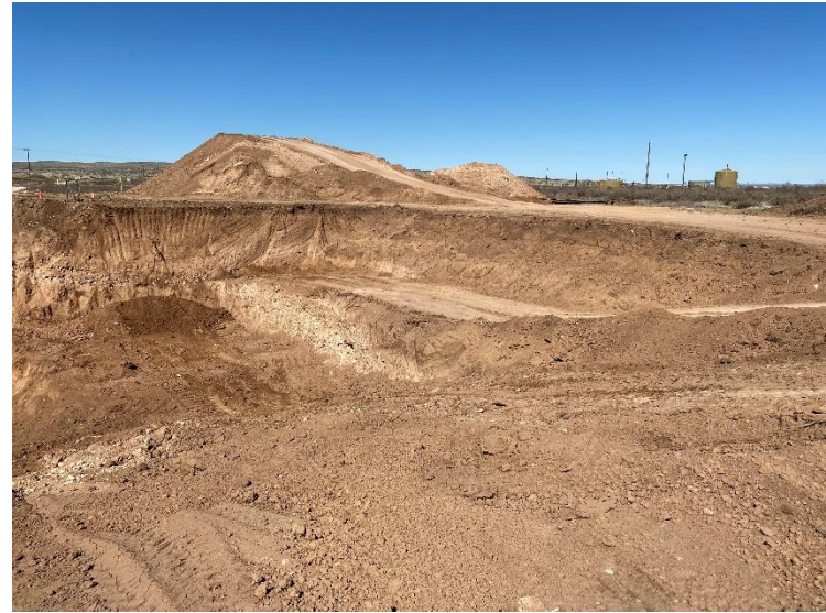
Photograph 10: View of the excavation facing east.
