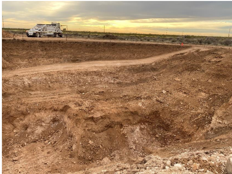
Photograph 15: View of the excavation facing southeast.
