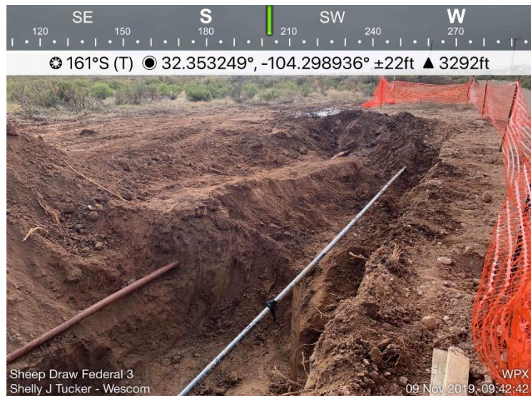
Photograph 3: View of the Site facing south. Photo by courtesy of Wescom.
