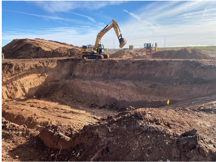
Photograph 9: View of the excavation facing east.
