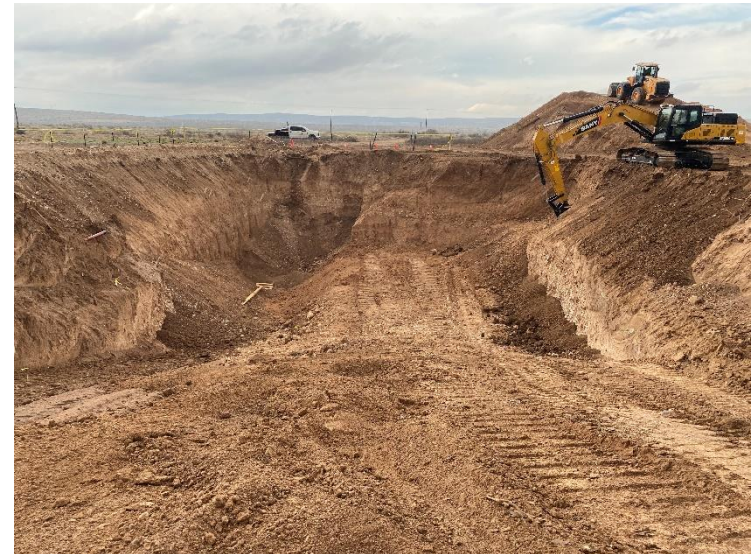
Photograph 8: View of the excavation facing north.
