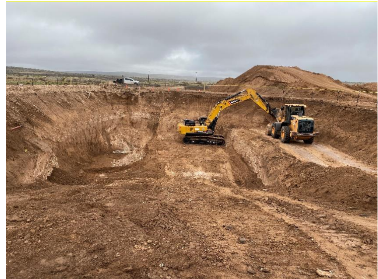
Photograph 12: View of the excavation facing north.
