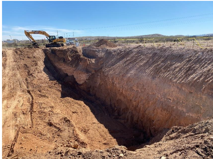
Photograph 11: View of the excavation facing southwest.
