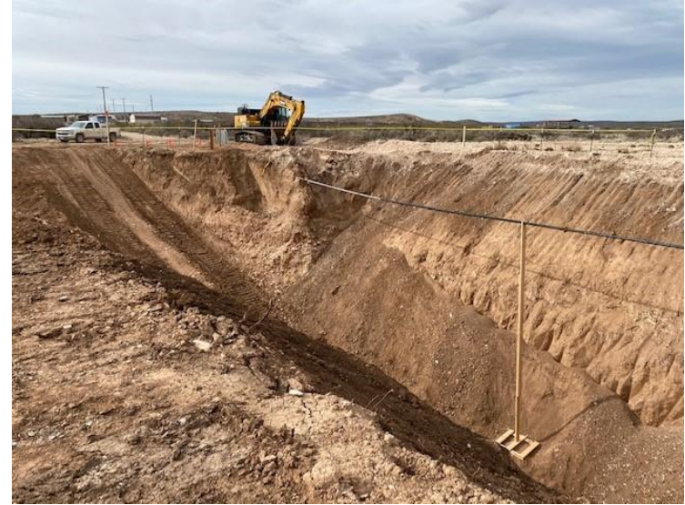
Photograph 6: View of the excavation facing southwest.
