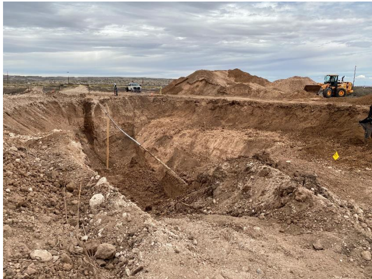
Photograph 7: View of the excavation facing northeast.
