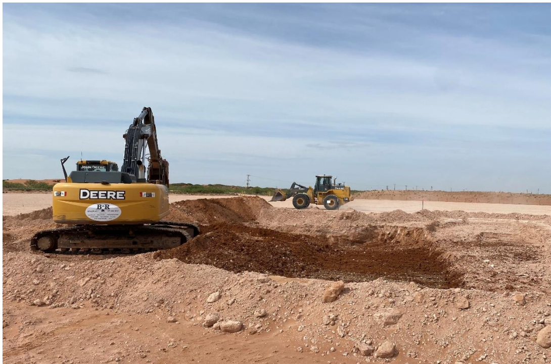
Southwestern view of excavation during excavation activities.
