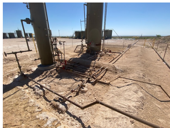
Photograph 4: View of hydrovac excavation around equipment facing southwest.
