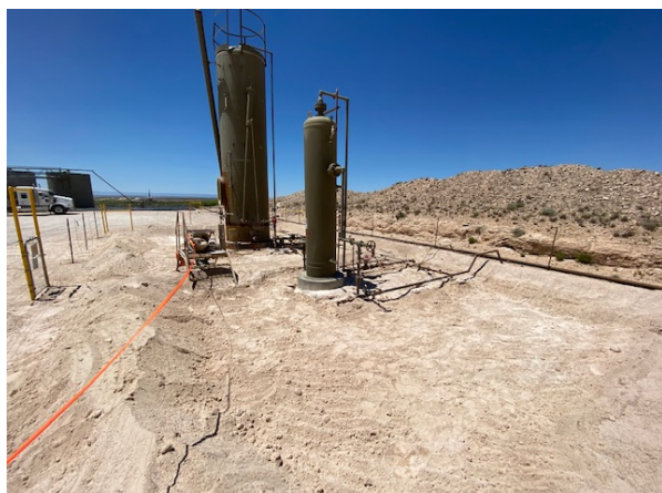
Photograph 5: View of excavation around equipment facing northwest.
