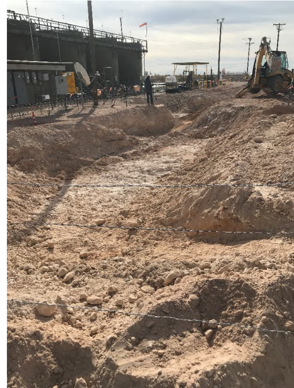
Photograph 4: South facing view of excavation.
