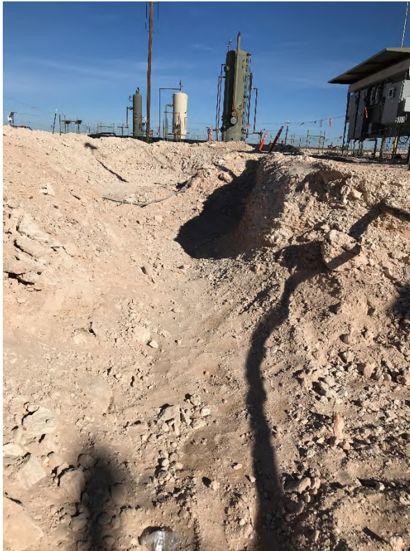
Photograph 3: North facing view of excavation.
