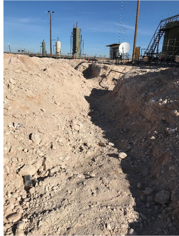
Photograph 2: North facing view of excavation.
