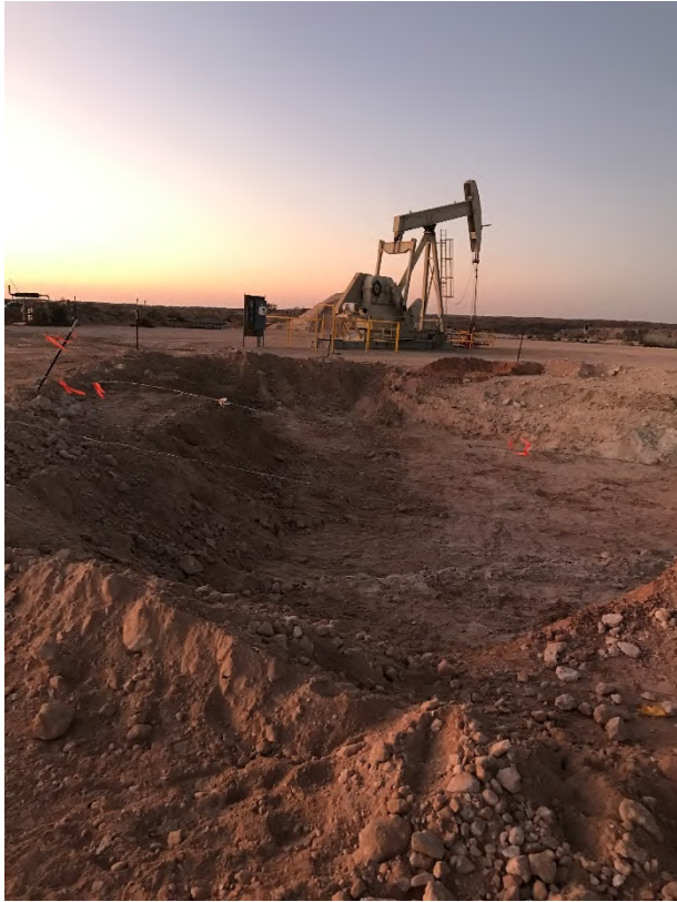
Photograph 1: Northwest facing view of excavation.
