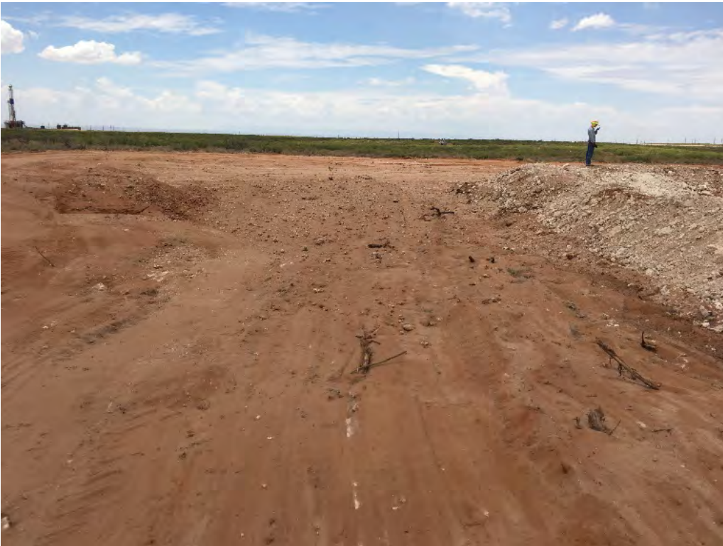
Photograph 10: Western view of completed backfill off-pad.
