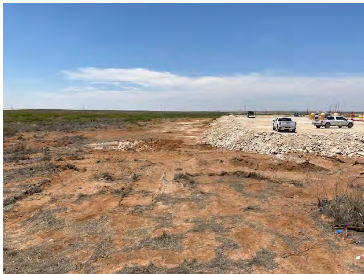
Photograph 5: Northwest view of SS12 and SS13.
