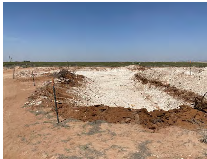
Photograph 6: Western view of excavation off-pad.
