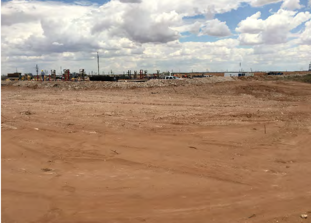
Photograph 9: Southeastern view of completed backfill off-pad.
