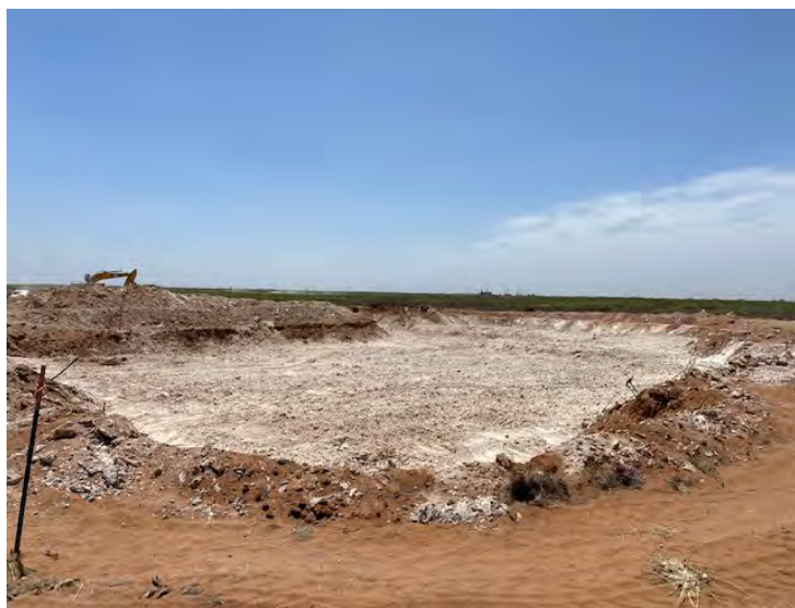
Photograph 7: Southeastern view of excavation off-pad.
