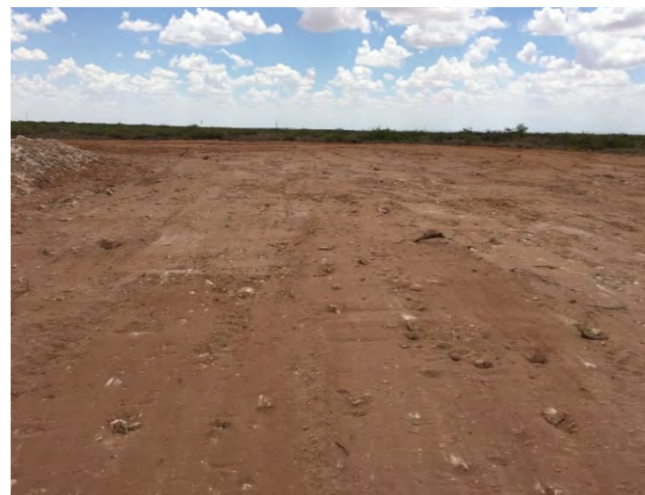
Photograph 8: Backfilled excavation northern view.
