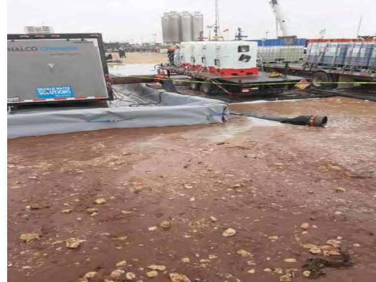
Photograph 2: Northwestern view of disconnected lay flat line and equipment.
