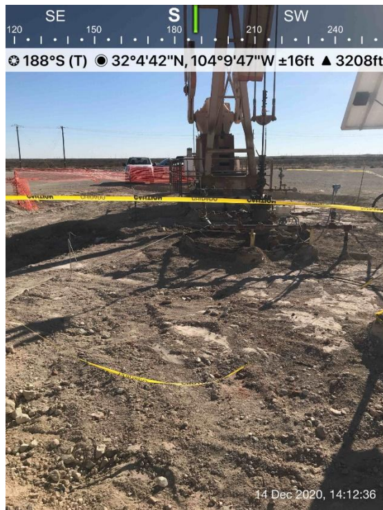
Excavated soil viewing south, December 14, 2020
