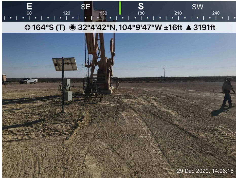
Backfilled excavation viewing south, December 29, 2020
