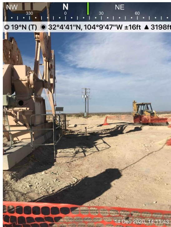
Excavated soil viewing north/northeast, December 14, 2020
