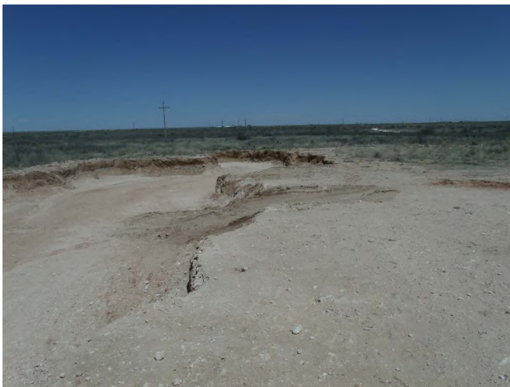
Photograph #3 – Looking northerly across excavation
