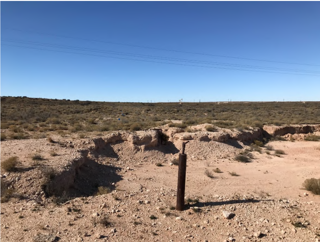
Photograph 2: View of excavation and drilling area facing west.
