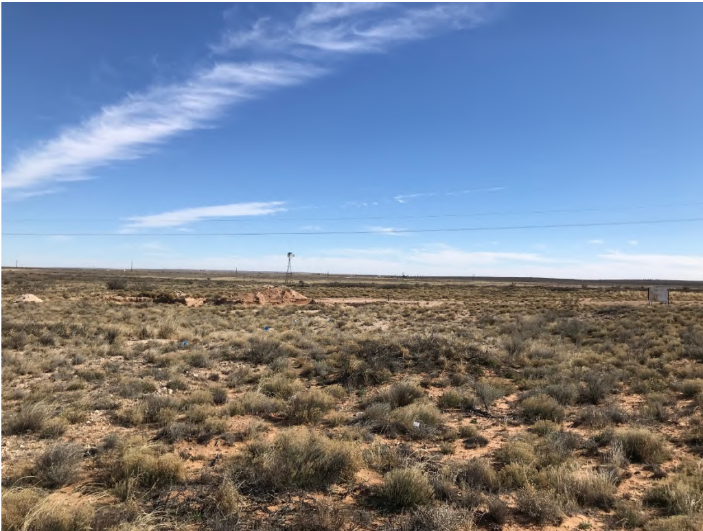
Photograph 4: View west of excavation facing east.
