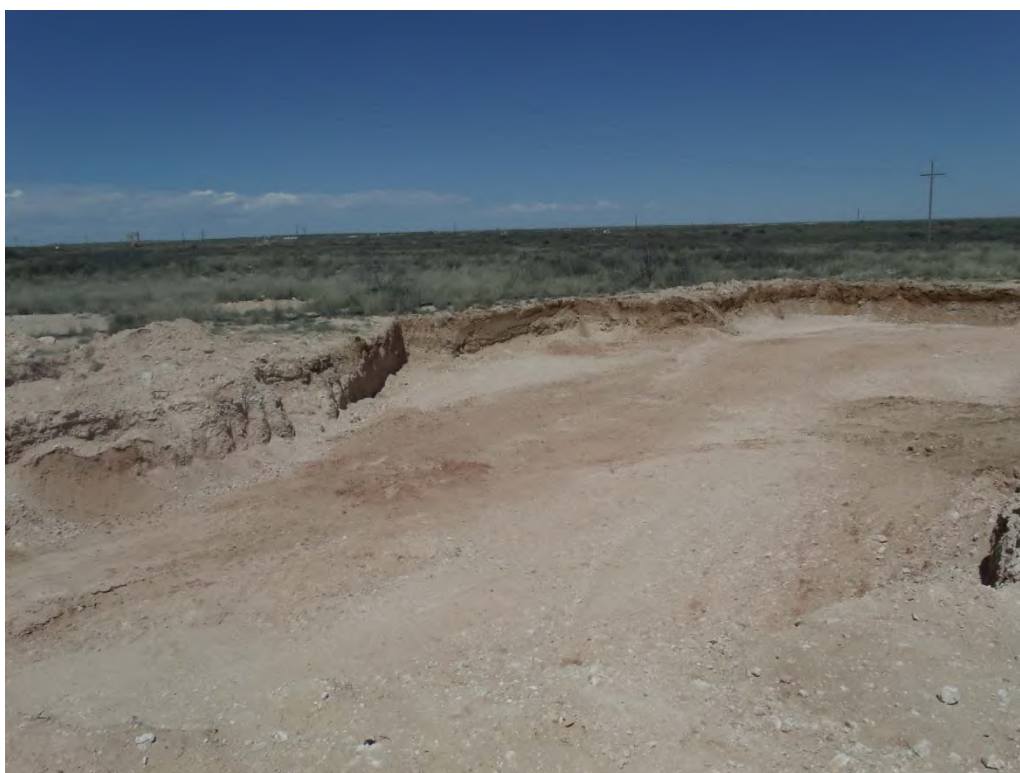
Photograph #2 – Looking north-westerly across excavation
