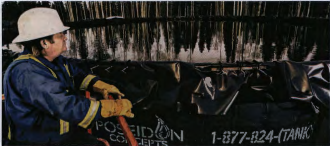
Photo 6: Clamping system holding liner in place. Spacing between clamping is 3-feet.
