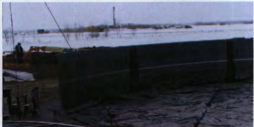
Photo 5: Interlocking panels of the modular impoundment.
