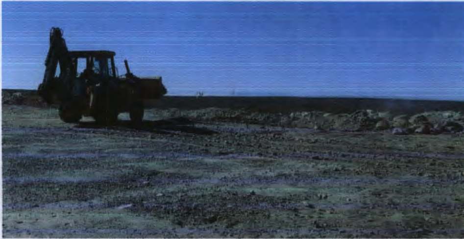
Figure 3: Re-using material from former containment berms from the CleanWave system to reinforce existing containment berms.
