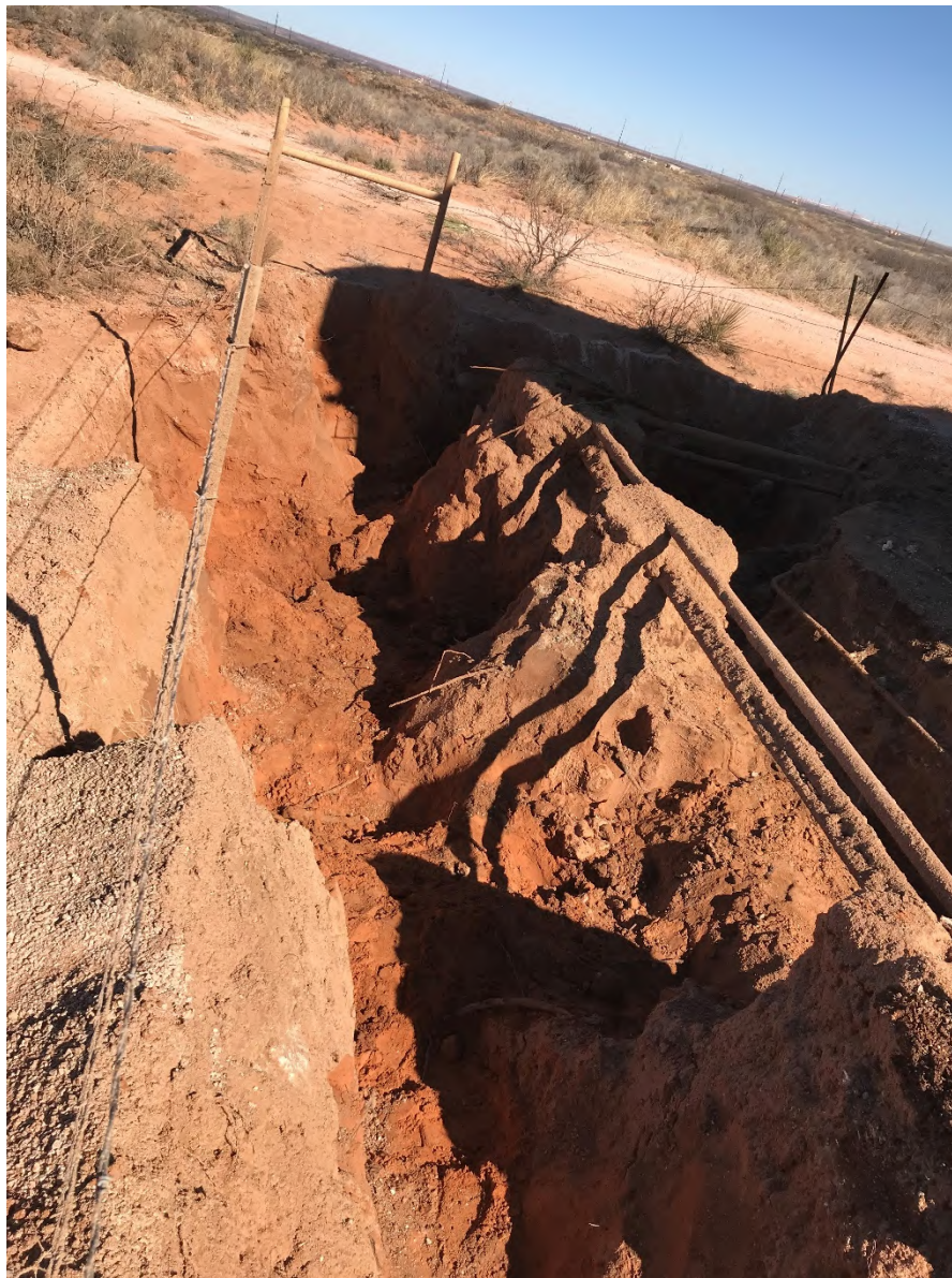
View facing west of initial excavation activities.
