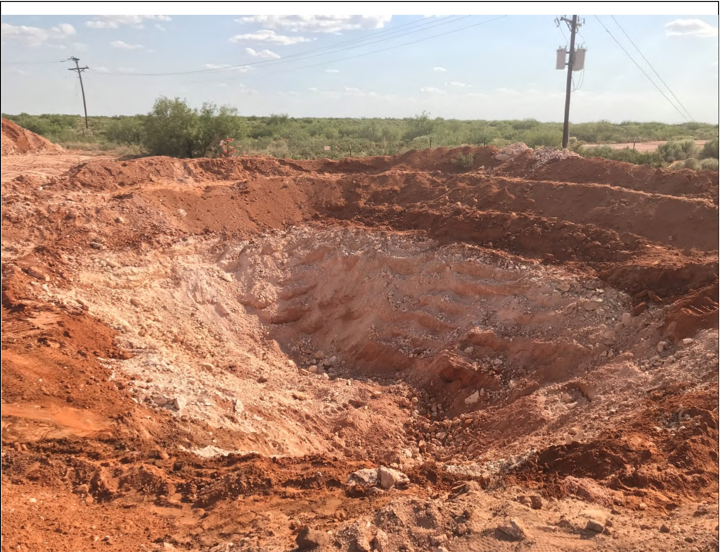
View facing southwest of the open excavation.
