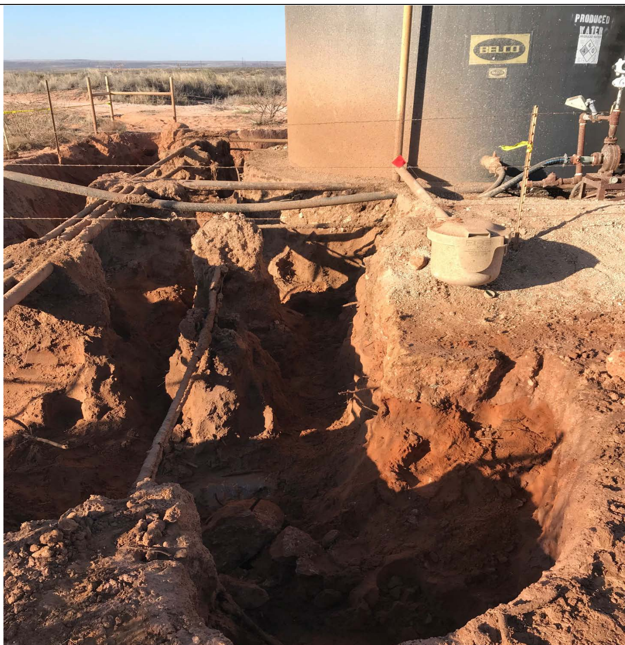
View facing north of initial excavation activities.
