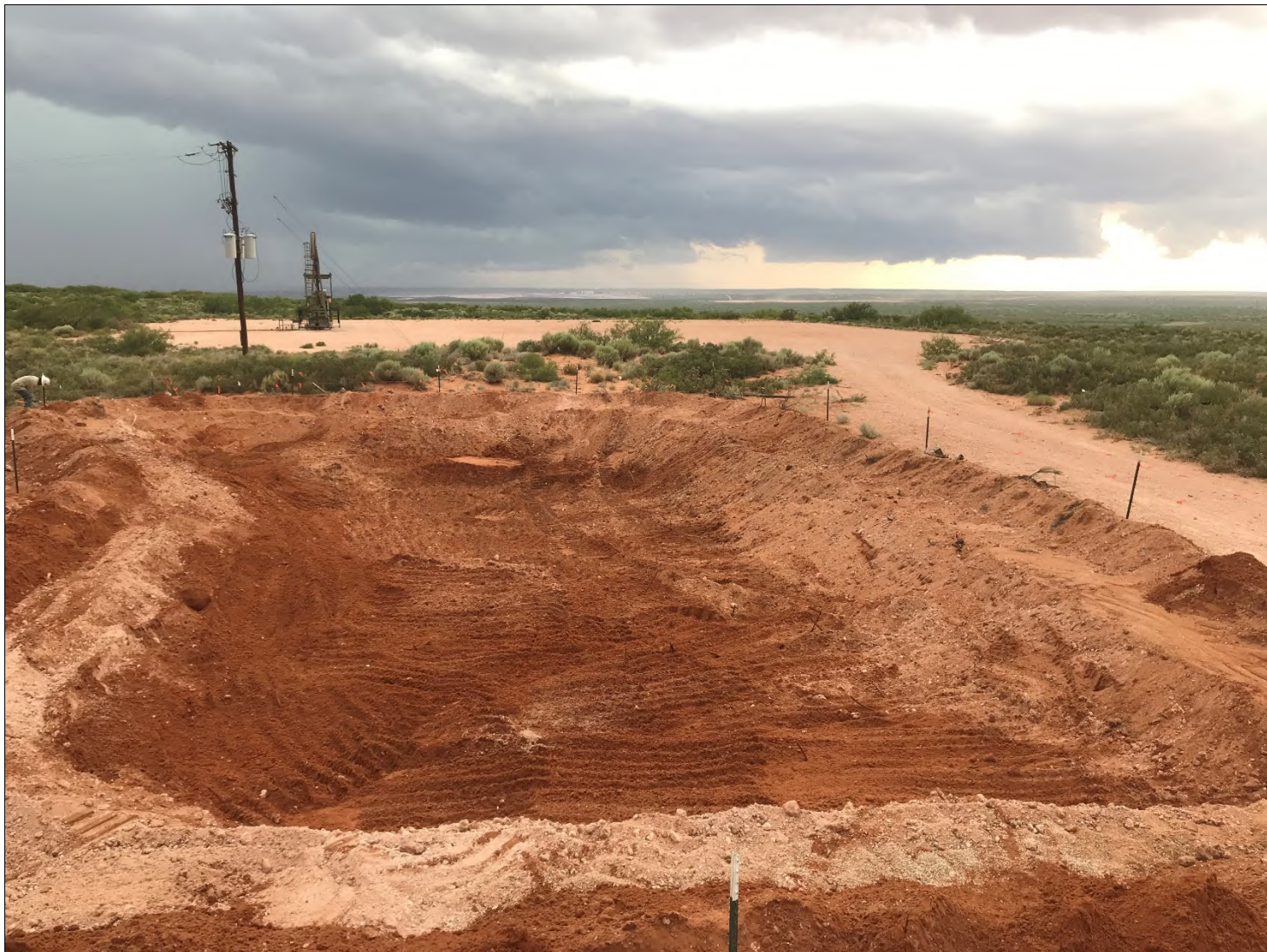
View facing west post tank battery removal.
