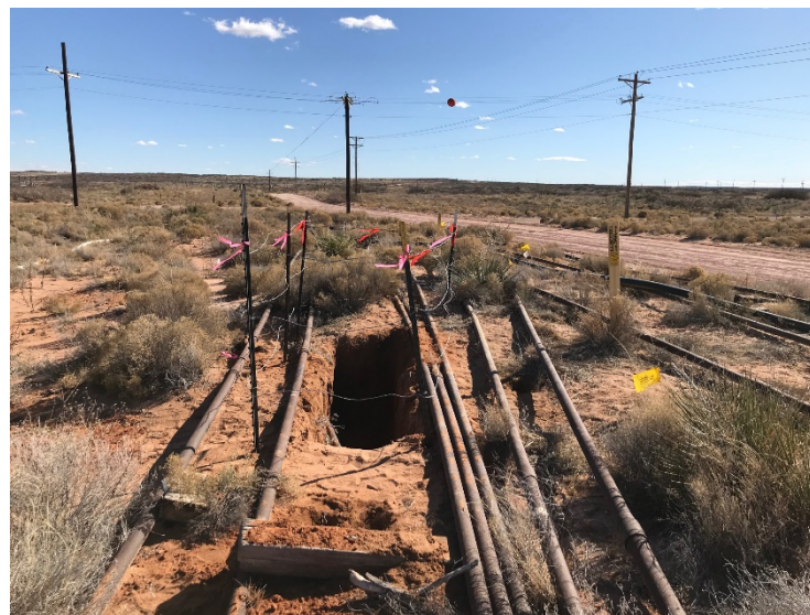
Photograph 2: Southeast facing view of the excavation.
