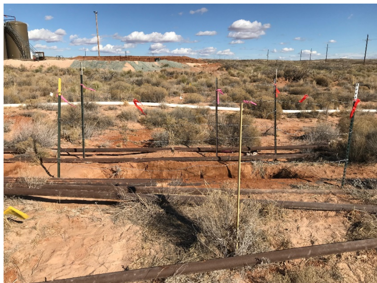
Photograph 3: North facing view of the excavation.
