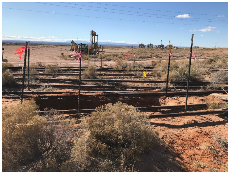
Photograph 1: South facing view of the excavation.
