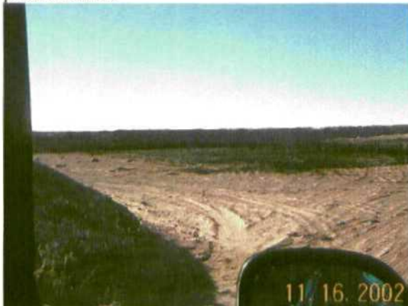
Photo 2. Cell 1 contaminated soils are tilled. Cell has one piece of trash (squashed container).
