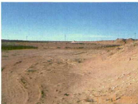
Photo 3. Cell construction. Pile in the back right corner is clean fill.
