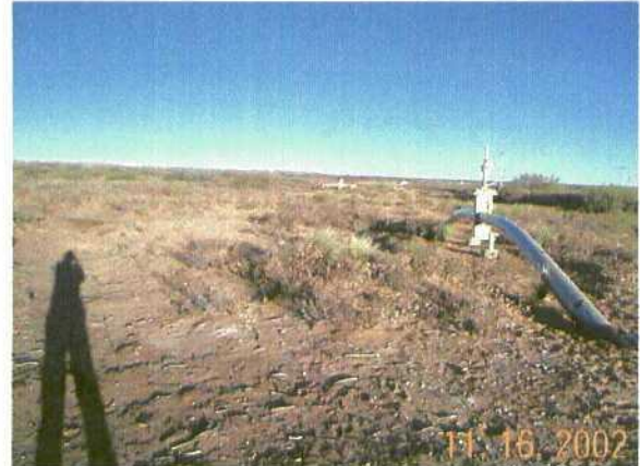
Photo 5. Pipeline ride-of-way west of the landfarm facility. Contaminated soil found in the pipeline ride-of-way.
