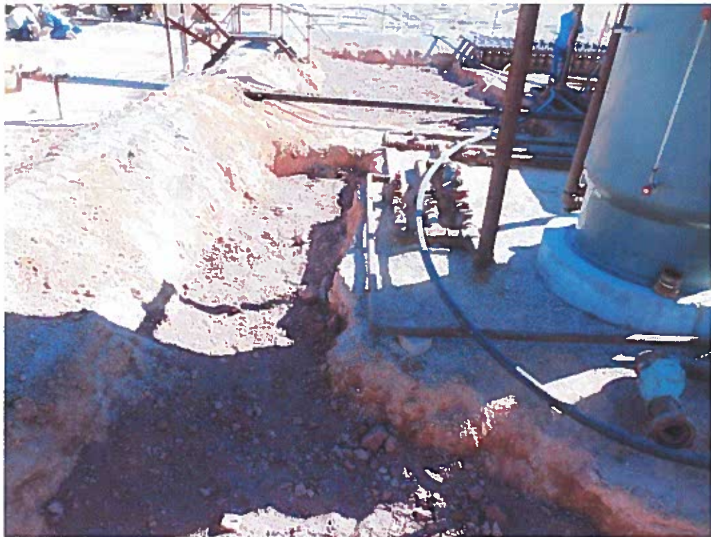
View East – AH-3 and AH-4 excavated with clay
