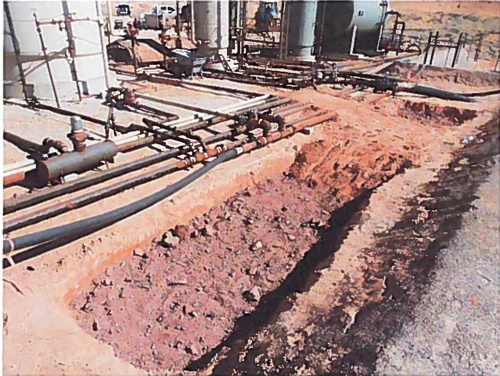
View East – AH-1 area at 2.0' with clay
