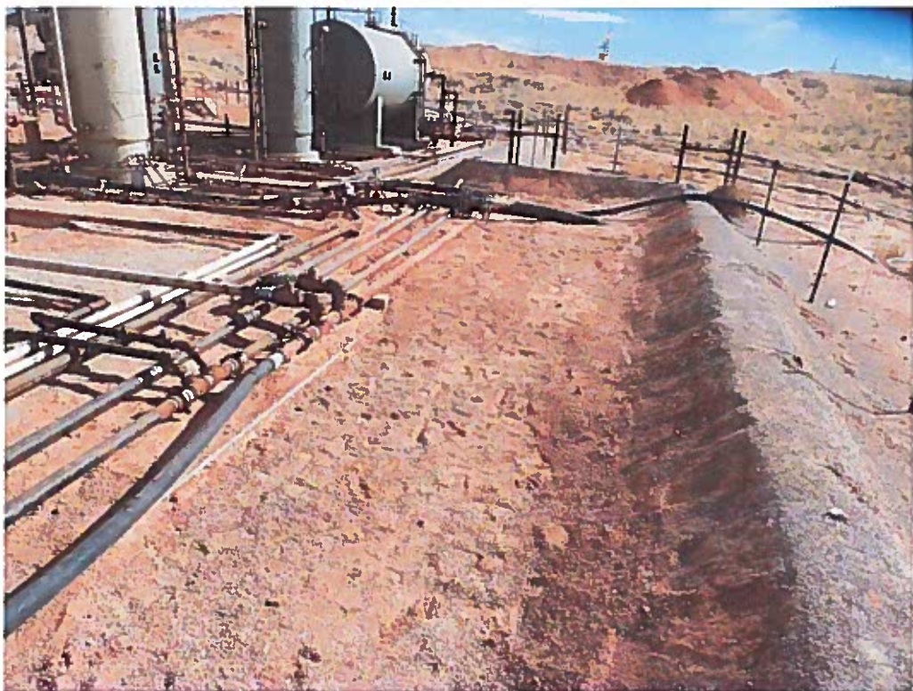
View East – AH-1 and AH-2 backfilled
