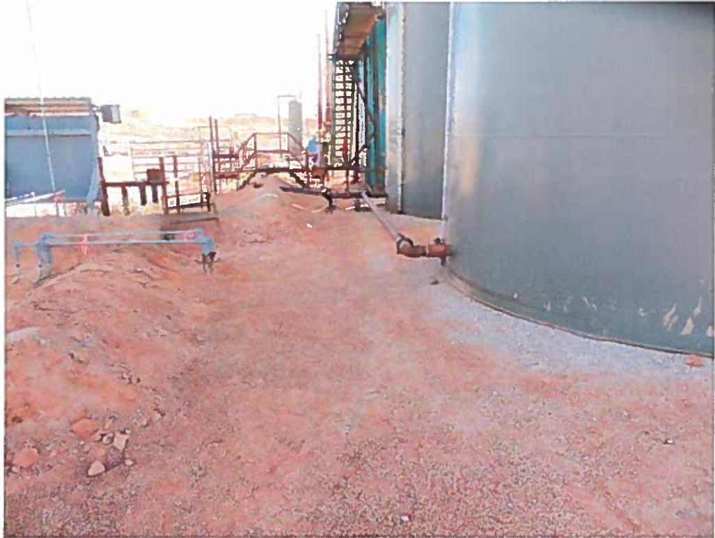
View East – Areas of AH-8 and AH-10 backfilled
