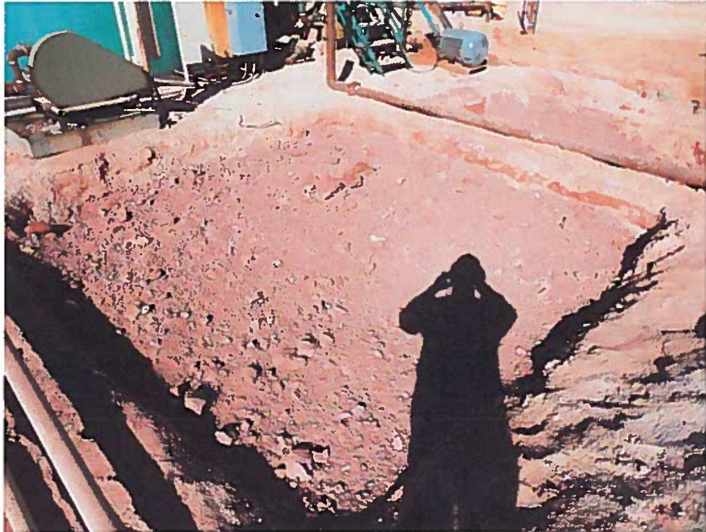
View North – AH-6 and AH-7 excavated with clay
