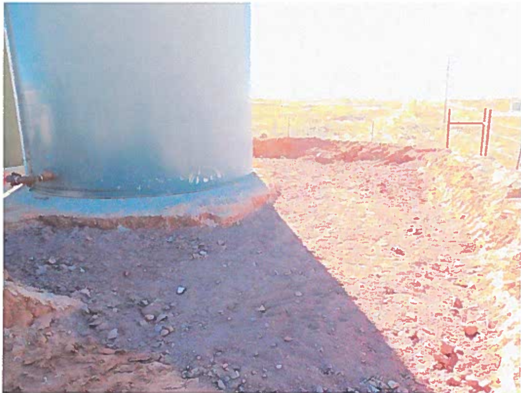
View South – Area of AH-12 excavated with clay
