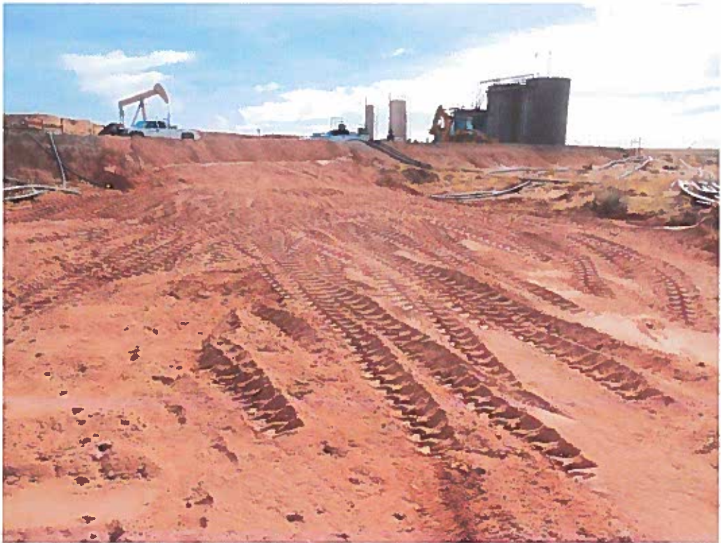
View East – AH-13 and AH-14 backfilled
