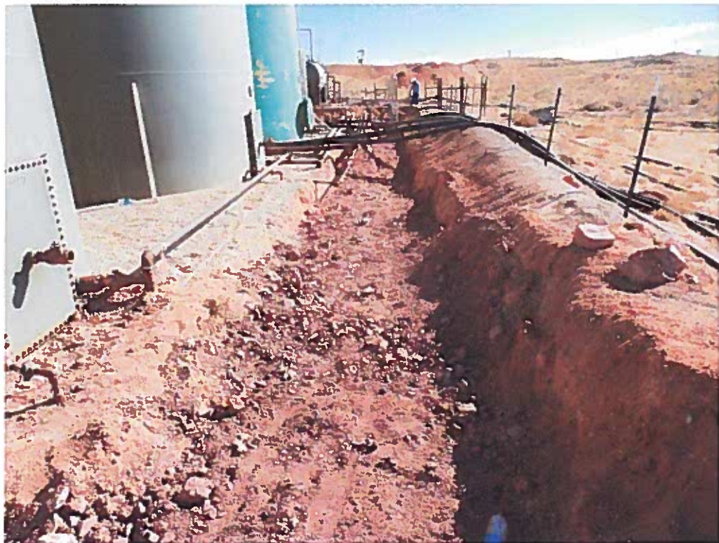
View East – AH-7, AH-9, and AH-11 excavated with clay
