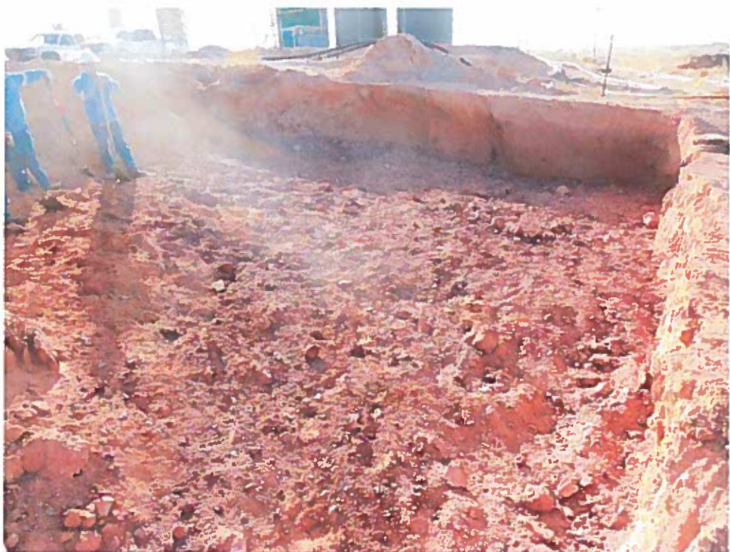
View South – Area of AH-13 excavated with clay
