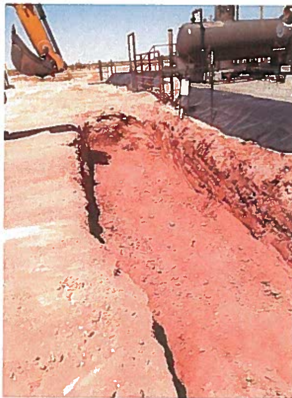
View West – Clay lined area of AH-1
