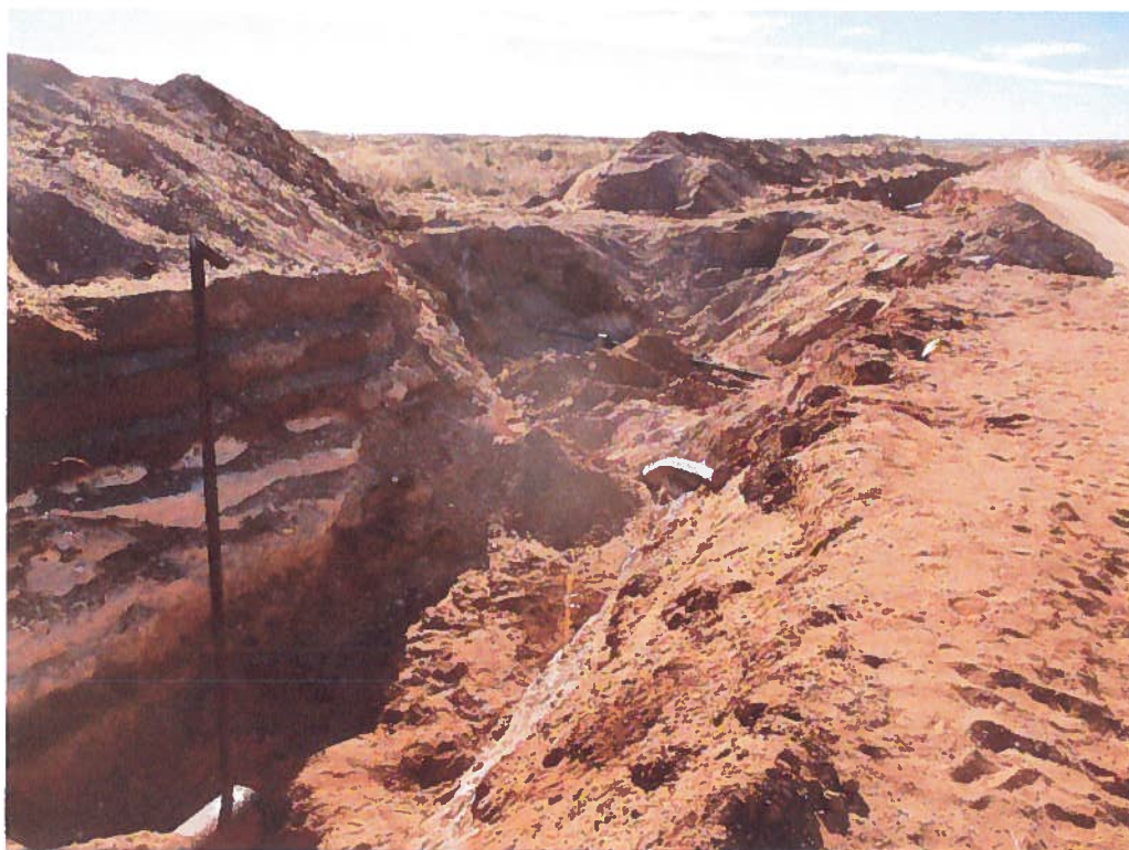
View West – Trench Area
