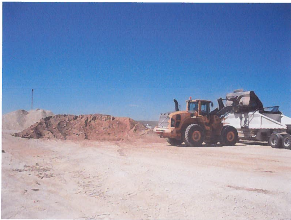
Loading impacted soil for disposal – 8/29/2014
