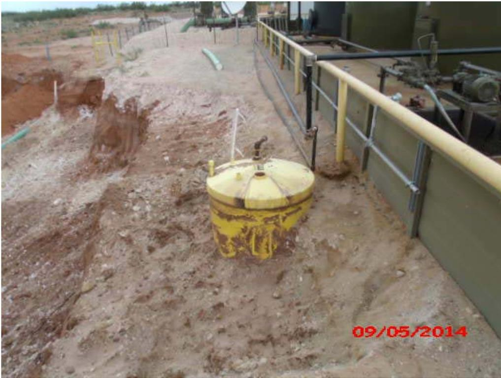
Photograph #5 – Excavated area around release point
