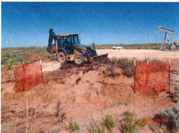
Scraping to 6 in bgs, facing northwest 9/9/14
