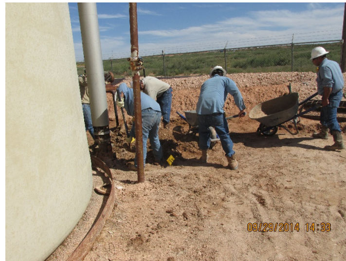
Hand-digging contaminated area 09/29/14
