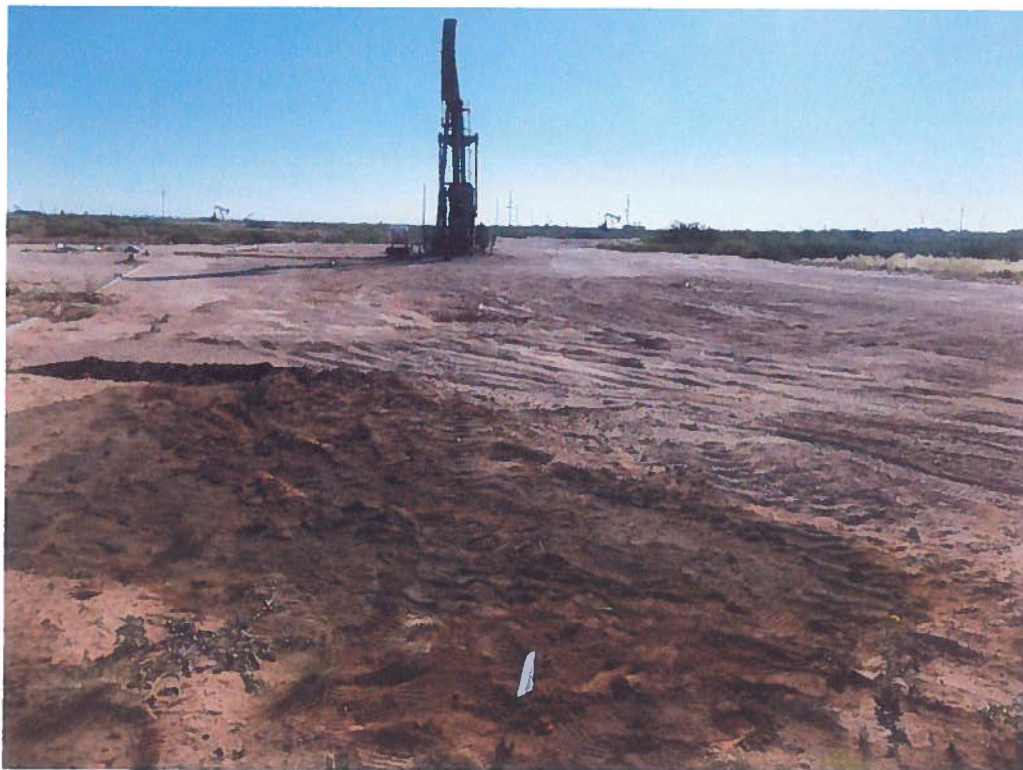
View East – AH-1, AH-2, AH-3, and AH-4
