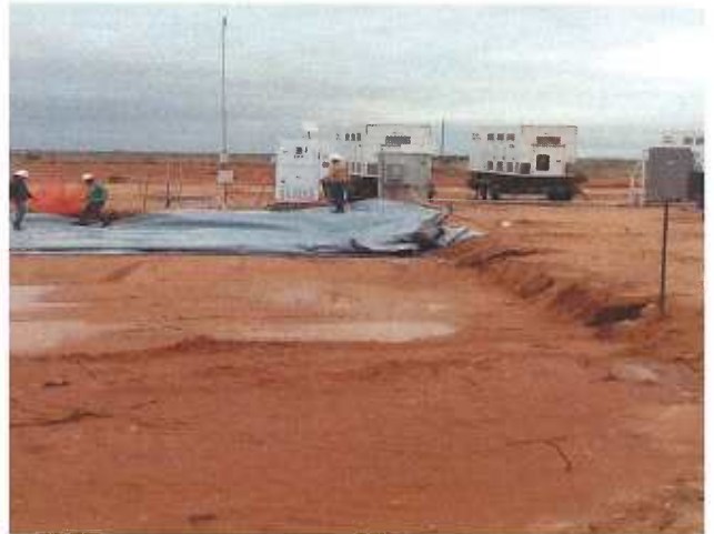
Liner Installation
