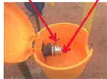
Loading Line Drain Valve
