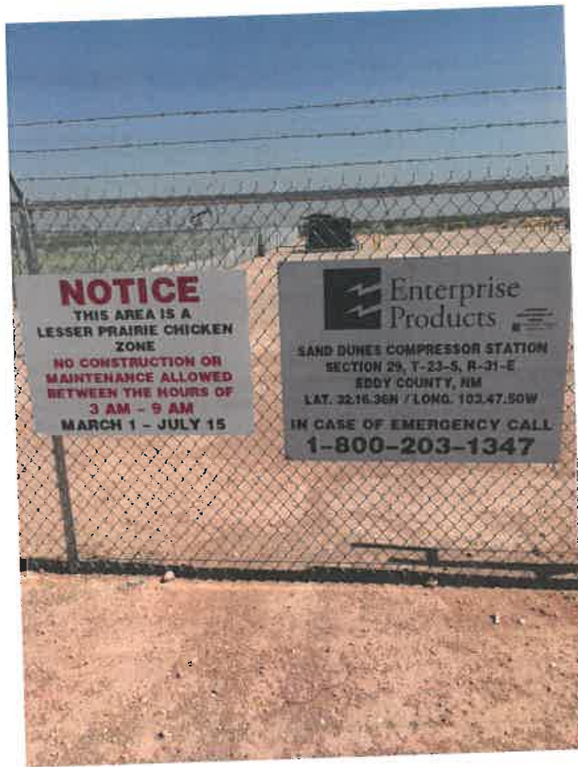
Fencing – 6 foot, 3-strand barbed wire
