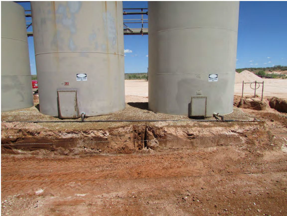
Middle of battery excavation facing North, August 18, 2016
