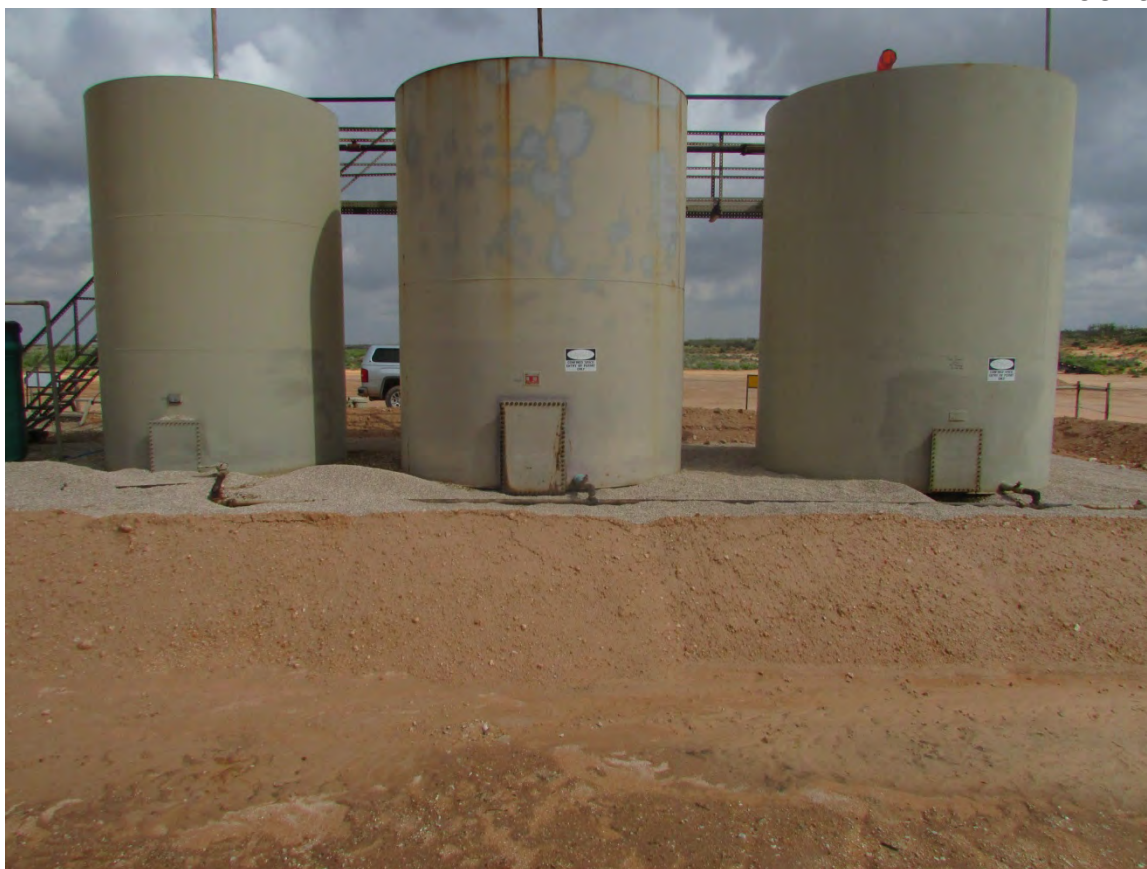
Middle of backfilled tank battery and new firewall facing North, September 3, 2016
