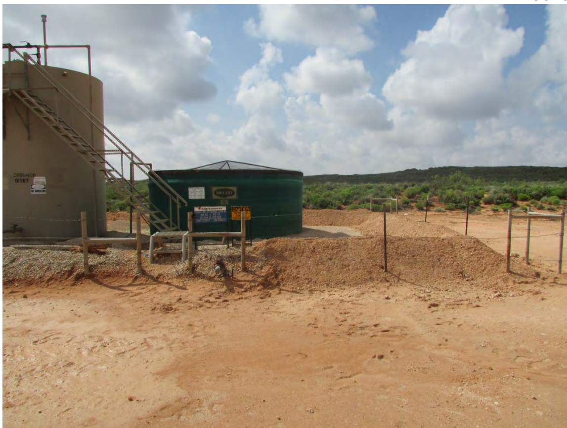
Northwest corner of backfilled tank battery and new firewall facing South, September 3, 2016
