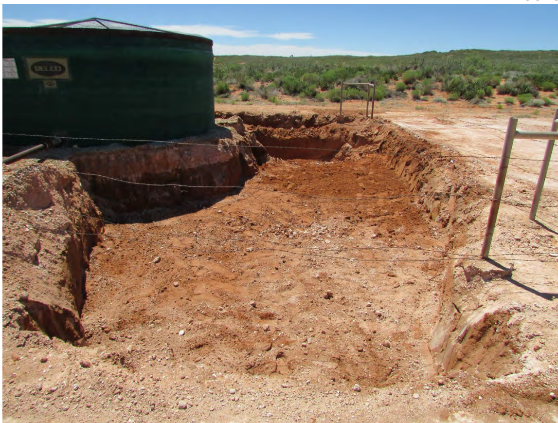
Northwest corner of battery excavation facing South, August 18, 2016
