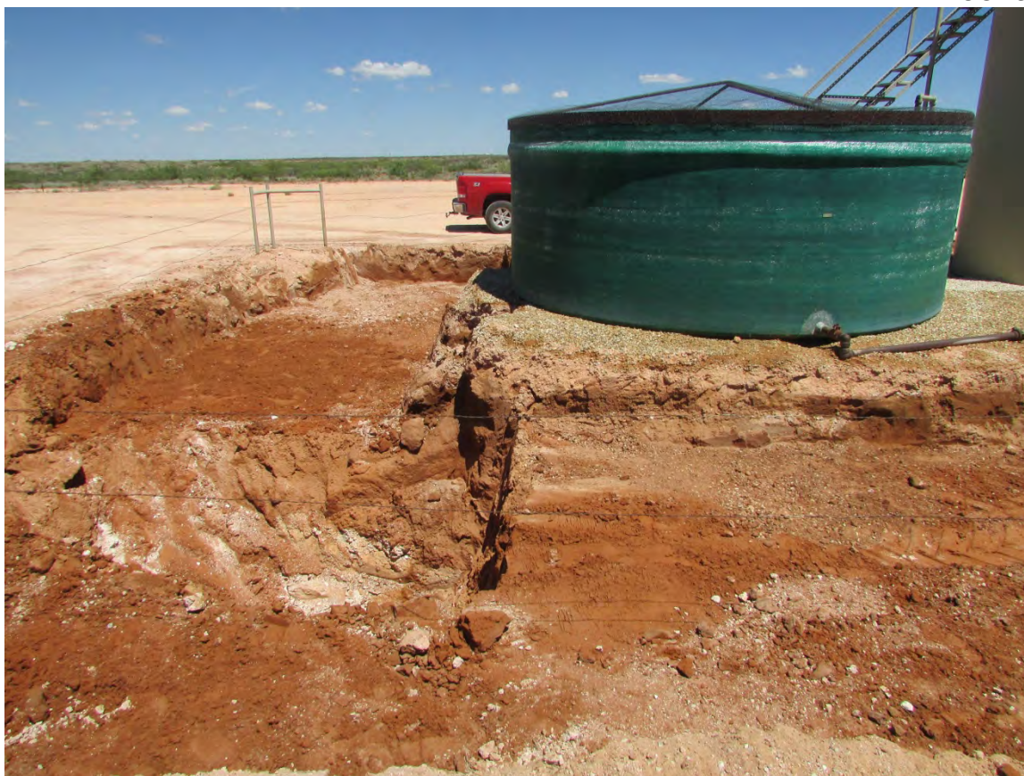
Southwest corner of excavation facing North, August 18, 2016
