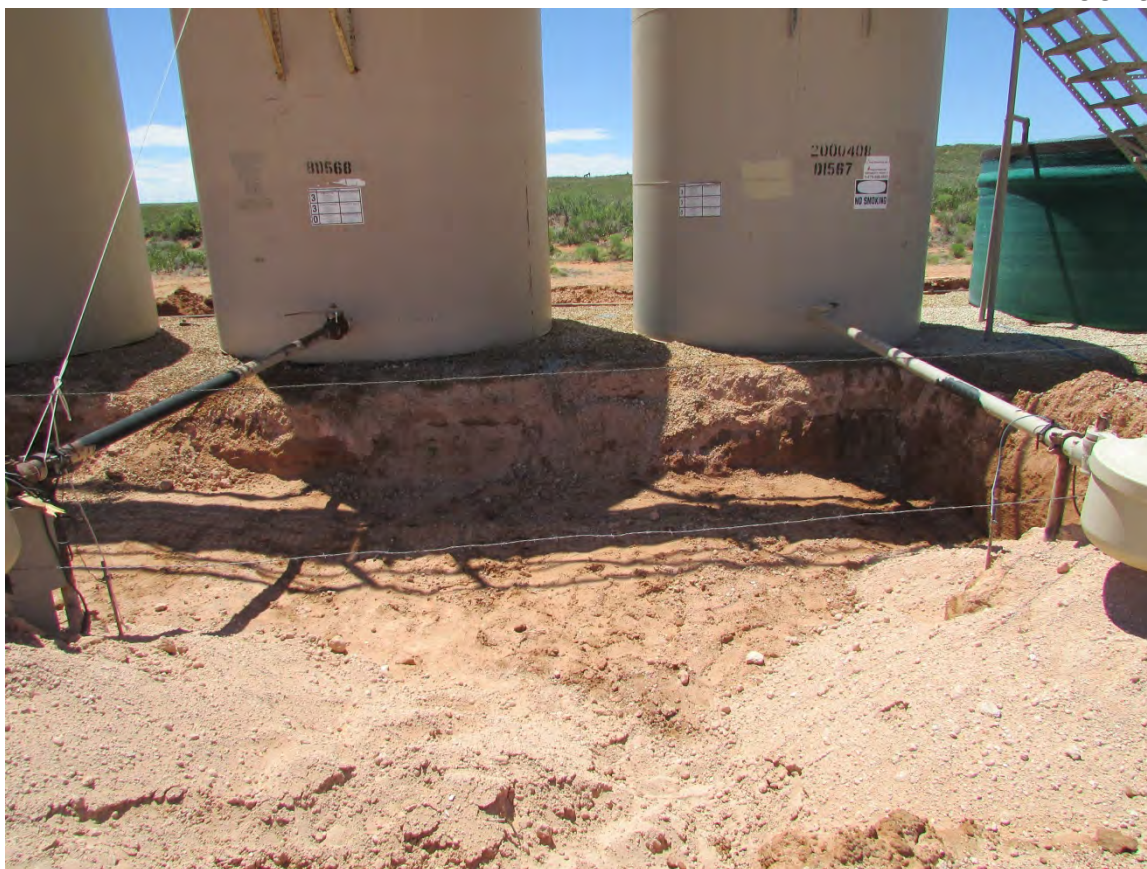
Middle of battery excavation facing South, August 18, 2016
