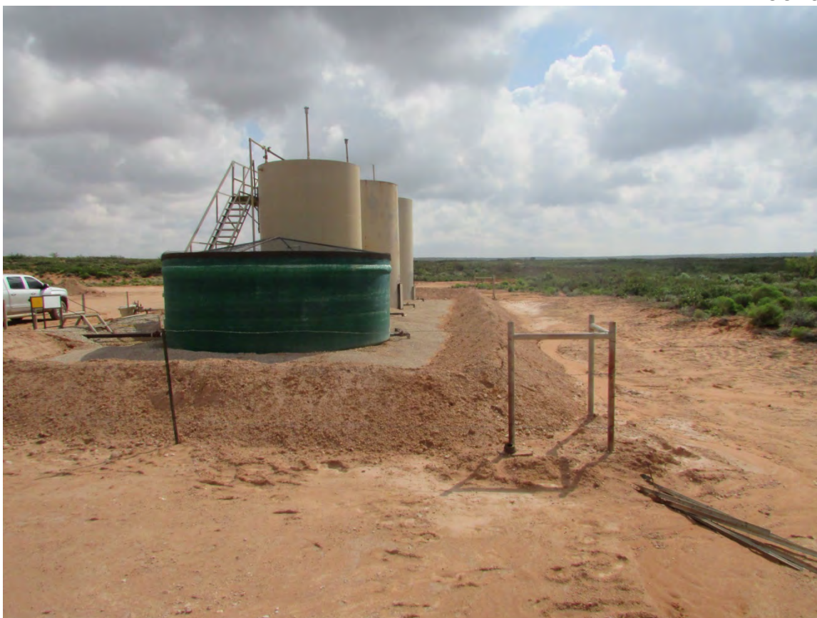
Southwest corner of backfilled tank battery and new firewall facing East, September 3, 2016
