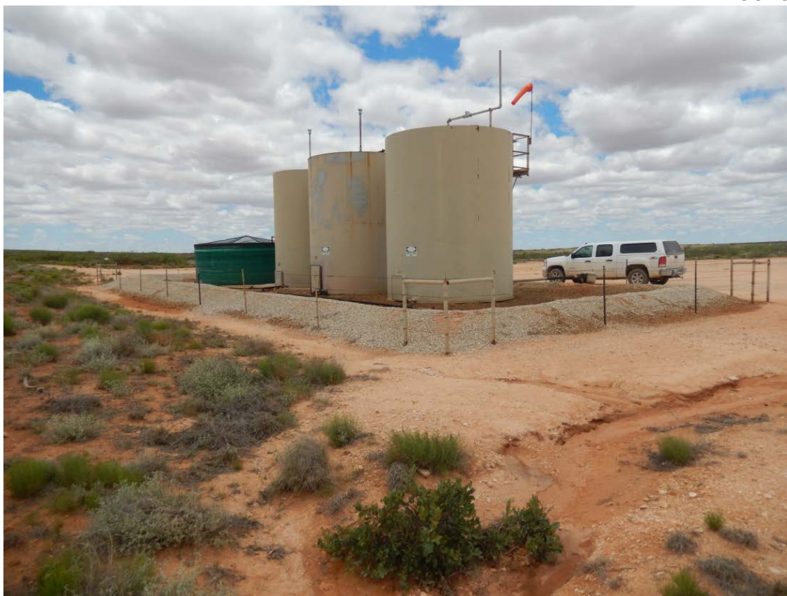
Stained Area inside and outside firewall facing Northeast, June 1, 2016
