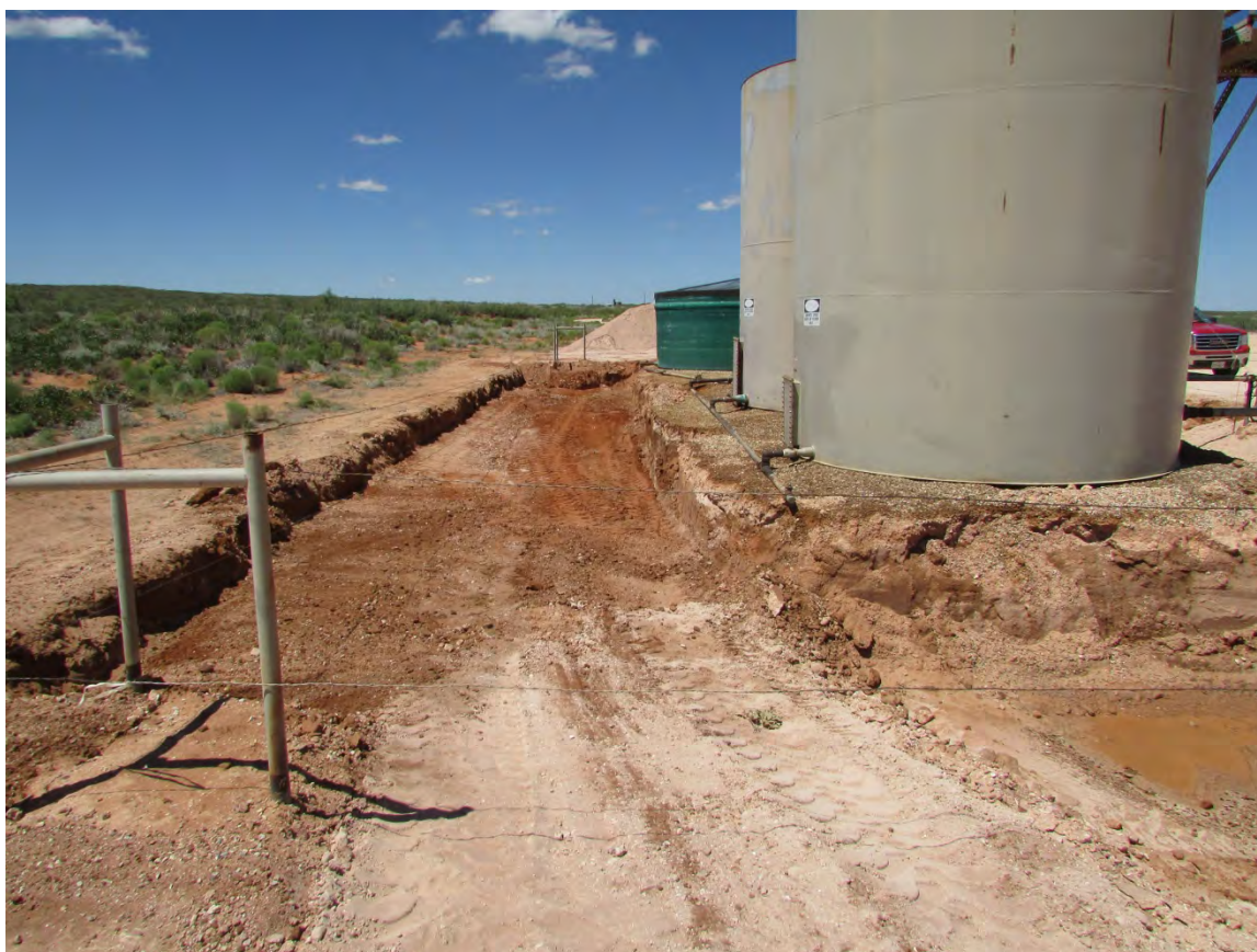
East side of battery excavation facing West, August 18, 2016
