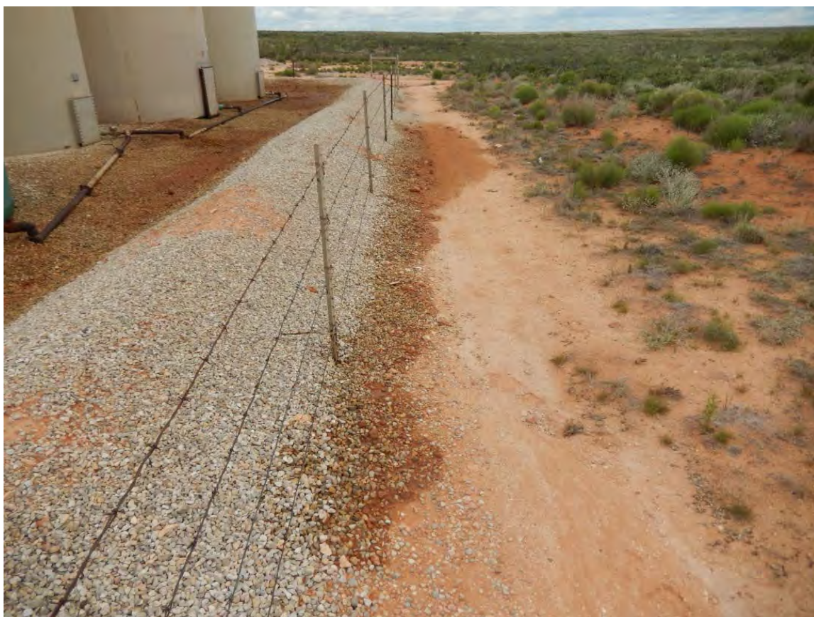
Stained Area inside and outside firewall facing West, June 1, 2016
