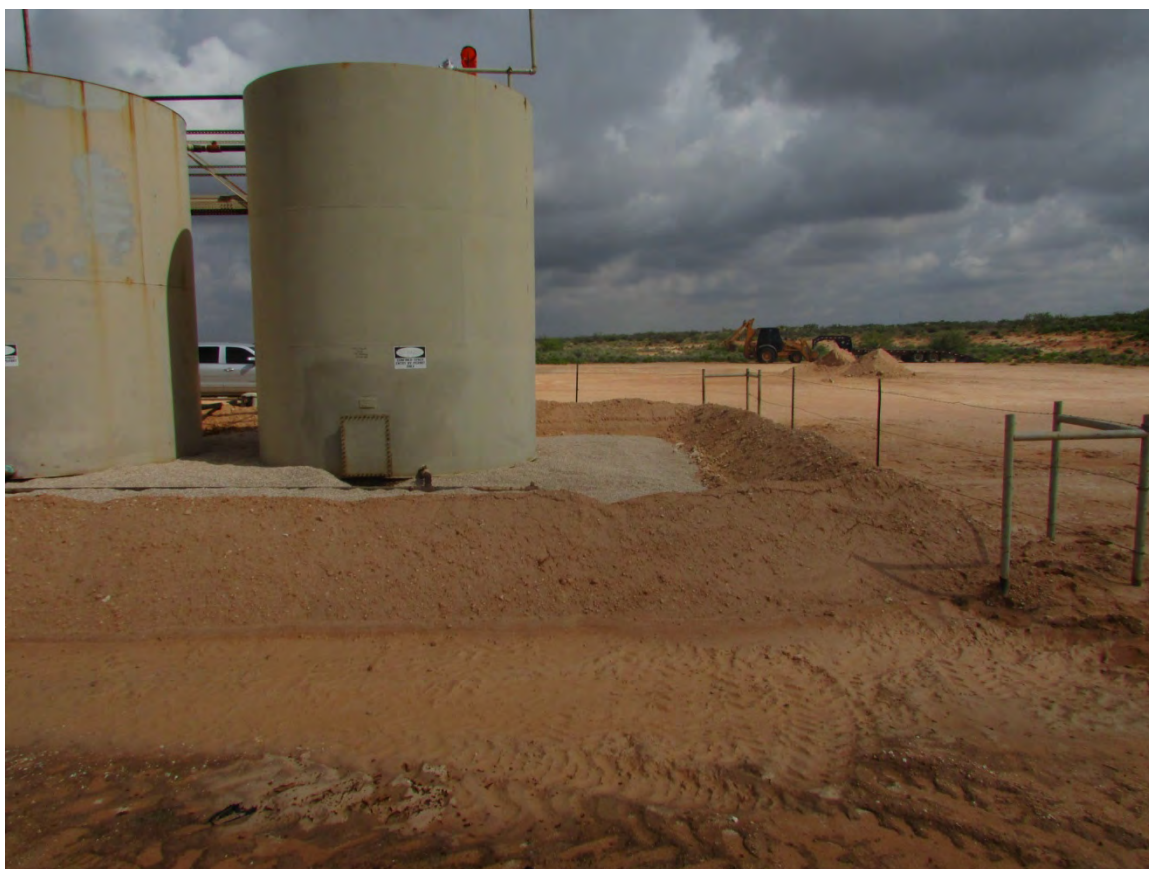
Southeast corner of backfilled tank battery and new firewall facing North, September 3, 2016
