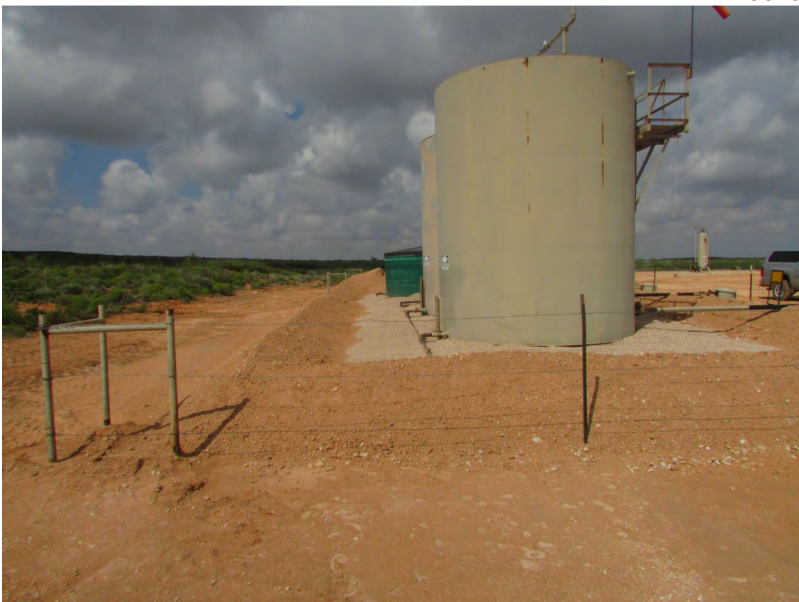
Southeast corner of backfilled tank battery and new firewall facing West, September 3, 2016
