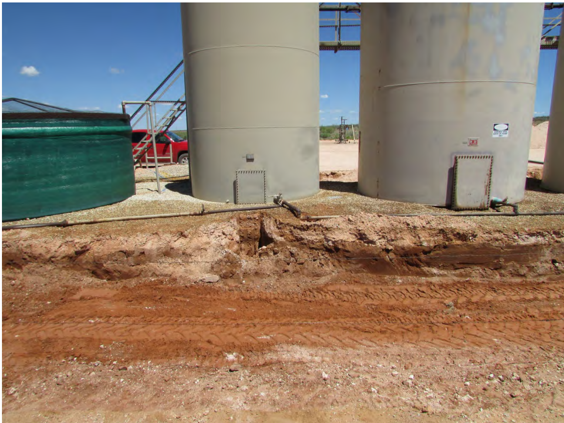
Middle of battery excavation facing North, August 18, 2016
