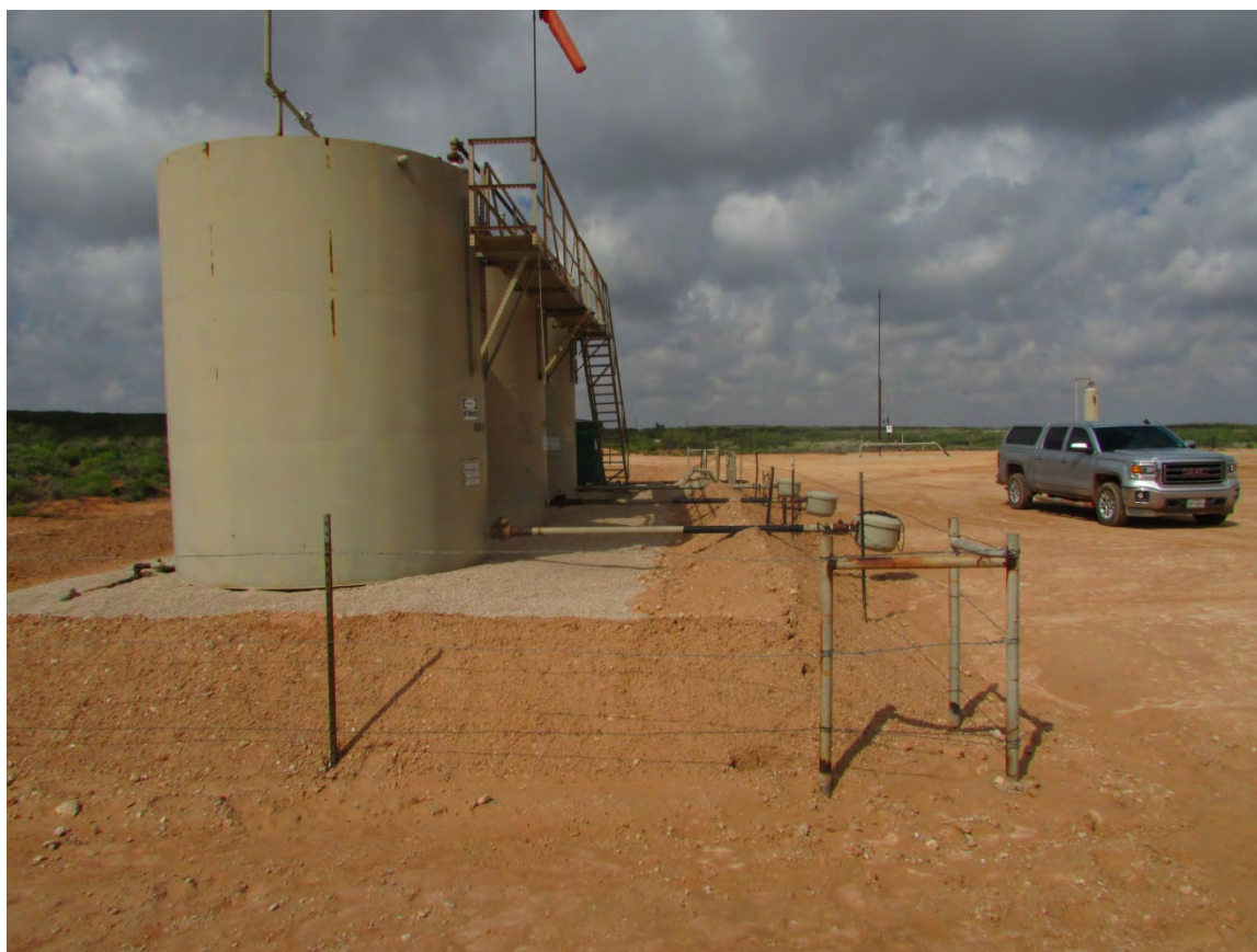
Northeast corner of backfilled tank battery and new firewall facing West, September 3, 2016
