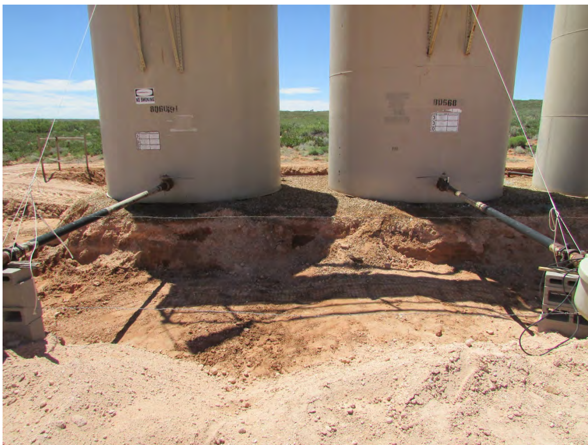
Middle of battery excavation facing South, August 18, 2016
