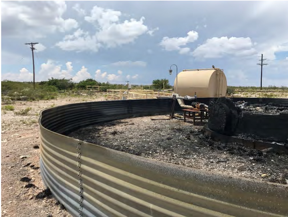
Indian Basin Station 210 – Release (Looking Northwest)
