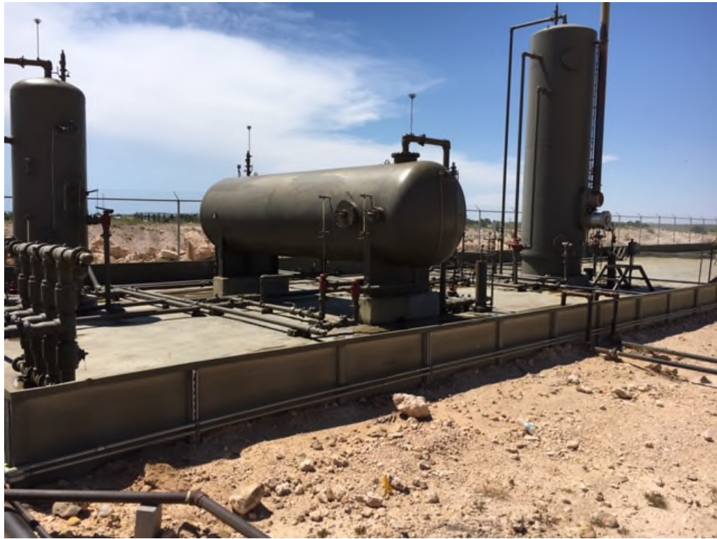
View West – Release area inside lined containment
