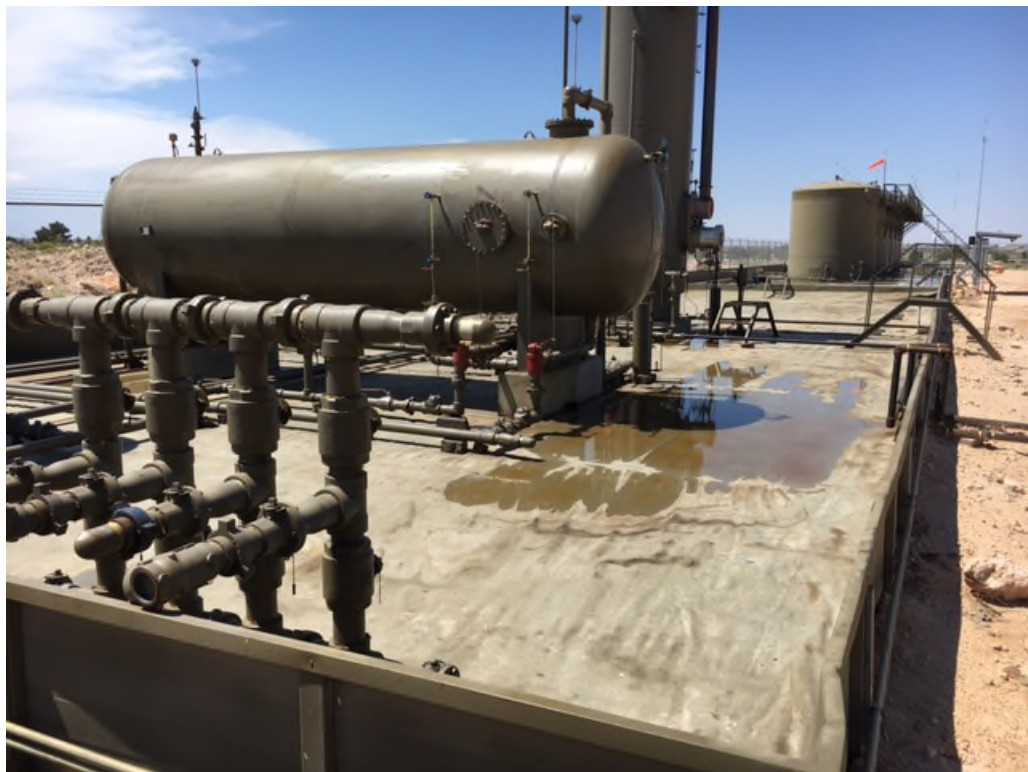
View North - Release area inside lined containment
