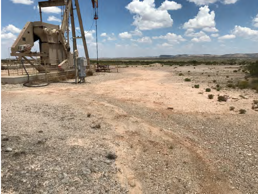
Indian Basin Station 210 – Release (Looking East)
