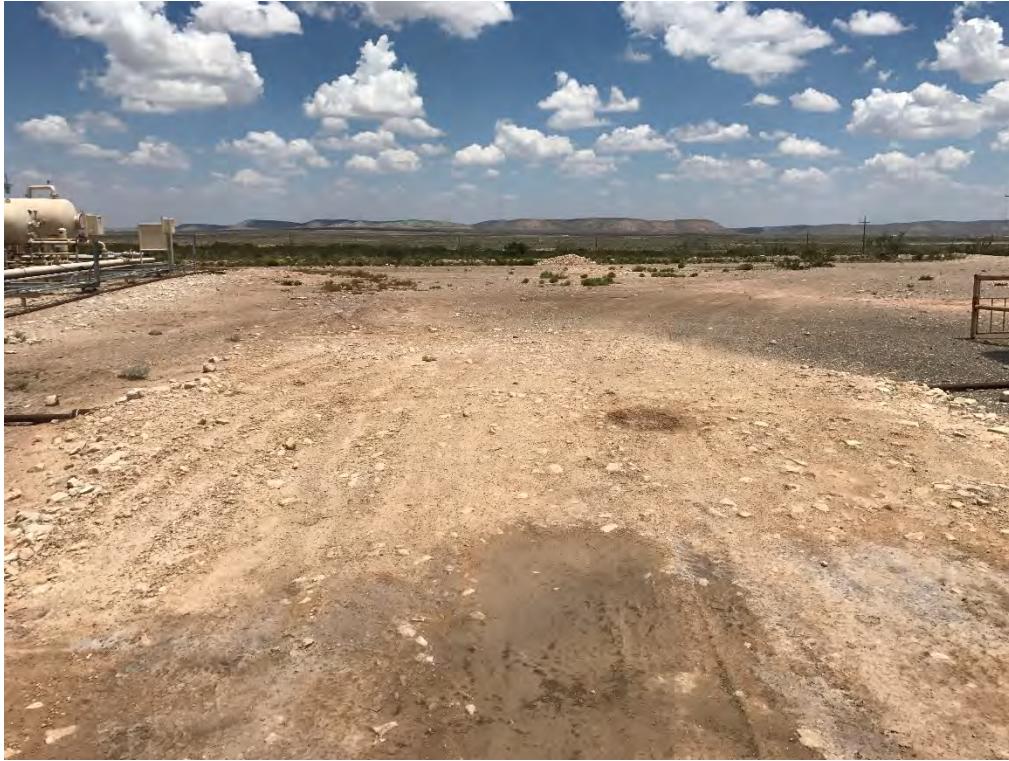
Indian Basin Station 210 – Release (Looking East)
