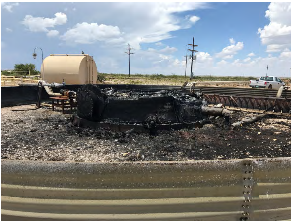
Indian Basin Station 210 - Release (Looking Northwest)
