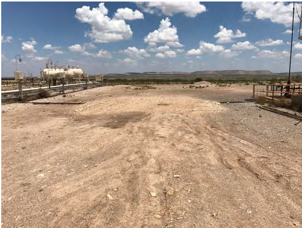
Indian Basin Station 210 – Release (Looking East)
