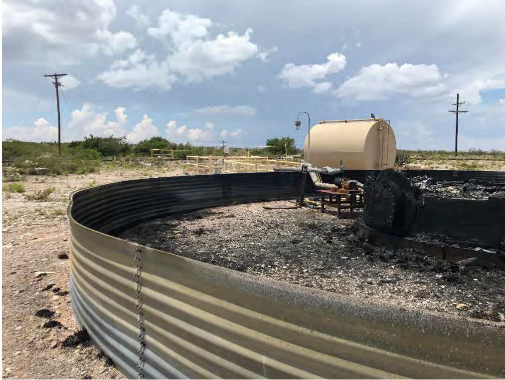
Indian Basin Station 210 – Release (Looking Northwest)
