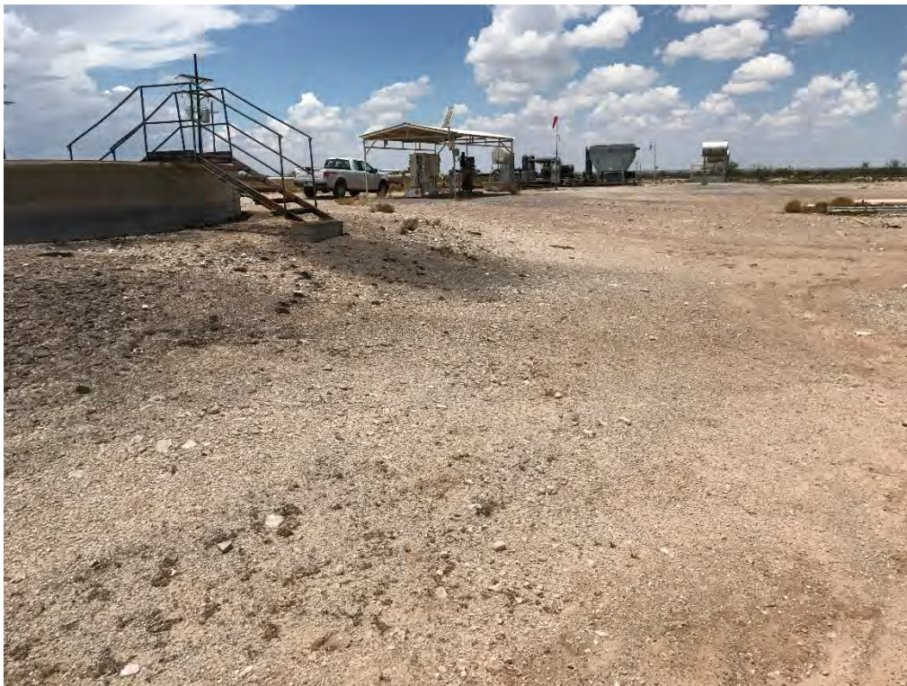
Indian Basin Station 210 – Release (Looking Northwest)
