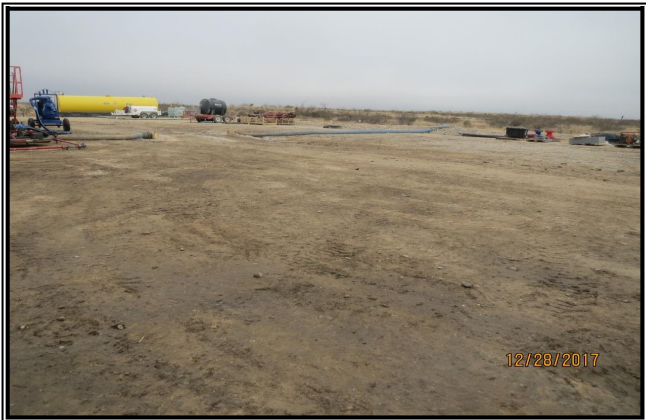
View of impacted area looking northeast.
