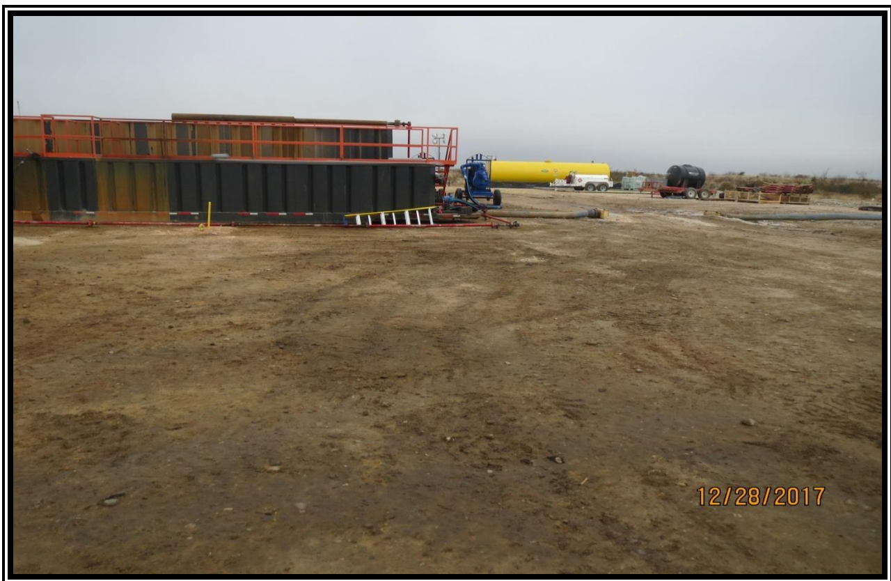
View of impacted area looking north.
