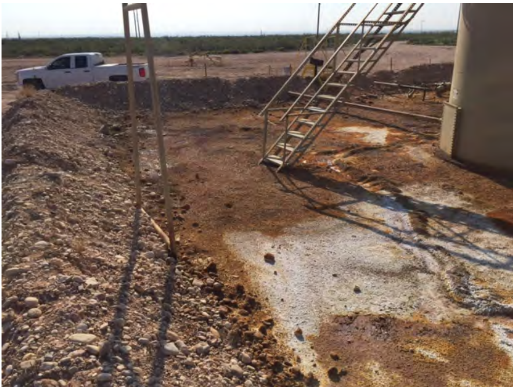
NEL 4 SWD Battery – Release (Looking East-Southeast)
