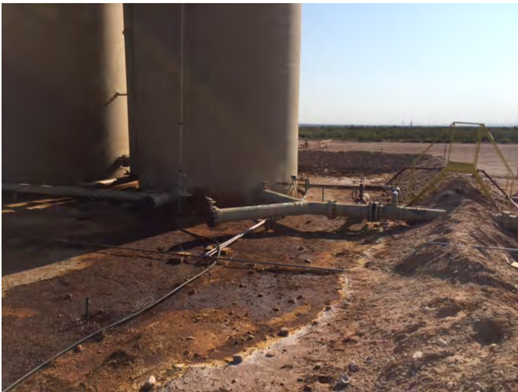
NEL 4 SWD Battery – Release (Looking East-Northeast)
