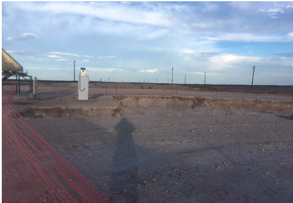
Photo 1. Excavation looking east
