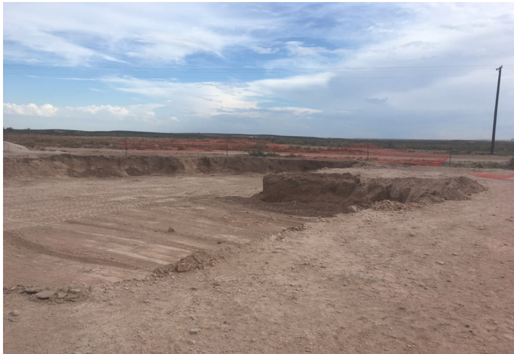
Photo 4. Excavation looking southeast
