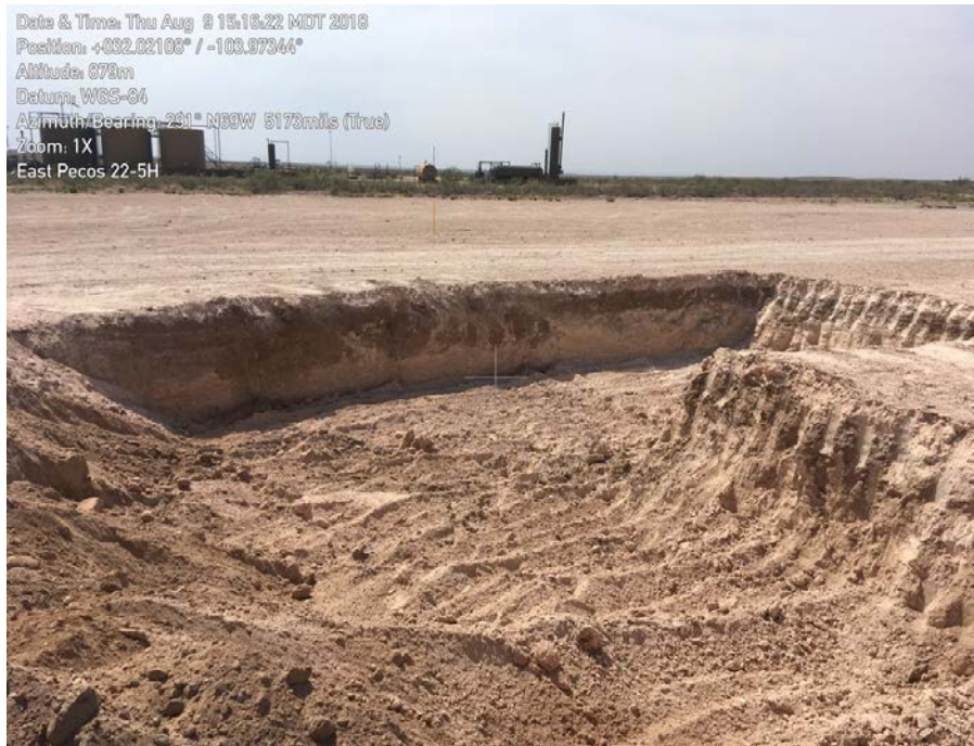
Photo 1. Excavation looking west
