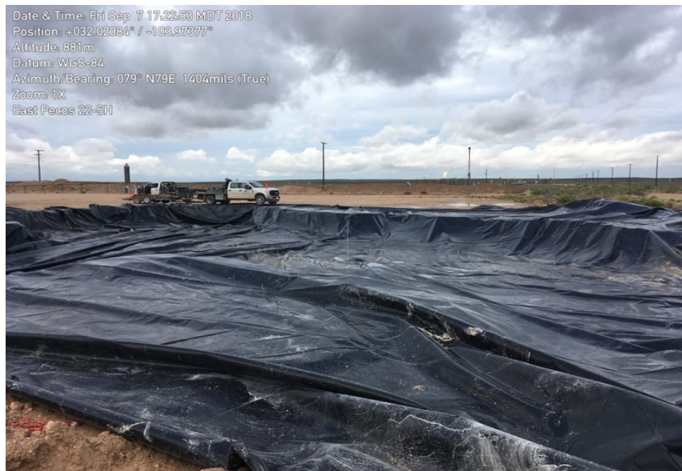
Photo 2. Excavation with liner looking east
