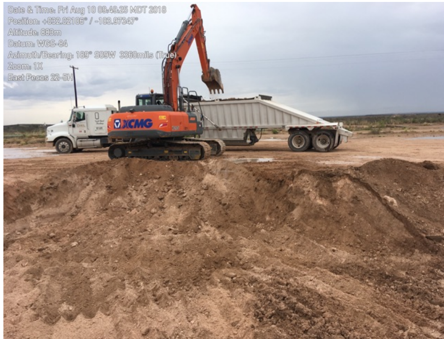
Photo 3. Excavator loading truck looking south
