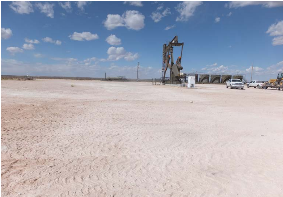
Photo 1. Overview of spill area facing north
