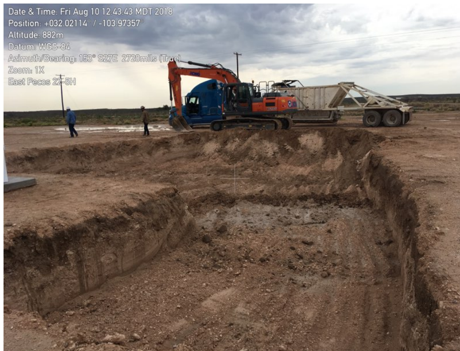
Photo 4. Excavator loading truck looking east
