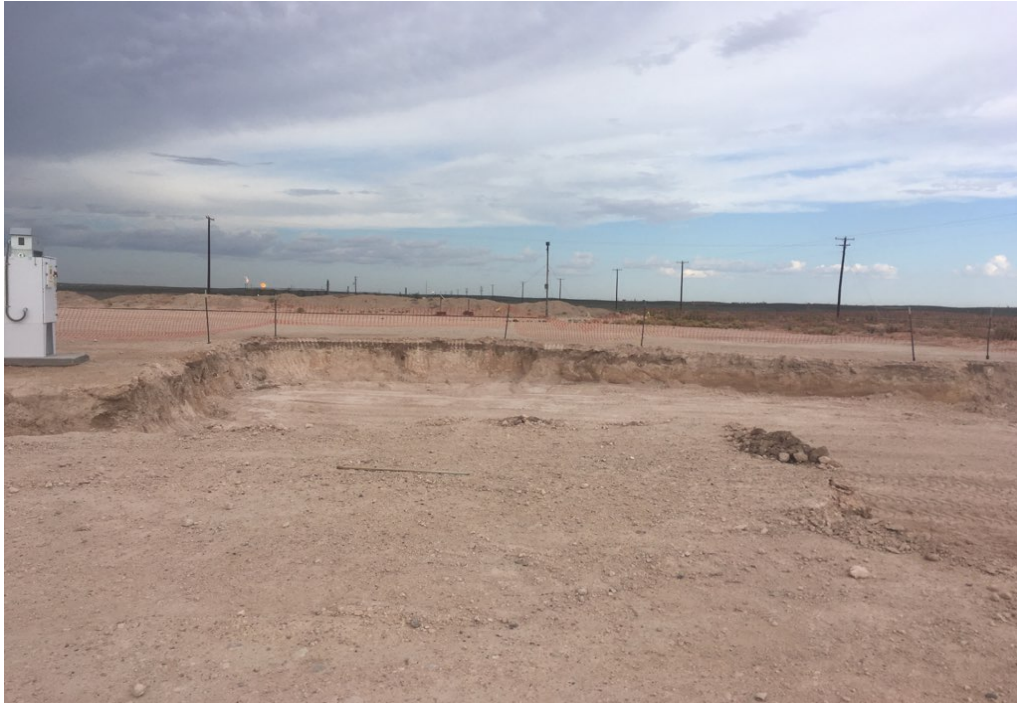
Photo 3. Excavation looking east
