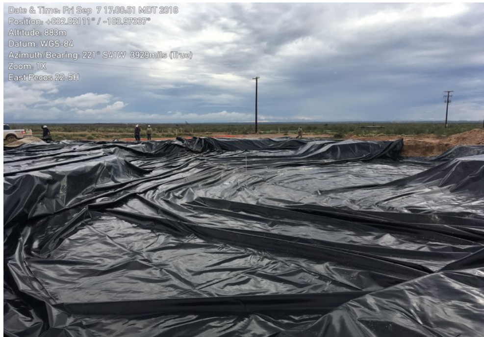
Photo 1. Excavation with liner looking south
