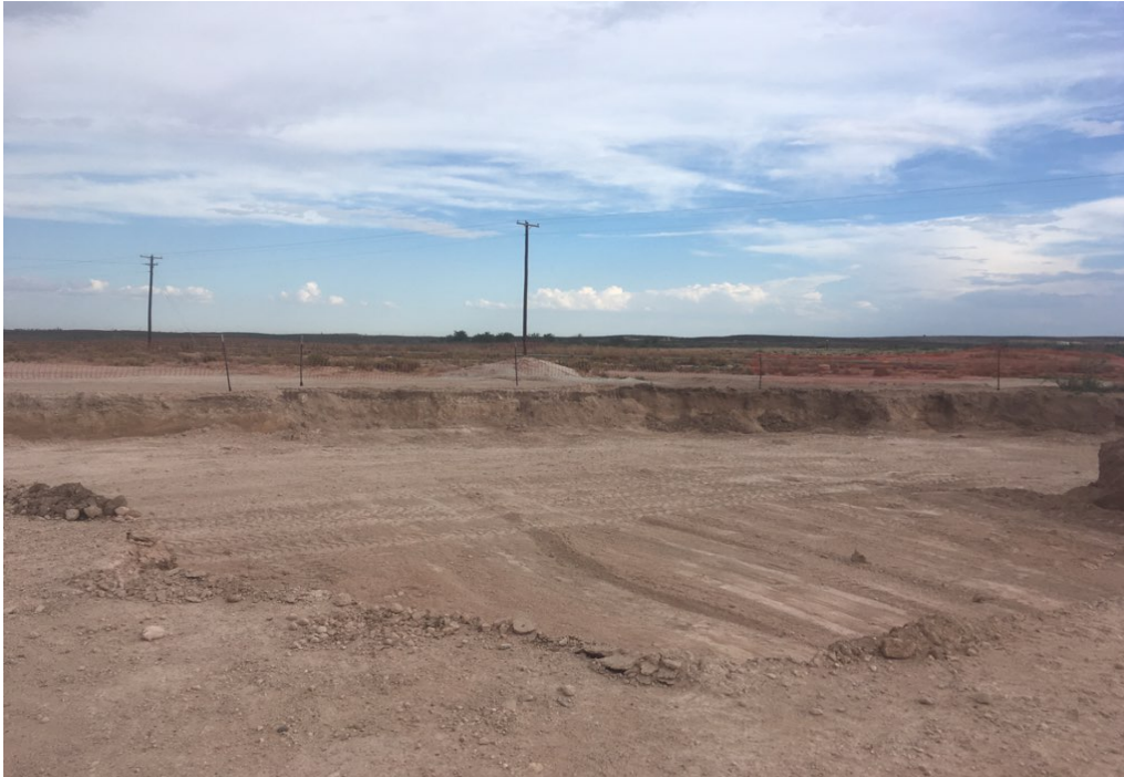
Photo 5. Excavation looking southeast
