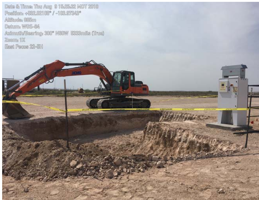
Photo 2. Excavation marked/blocked off looking west
