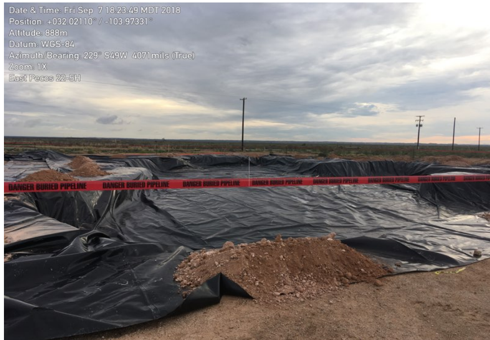
Photo 3. Excavation with liner weighted down looking south
