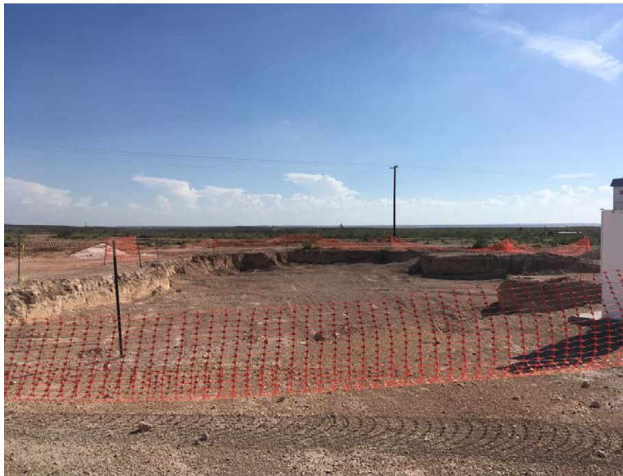
Photo 6. Completed excavation looking south
