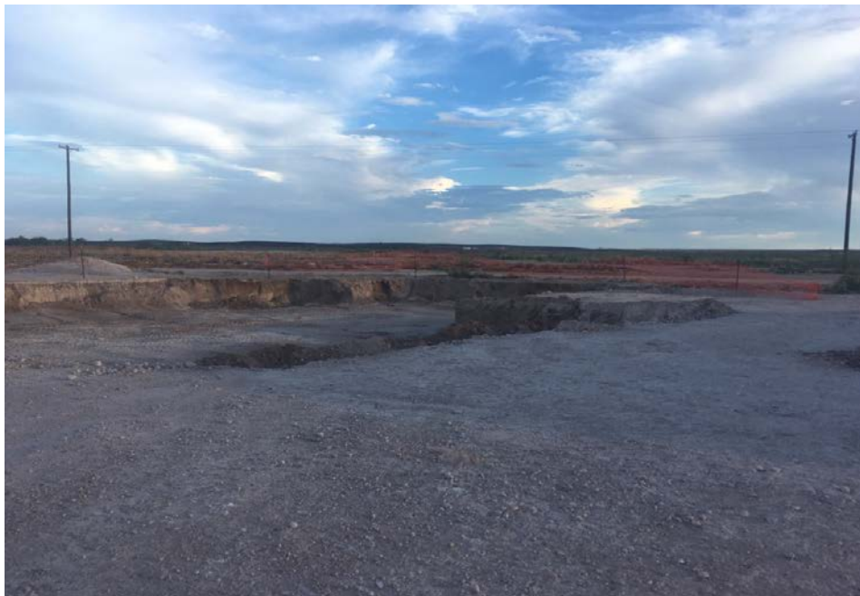
Photo 2. Excavation looking southeast
