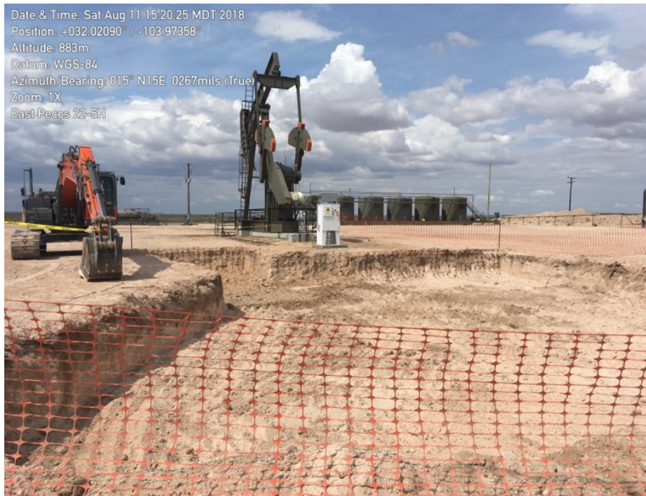
Photo 5. Excavation fenced off looking north
