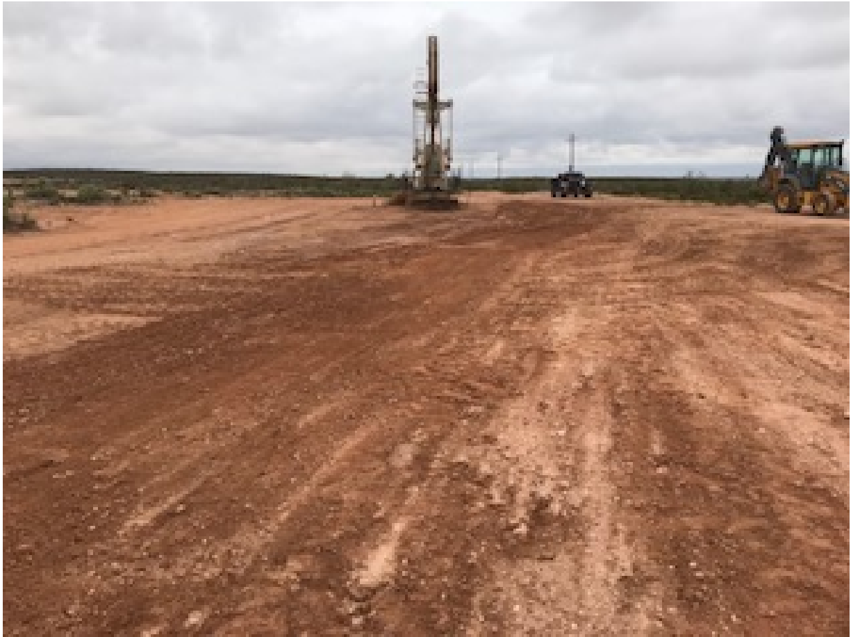
Release footprint on pad surface after excavation – view west
