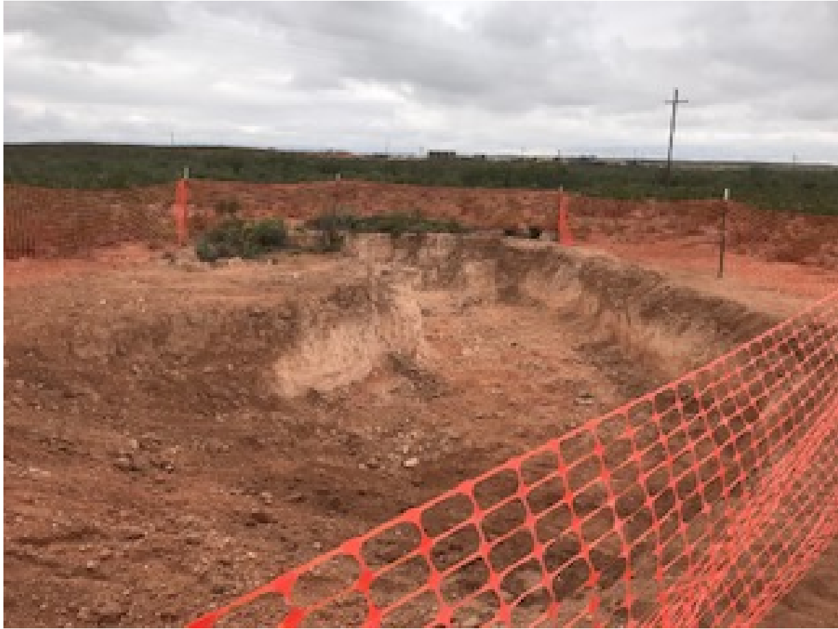
Excavation area in pasture – view north
