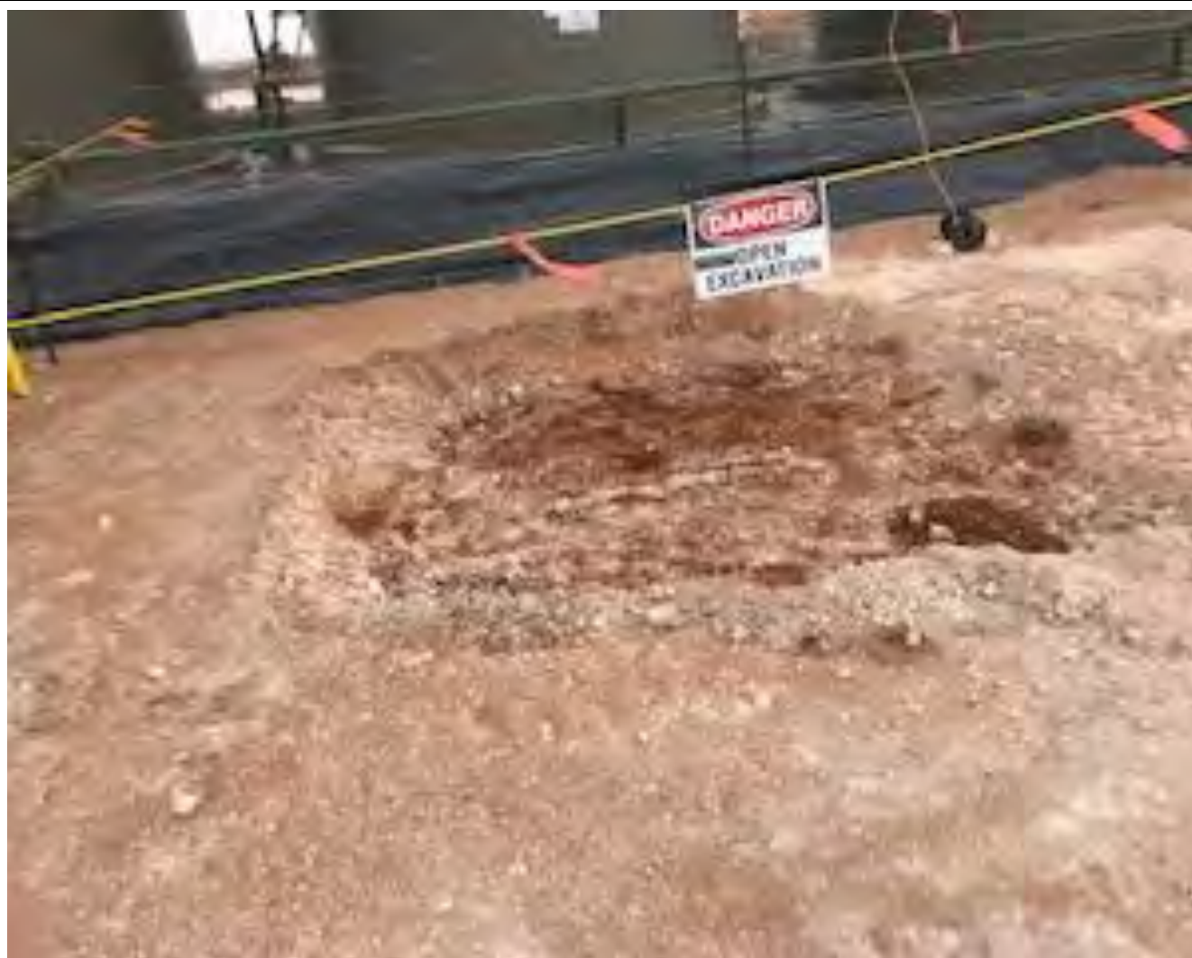
Southern view of the smaller excavation on the well pad.
