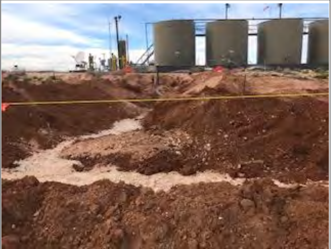
Northern view of the larger excavation in the pasture.
