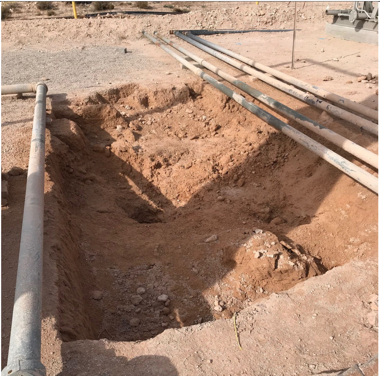
View south of southeastern excavation.
