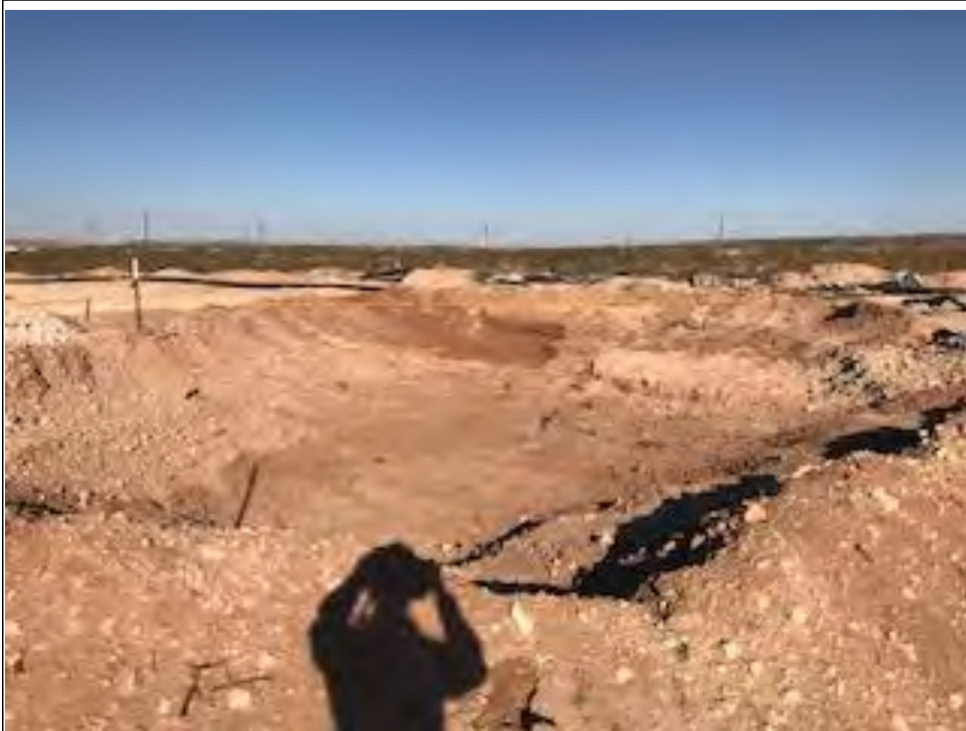
Eastern view of the final excavation extent. The sidewalls of the excavation are sloped, and the final excavation depth is 2.5 feet.
