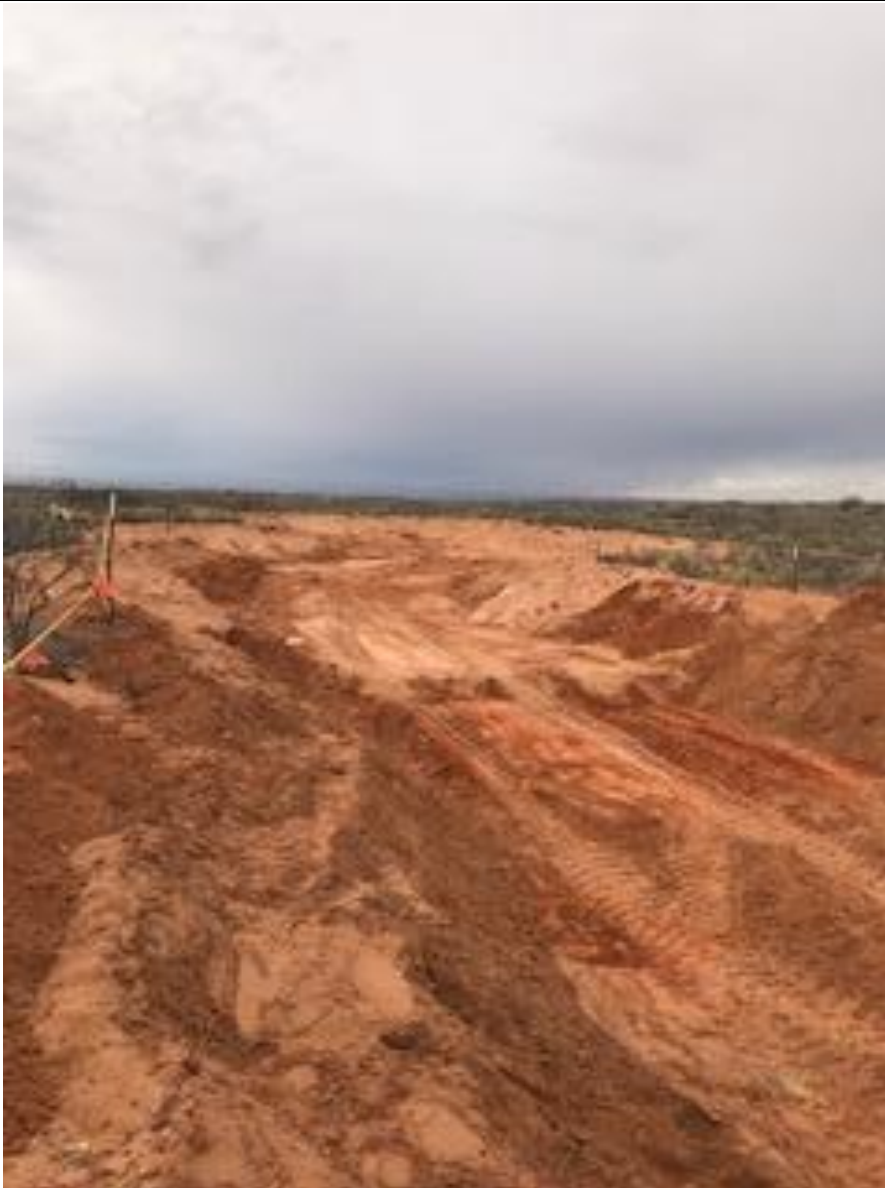
Western view of the final excavation extent.
