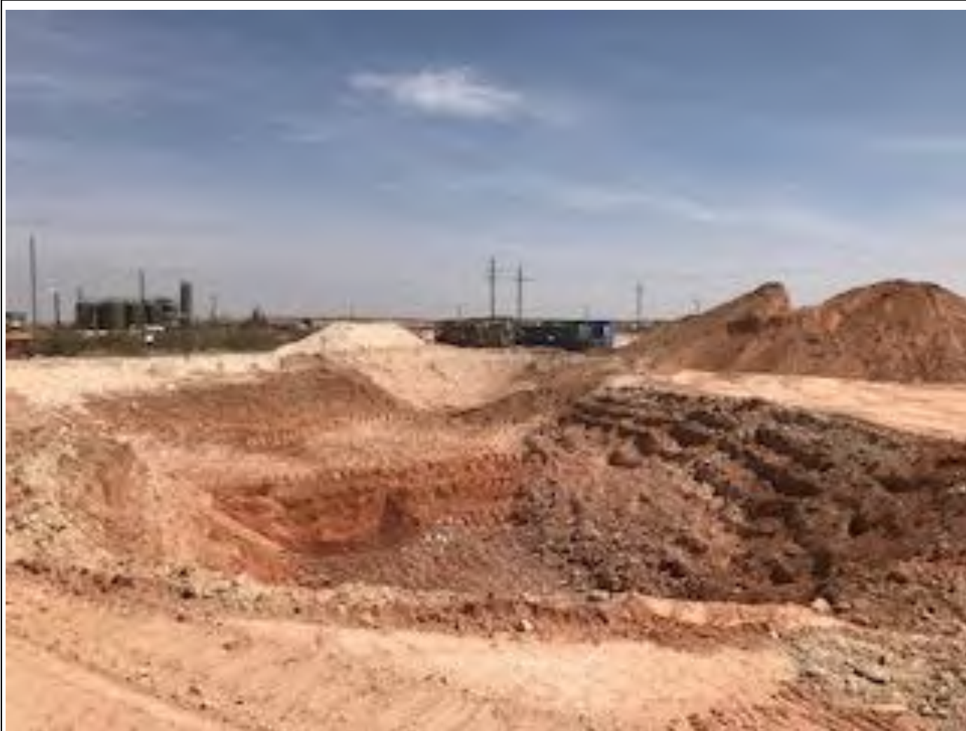
Western view of final excavation extent.
