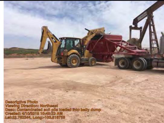
Contaminated soil pile loaded into belly dump
