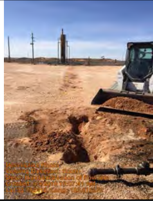
Hand excavation of flow line
