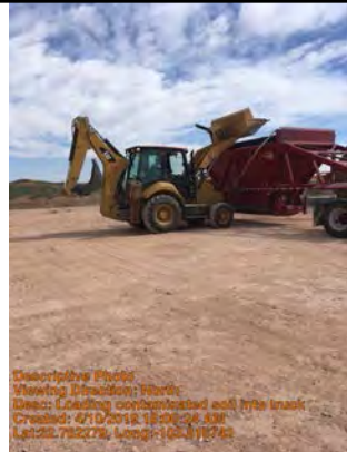
Loading contaminated soil into truck
