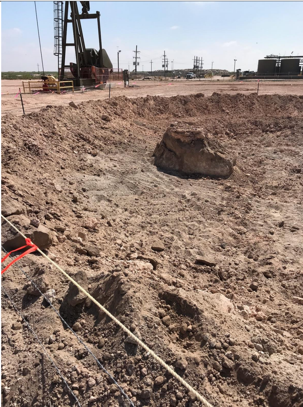
Northeastern view of final excavation extent.
