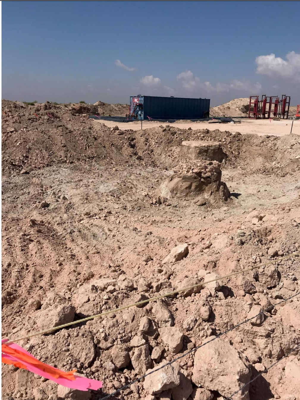
Northwestern view of final excavation extent.
