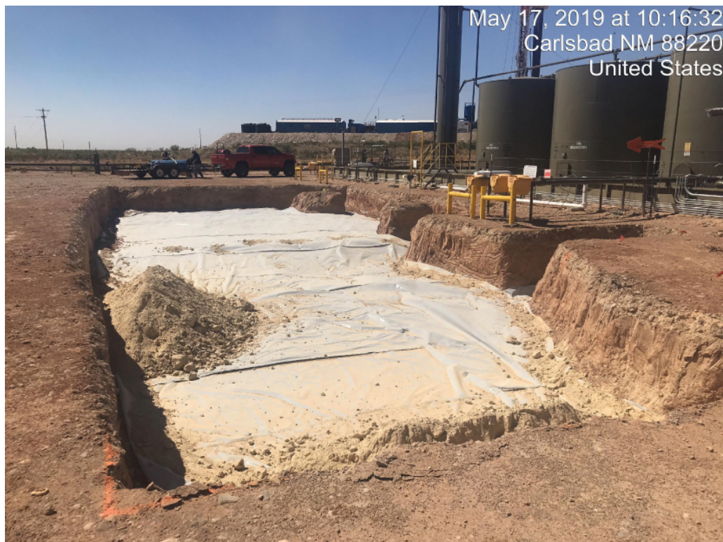
View South – Lined Excavation Area
