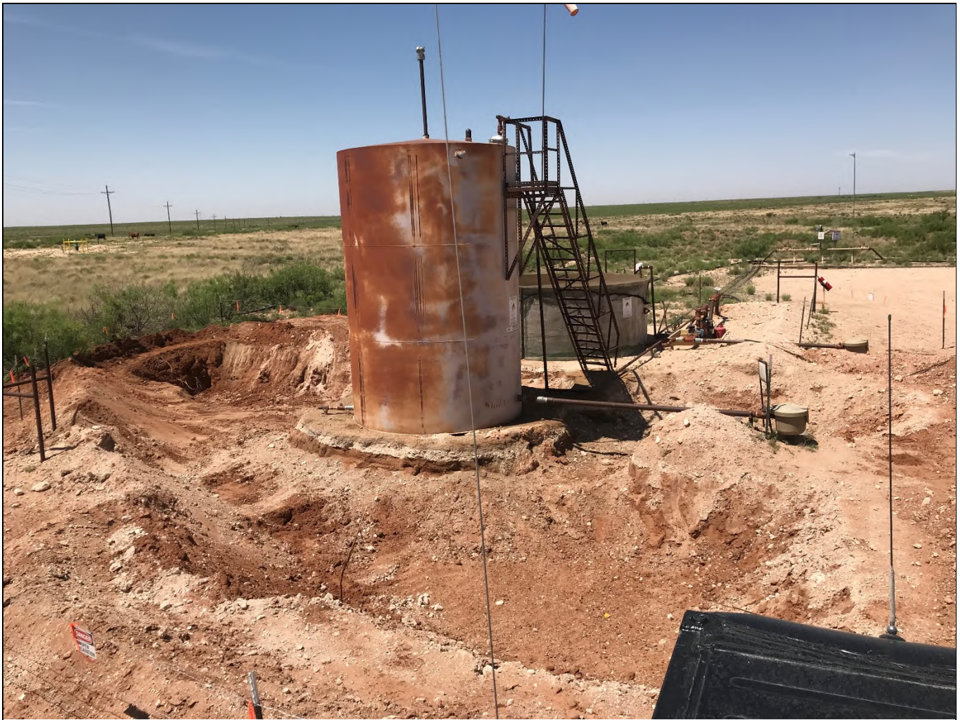
View facing southwest of the excavation.
