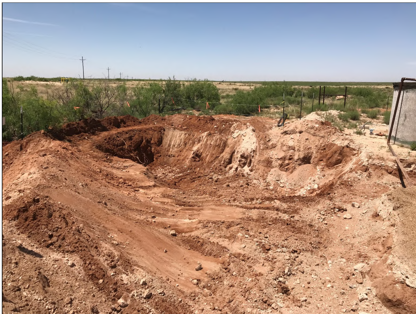
View facing southwest of the excavation.
