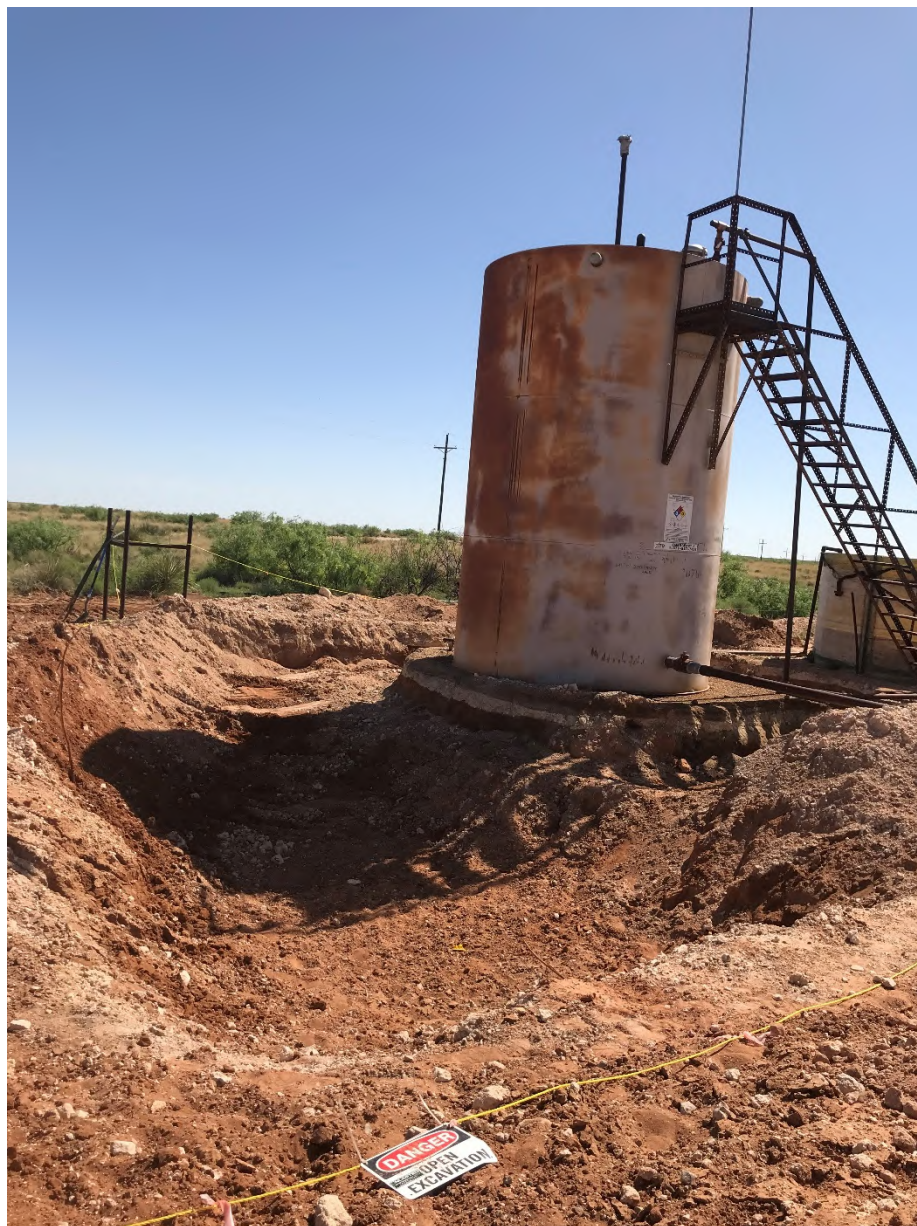
View facing south of the excavation.
