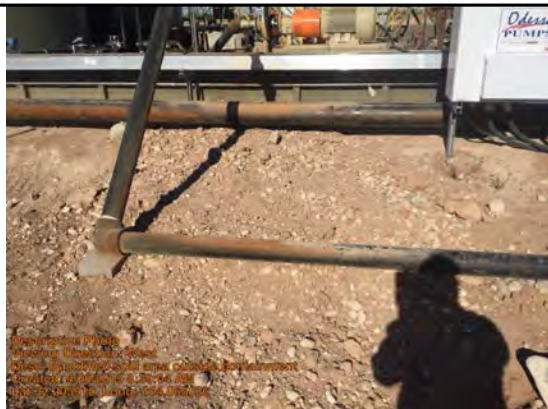
Backfilled spill area outside containment
