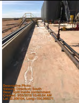
Spill inside containment on east side near separators
