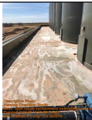
Spill inside containment extending south towards south end of containment near tanks on east side
