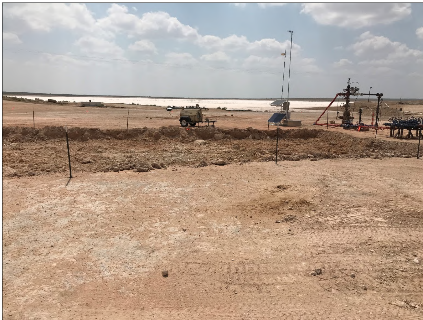
View facing west of the excavation and lake in the background.
