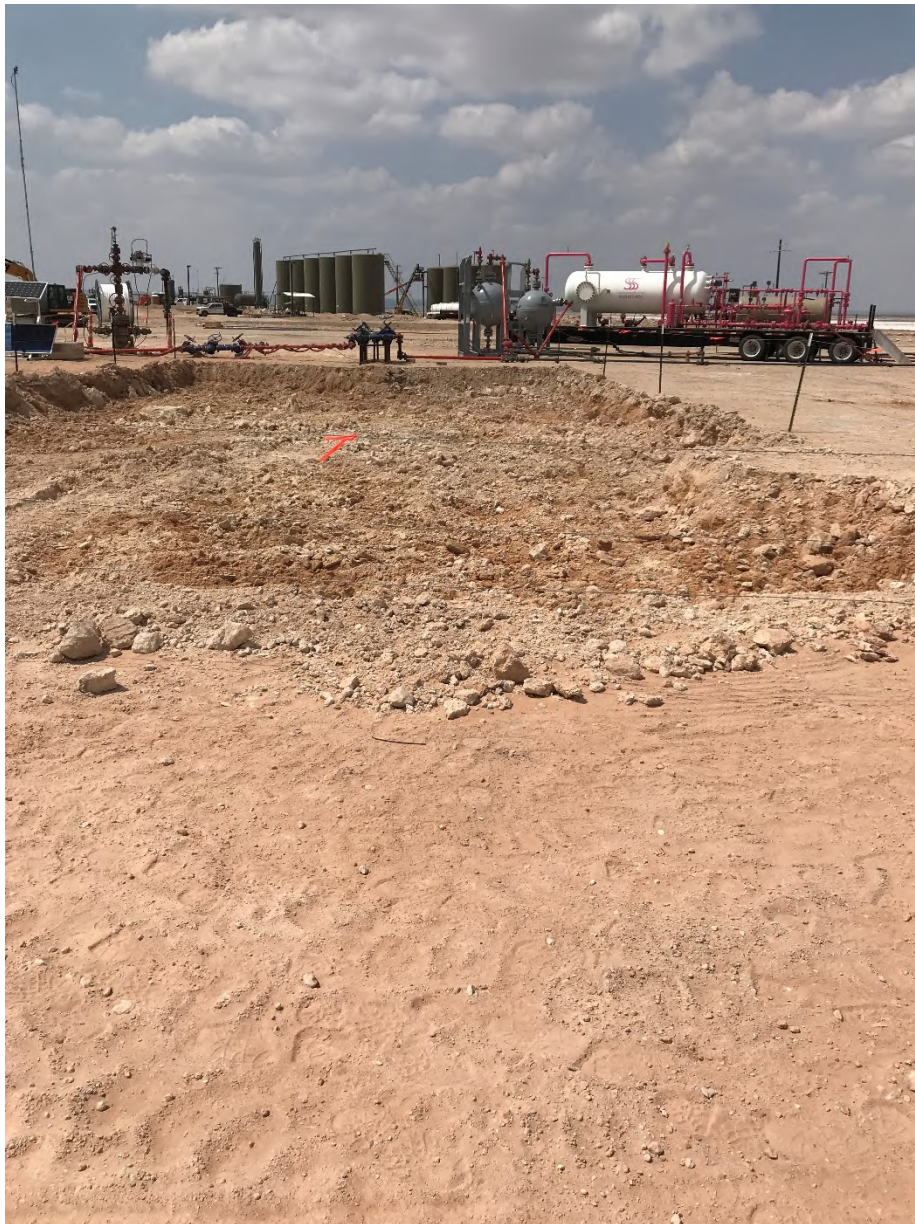
View facing north of the excavation.
