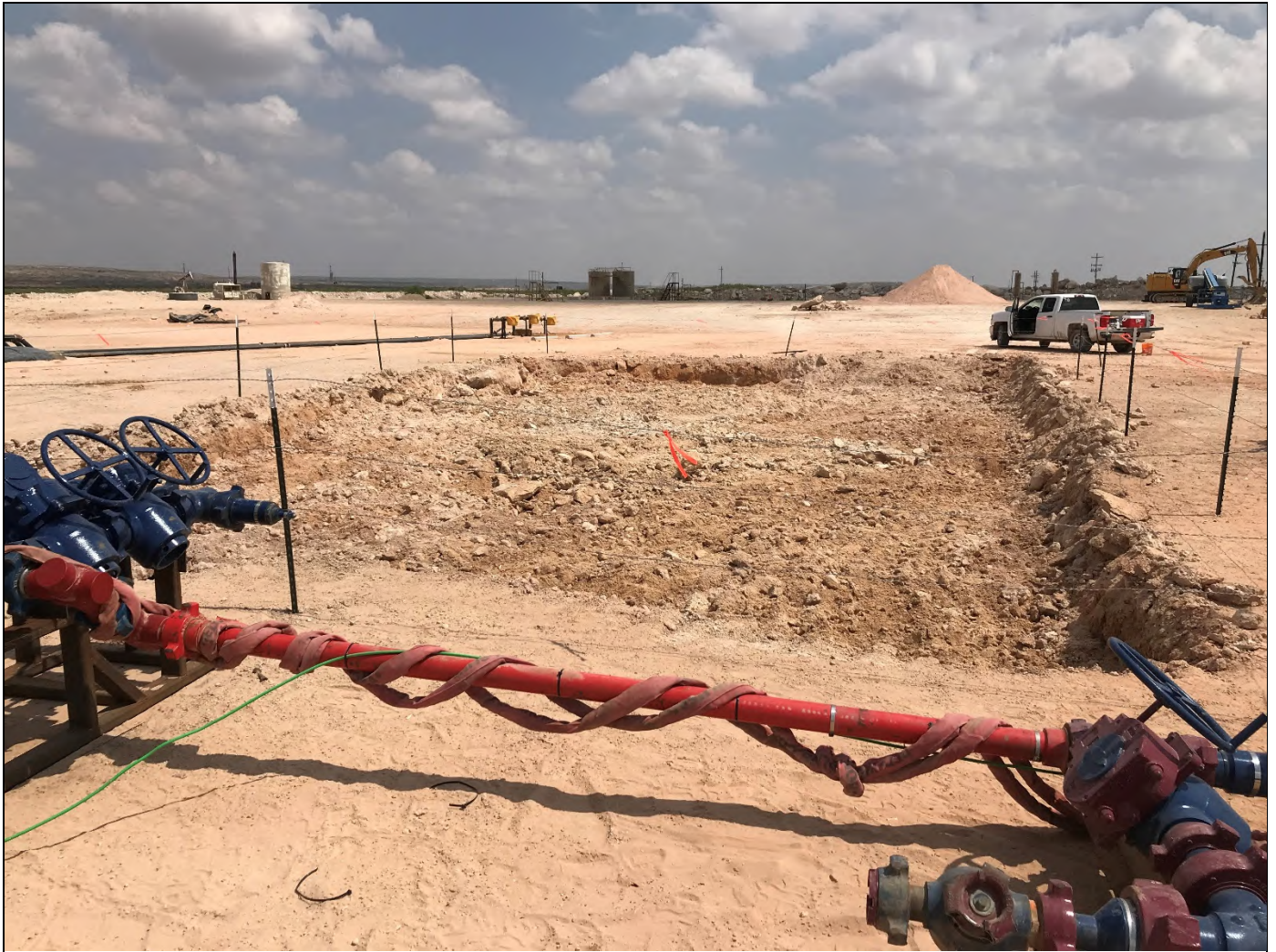
View facing south of the excavation.
