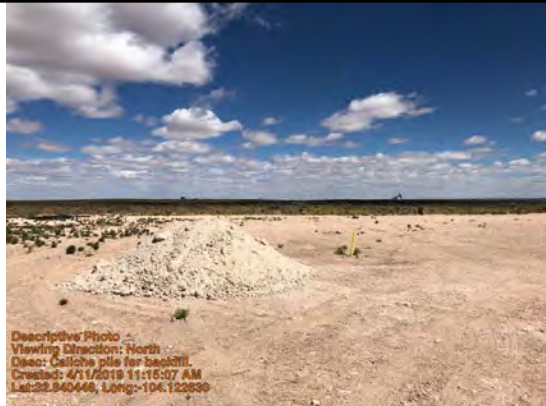
Caliche pile for backfill.
