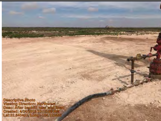
After backfill near well head
