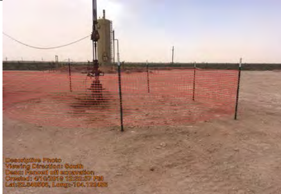
Fenced off excavation
