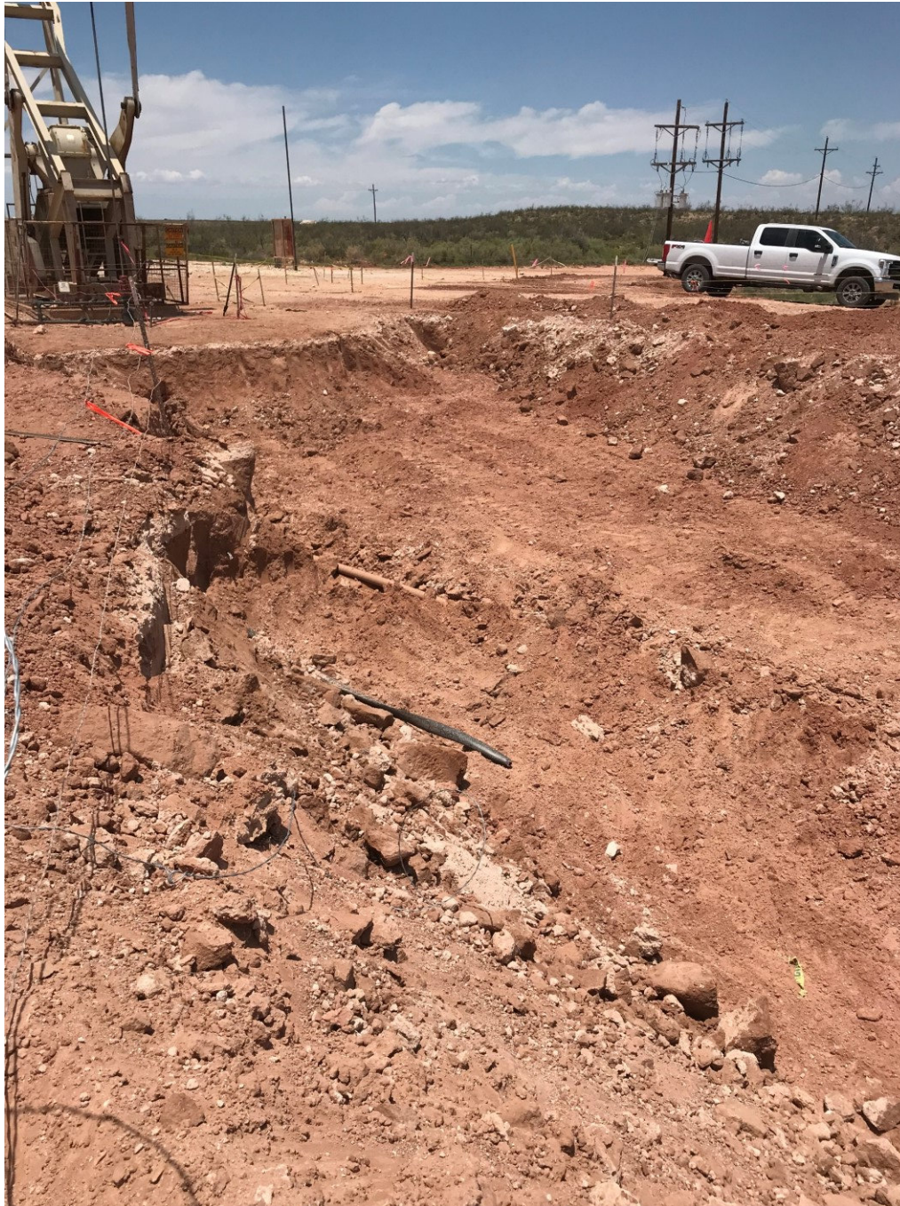
Western view of western portion of final excavation extent.
