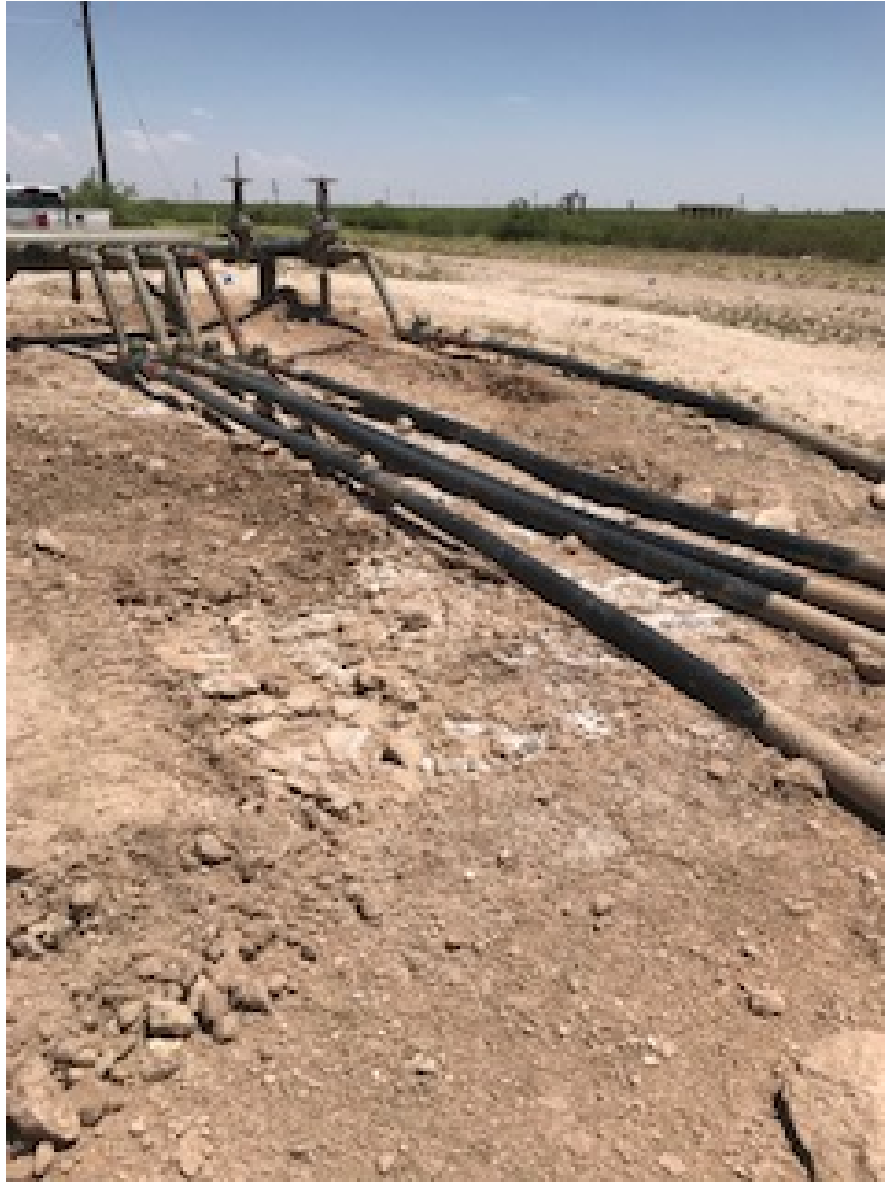
Excavation area – view north
