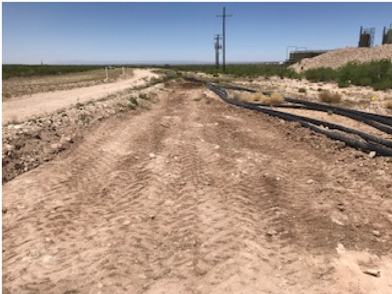
Excavation area – view south
