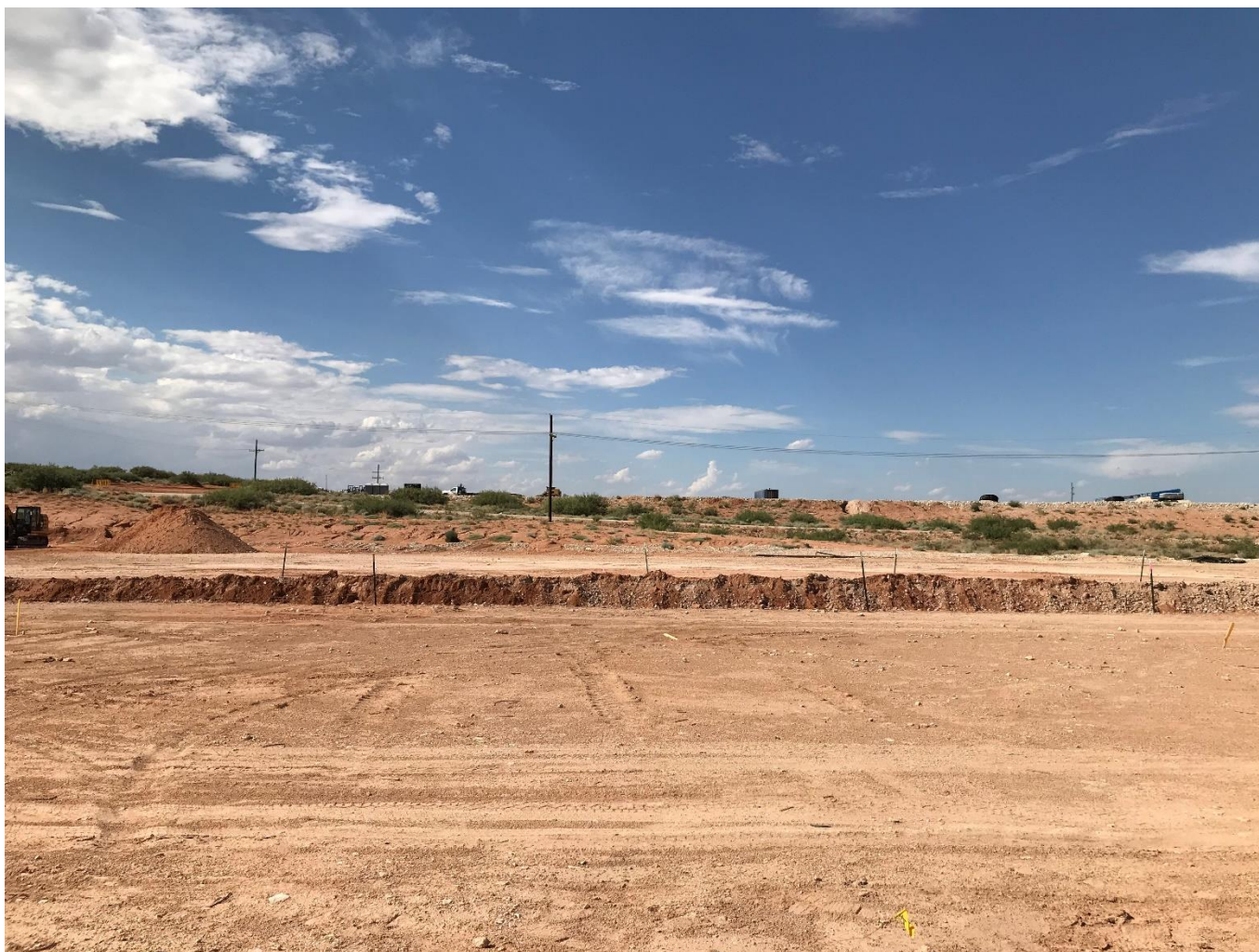
Northern view of final excavation extent.
